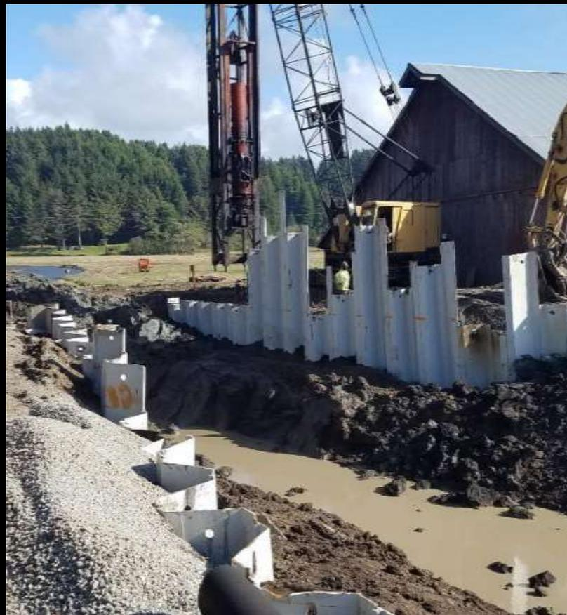
**Sheet Pile Installation Near Narrowed Channel and Barn Crossing**
