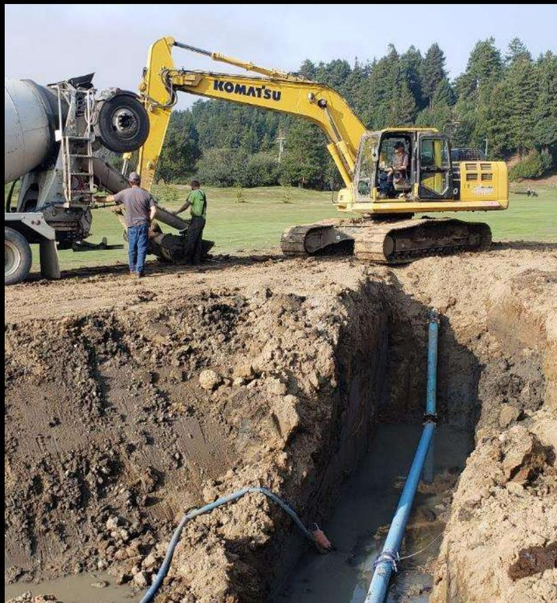
**Irrigation Water Line Replacement Under Widened Channel**
