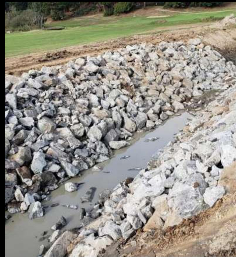
**Temporary Rock Grade Control Between Phases of Work**
