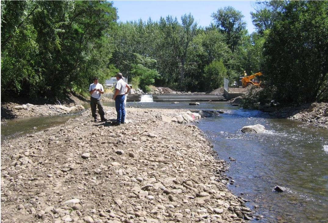
**Figure 44.** Looking upstream across the W-weir at Swackhammer just after its construction in July, 2005. Note the presence of the side channel located in the right arm of the W-weir. Native material was used to backfill the larger rocks of the arms.
