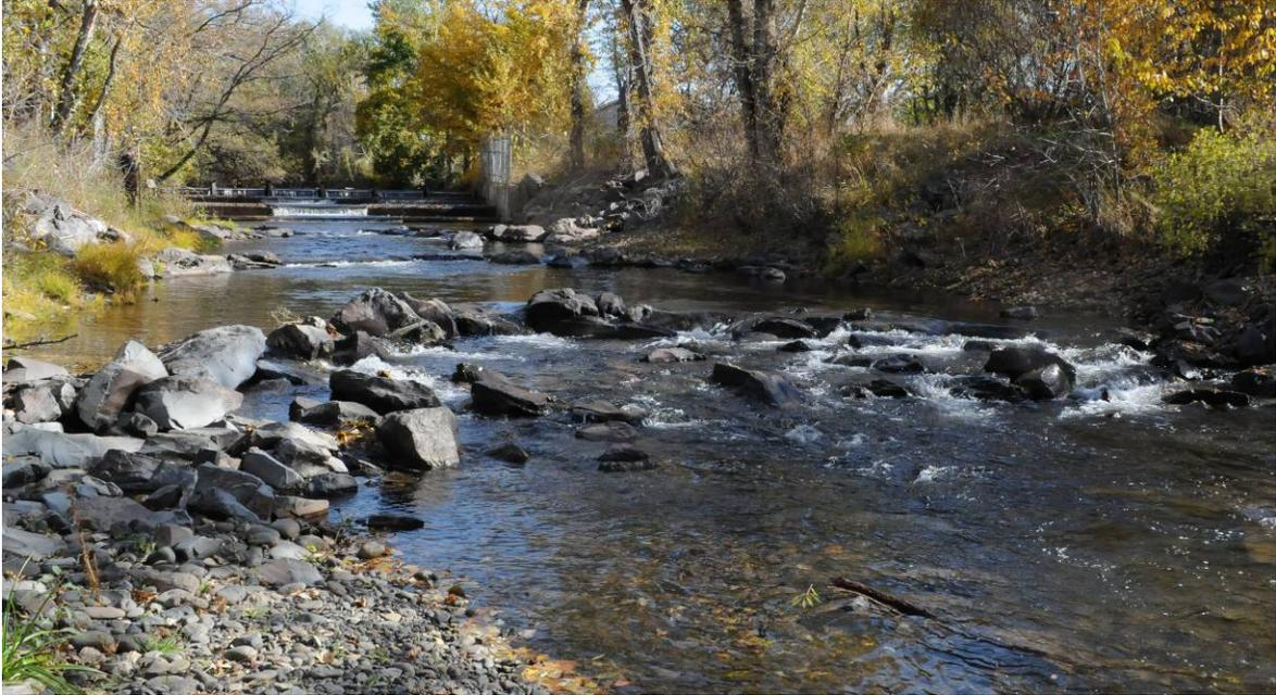
**Figure 61. Series of three U-weirs along Catherine Creek, just downstream from the Hempe-Hutchinson Diversion weir and fish passage structure. October 2008.**
