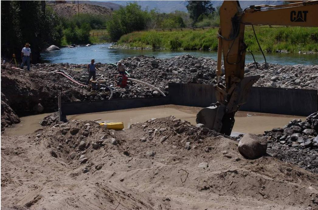
**Figure 18. Metal plate installed along the structure cross bar and left arm at East Fork Salmon EF 10-11.**
