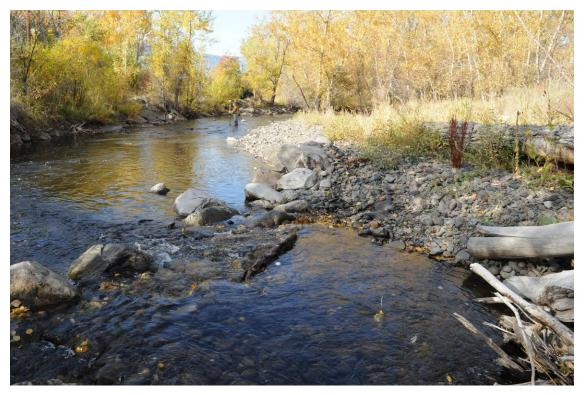
Figure 46. Right arm of left U-weir at Swackhammer. The center section and right arm of the structure are completely buried. October 2008.
