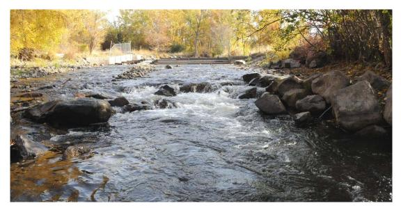
Figure 51. Photo looking upstream across left U-weir at Swackhammer. Several dislodged rocks have fallen into the scour pool. October 2008.
