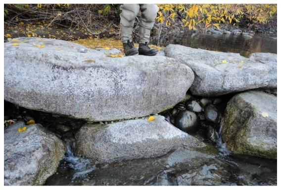
Figure 84. Spacing between header and footer rocks has filled in with sediment at Entiat River structure at RM 4.6.
