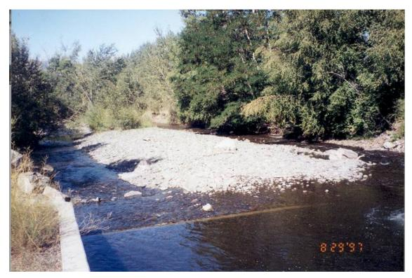
Figure 42. Prior to installation of the W-weir at Swackhammer, the area downstream from concrete weir was a depositional zone. This picture illustrates the conditions on August 29th, 1997 looking downstream.
