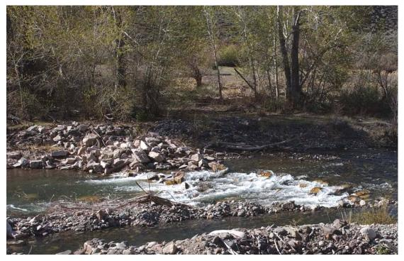
Figure 5. East Fork Salmon EF 7-8 on April 2004. Note smaller material along the left arm of structure.
