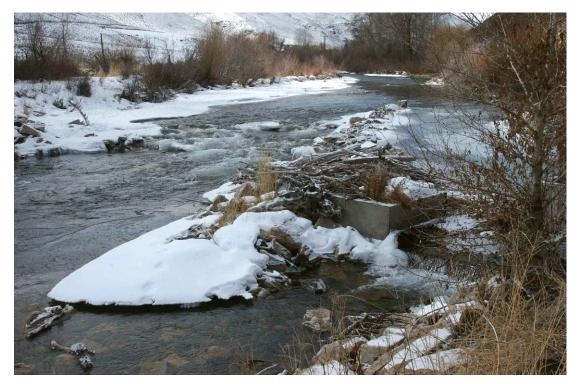
Figure 10. Looking upstream at the East Fork Salmon EF 7-8 structure in February 2006. Notice the berm extending upstream of the structure to guide flow toward the diversion gate.
