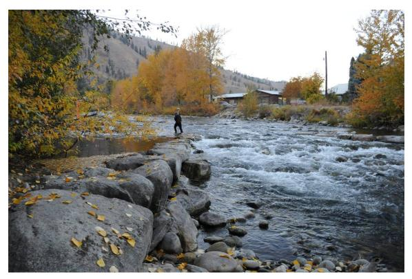
Figure 83. Header rocks along right arm of Entiat River structure at RM 4.6.
