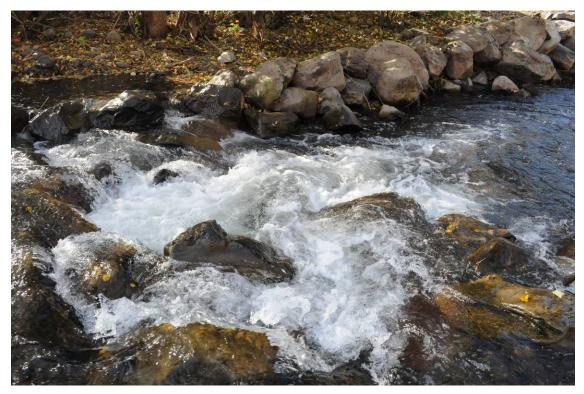
Figure 49. Throat of structure at Swackhammer. Several rocks have slumped into downstream scour pool, creating a series of steps, rather than a steep drop. October 2008.
