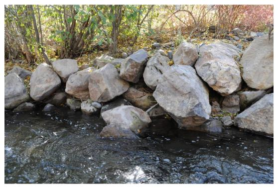
Figure 47. Left arm of left U-weir at Swackhammer. Note the slumping of some of the material where the footers have been dislodged and scoured. Some of this material does not appear to be present following initial construction but may have just been covered with backfilled material. October 2008.
