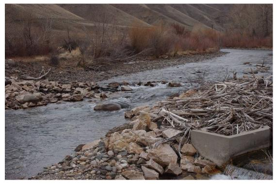
Figure 9. Looking upstream at the East Fork Salmon EF 7-8 structure in March 2003. Loose woody debris has piled up along the diversion channel and structure.
