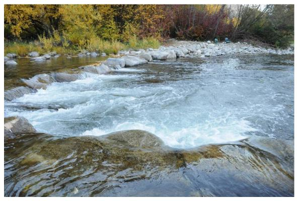
Figure 95. Throat of Entiat River structure at RM 5.1 which is acting hydraulically like a drop.
