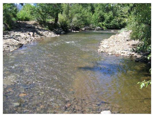
Figure 54. Photograph of the U-weir at Swackhammer just after construction in July 2005. The arms of the structure were backfilled and the throat set at grade.
