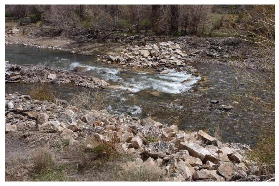
Figure 7. Looking down across the top of the East Fork Salmon EF 7-8 structure in May 2003. Note the lack of a berm extending upstream of the structure.
