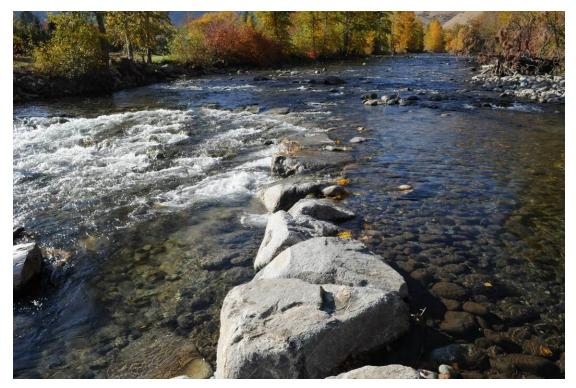
Figure 91. Throat of Entiat River structure at RM 3.4 is acting hydraulically similar to a ramp rather than a drop.
