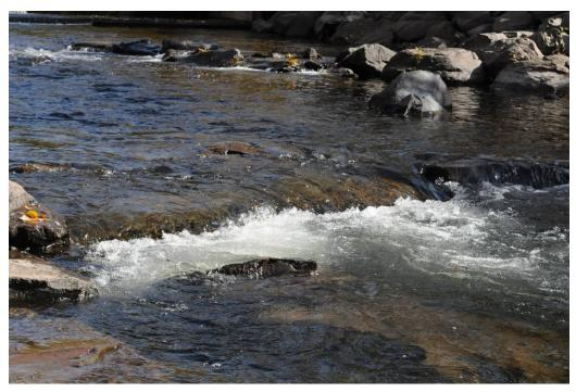
Figure 66. Remaining throat of HH2 at Hempe-Hutchinson. Note the titling of the footers and the headers that have slumped into the downstream scour pool.
