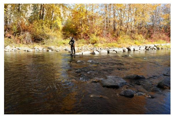
Figure 77. Throat of Entiat River structure at RM 3.2 where the majority of the header rocks have been dislodged.
