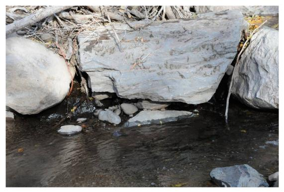
Figure 50. Rocks along right arm of left U at Swackhammer, illustrating minor seepage underneath and between the header rocks. October 2008.
