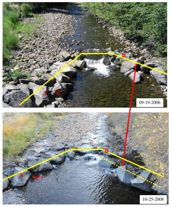
Figure 35. Bear Creek Site B U-Weir Looking Upstream showing rock movement along the left arm.
