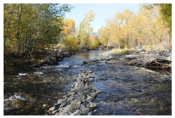
Figure 48. Looking downstream across W-weir at Swackhammer. Note the entire center and right arms have completely filled in with sediment and debris. October 2008.
