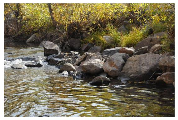
Figure 58.Connection of the throat and left arm of the structure at Swackhammer. Several rocks have fallen into the scour pool along the left arm of the structure.
