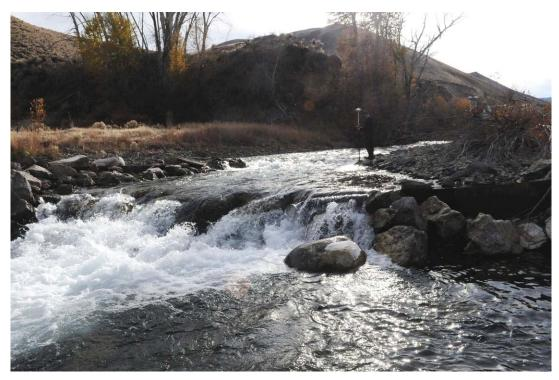
Figure 22. East Fork Salmon EF 10-11 in October 2008. Note significant change in drop height since construction, mobilization of larger boulders, and excessive deposition upstream of structure.
