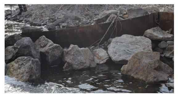
Figure 23. Exposed metal support along East Fork Salmon EF 10-11 structure cross bar (October 2008).
