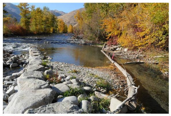
Figure 92. Gravel deposition upstream of the left arm of the Entiat River structure at RM 3.4
