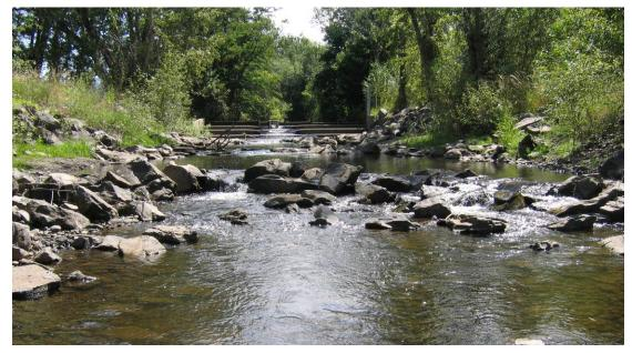
Figure 63. HH1 at Hempe Hutchinson in July 2005. Substantial shifting of the structure material occurred since the date of construction.
