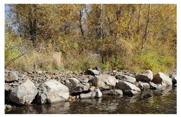
Figure 56. Right arm of U-weir at Swackhammer. Some voids present between larger rocks and a lot of the native backfilled material has been scoured out of structure. October 2008.
