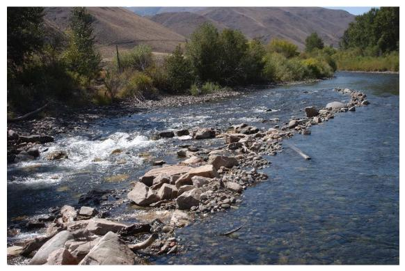
Figure 11. Looking upstream at the East Fork Salmon EF 7-8 structure in September 2007. The berm has been extended well beyond the head of the structure. Also, note seepage through the left arm of the structure.
