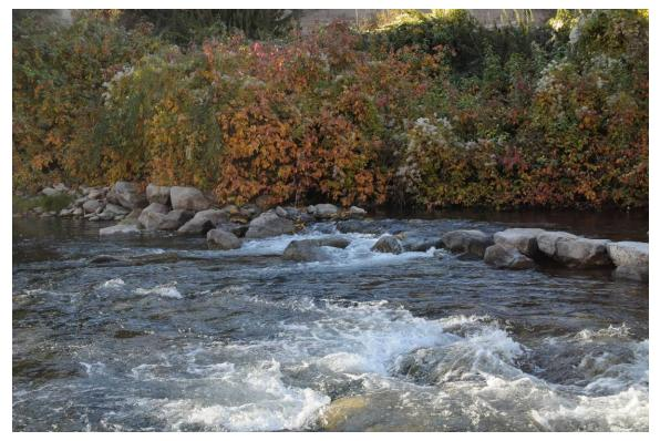
Figure 75. Looking at right arm of Entiat River structure at RM 3.1 with several dislodged header rocks.
