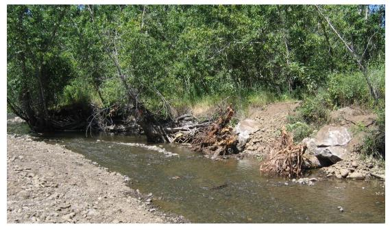
Figure 52. Rootwads installed along right bank between W- and U-weirs at Swackhammer. Photo looking downstream just after construction (July 2005).
