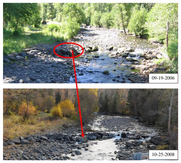
Figure 36. Bear Creek Site D1 U-Weir Looking Upstream displaying rock movement along both arms.
