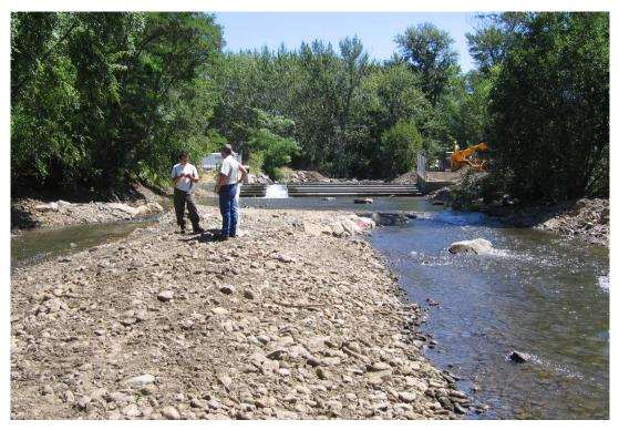
Figure 44. Looking upstream across the W-weir at Swackhammer just after its construction in July, 2005. Note the presence of the side channel located in the right arm of the W-weir. Native material was used to backfill the larger rocks of the arms.
