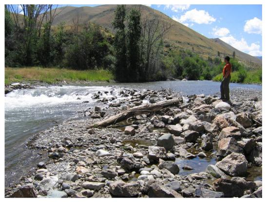
Figure 21. East Fork Salmon EF 10-11 in July 2005. Note depositional zone upstream from structure on right side of the photo (left bank)
