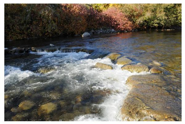
Figure 74. Throat of Entiat River structure at RM 3.1 showing movement of several header rocks.
