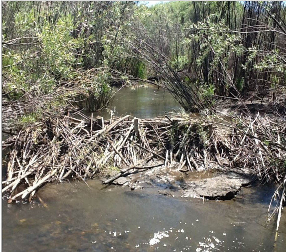
Figure 3-4. Photo of a beaver dam analog with post line and willow weave (photo from Dr. Michael Pollock).
