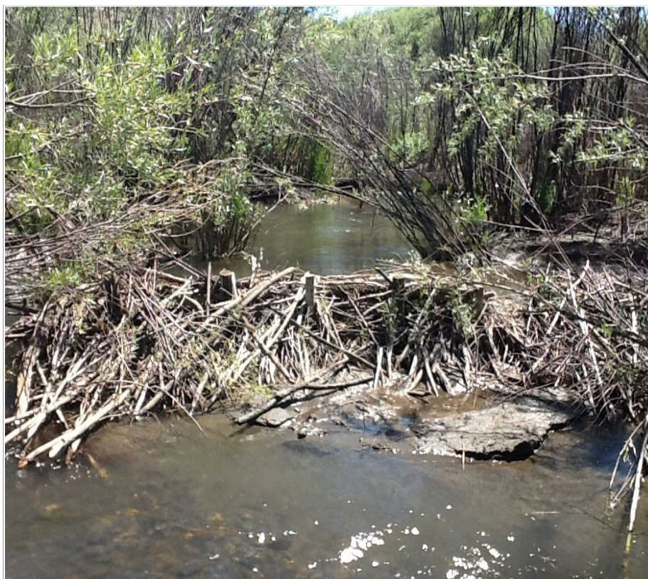
Figure 3-4. Photo of a beaver dam analog with post line and willow weave (photo from Dr. Michael Pollock).
