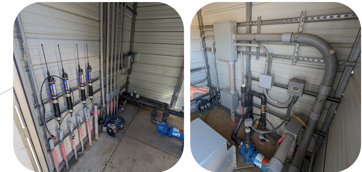
Powerhouse for flow regulation
