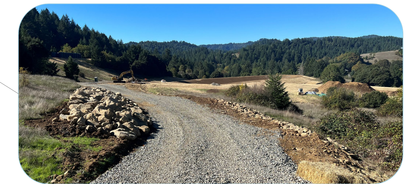
Upgraded access road and culverts
