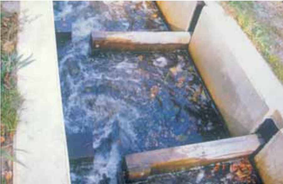
Figure 5.20: Slot current in a slot pass
