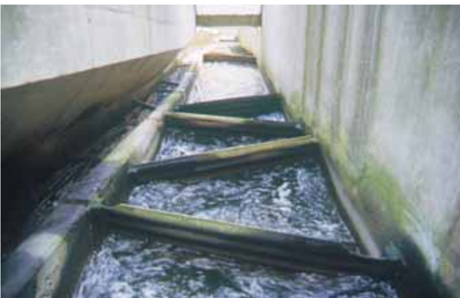
Figure 5.40: Rhomboid pass and eel ladder on the Sauer dam at Rosport (Rhineland-Palatinate).
