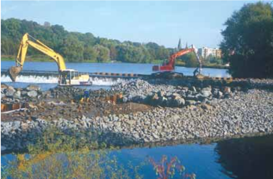
Figure 4.40: Spillenburg weir; fish ramp under construction
