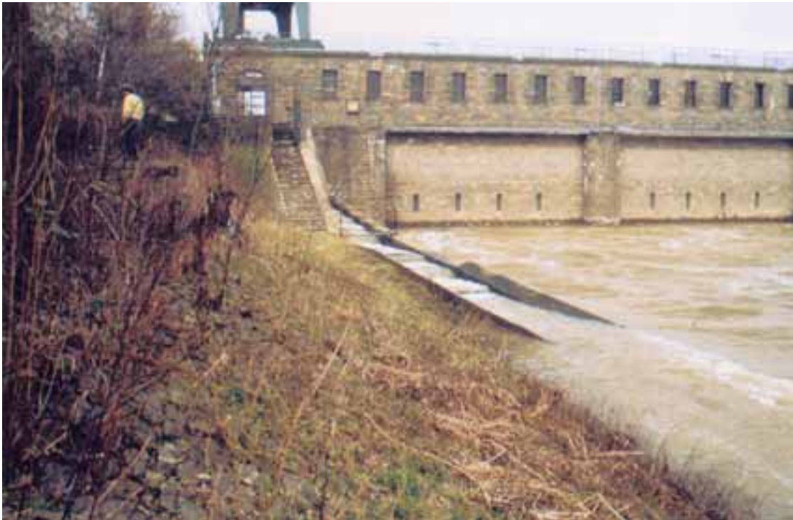
Figure 5.11: The Coblenz/Moselle fish pass (view from tailwater)
