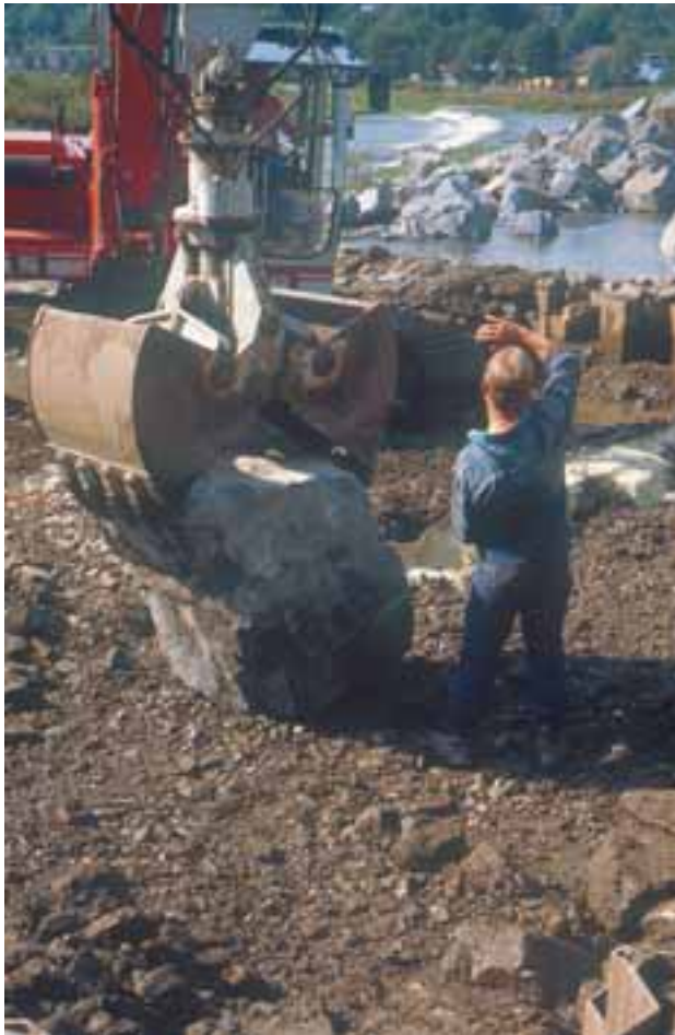
Figure 4.38: Setting the boulder bars
