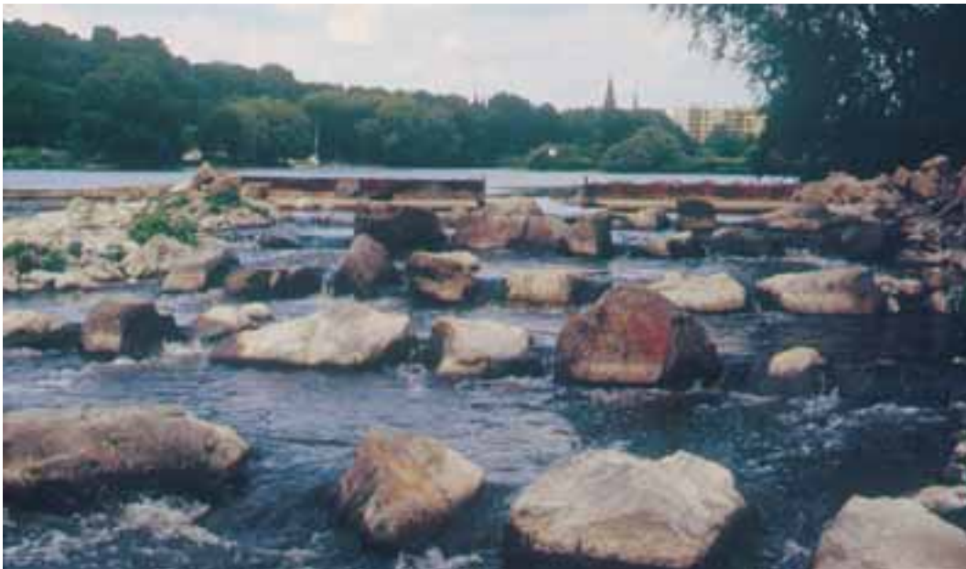
Figure 4.41: Spillenburg weir; fish ramp after completion
