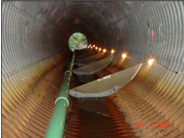
Figure 7-9. Baffles in circular pipe culverts are most commonly positioned in the “corner”, but can also be placed on the side. (Photos courtesy of Caltrans and ODOT)
