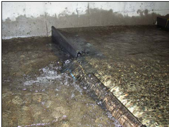
Figure 7-6. Baffle weirs spanning a steep-slope box culvert. (Photos courtesy of ODOT)
