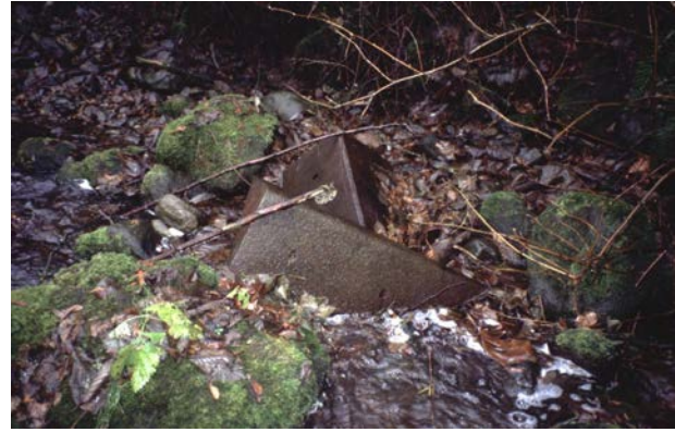
b) failure due to insufficient anchoring
