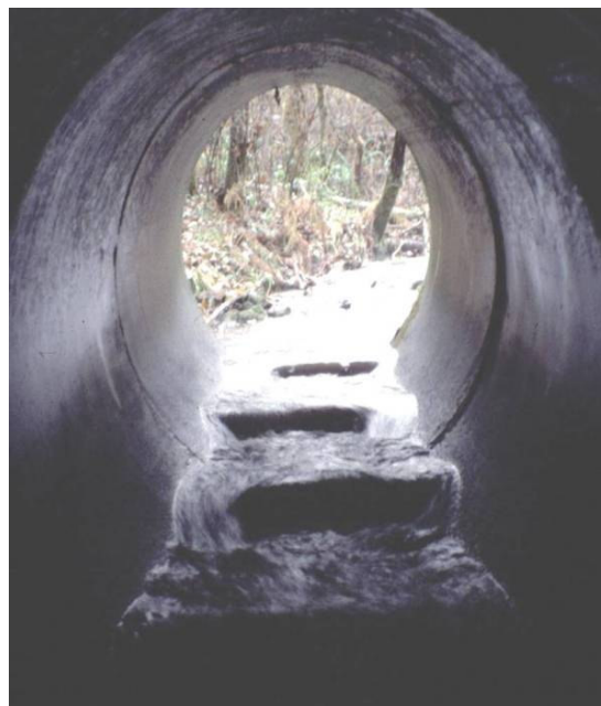
Figure 2-6. Baffles under low-flows
