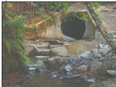
b) concrete weirs
