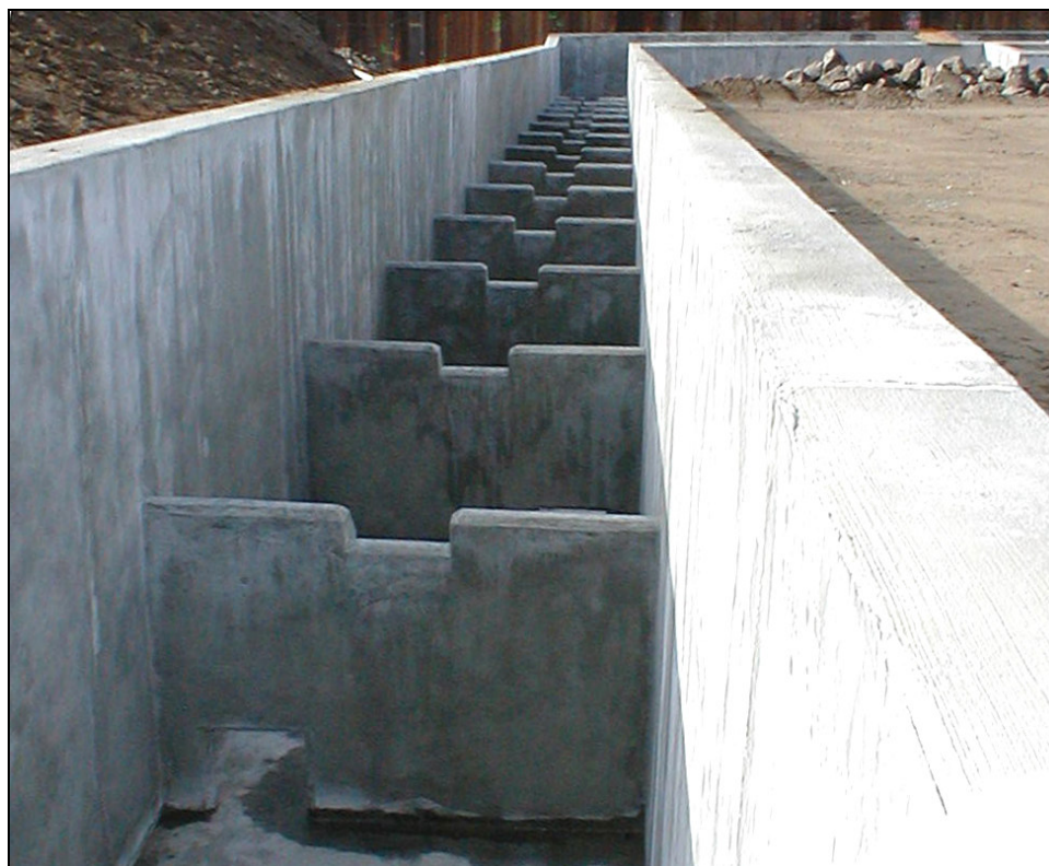
Figure 9.1. Pool and weir ladder.
