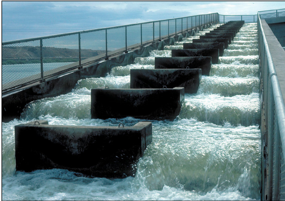
Figure 9.2. Ice Harbor fishway (courtesy of U.S. Army Corps of Engineers).
