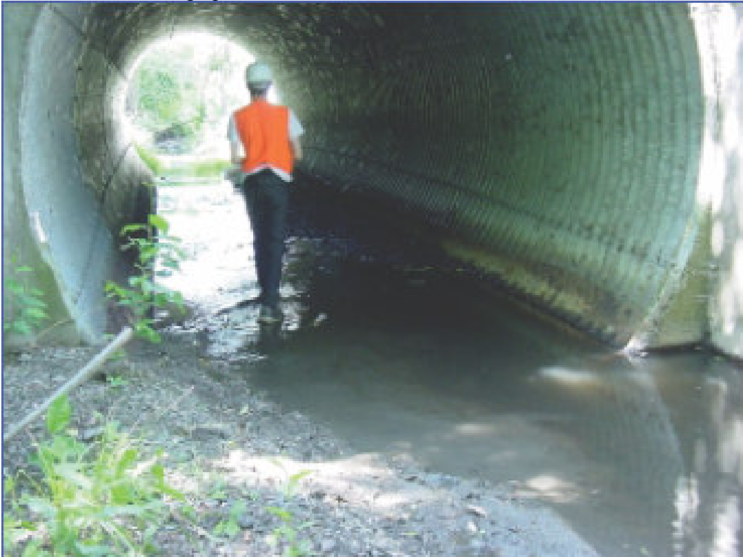
Culvert outlet looking upstream
