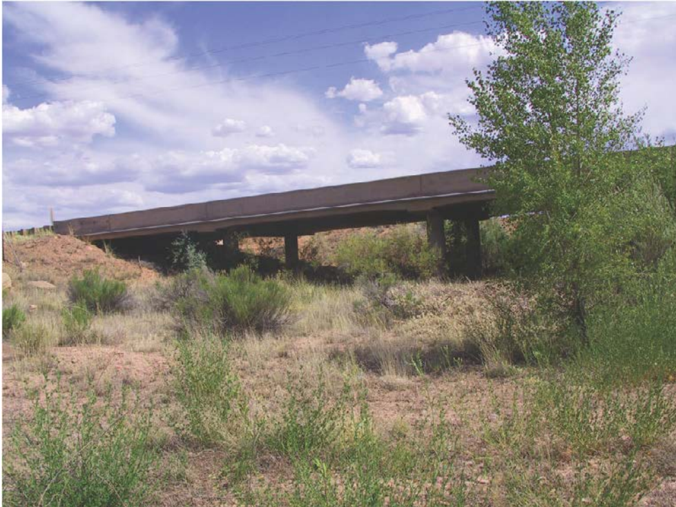
Stoney Creek Bridge
