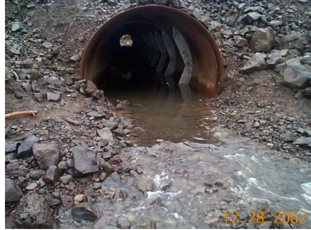
Figure 7-9. Baffles in circular pipe culverts are most commonly positioned in the “corner”, but can also be placed on the side. (Photos courtesy of Caltrans and ODOT)
