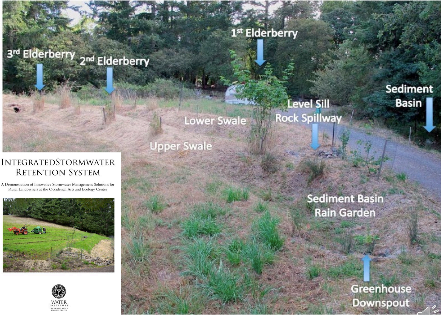
Figure 2. Image of the sediment basins and swales planted with California natives as of July 2012
