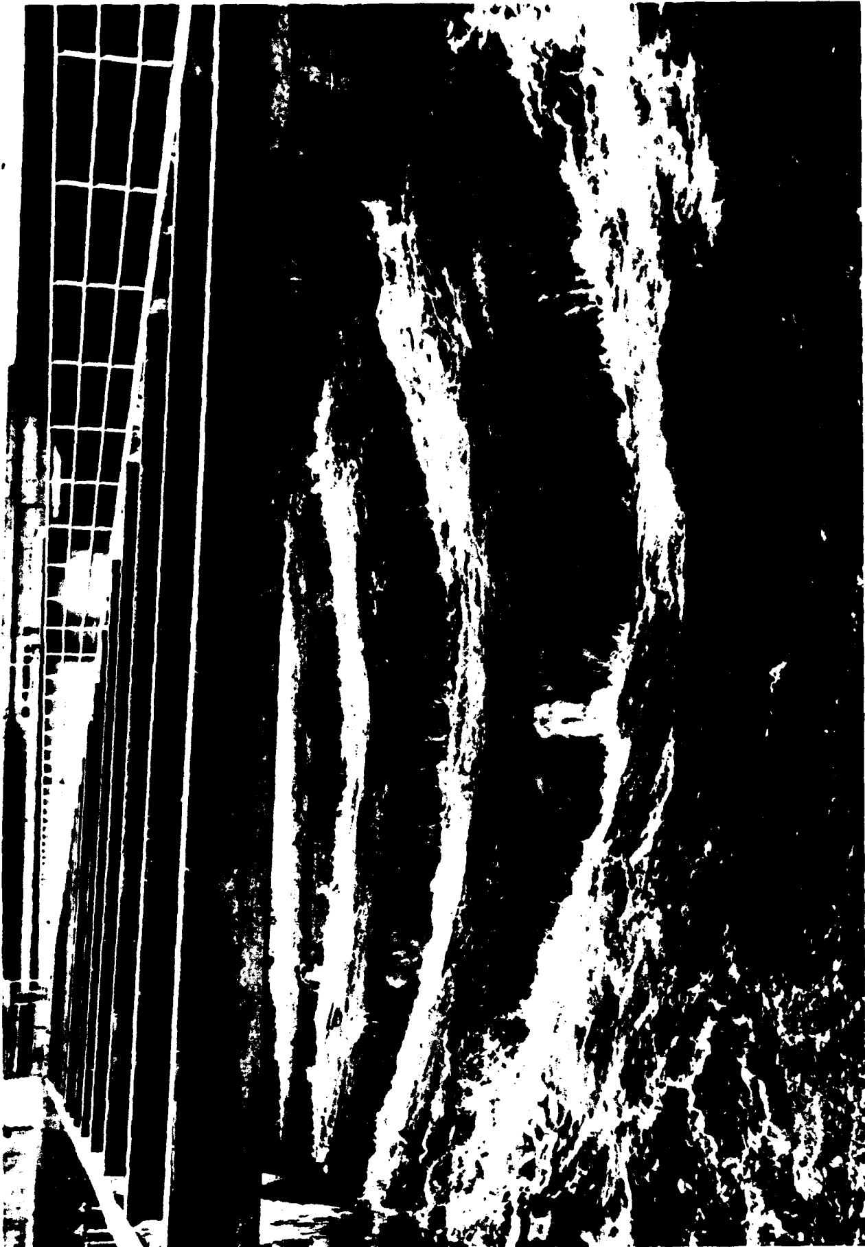
Z McNary Dam Fishways Showing Undesirable Surge Corps of Engineers, Walla District
