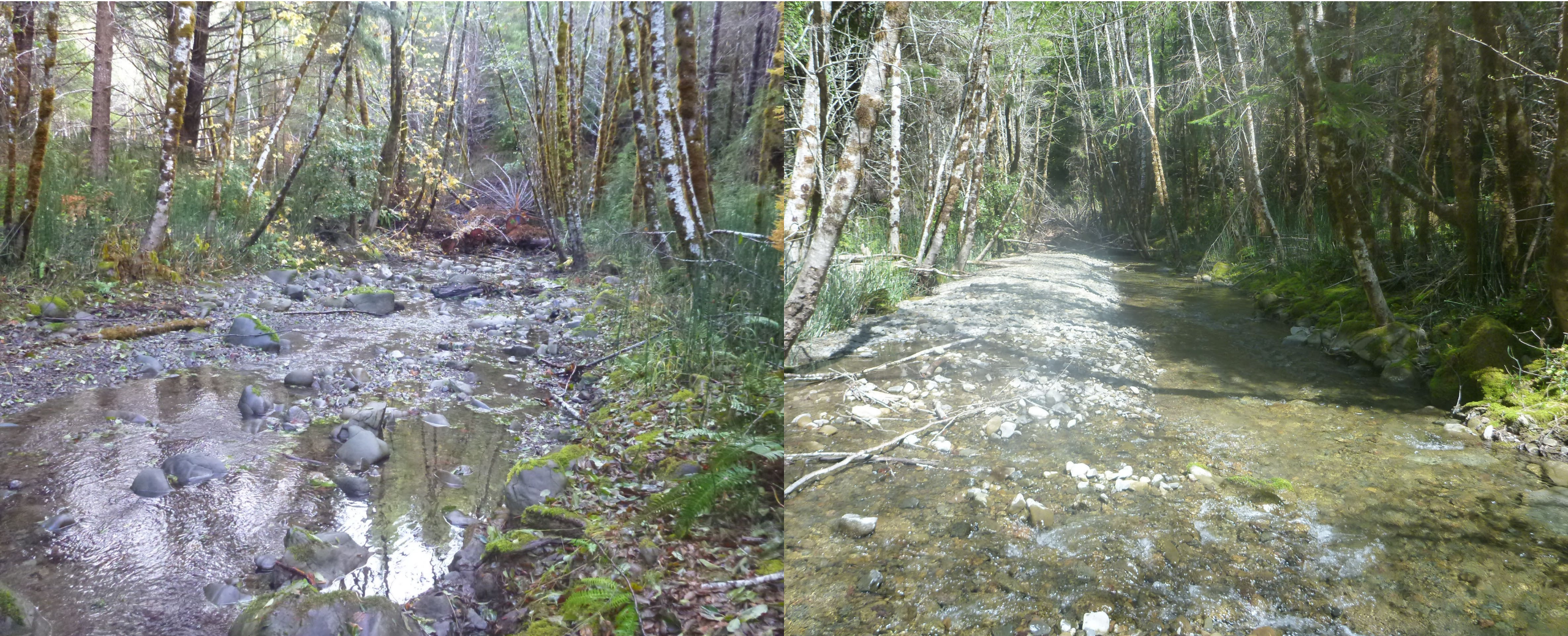
Sholes Creek Site. November 2020 post wood placement but prior to high flows (left), April 6 2021 (right), after desposition of spawning sized gravel
