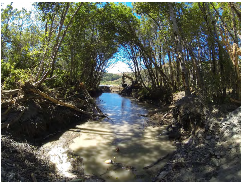
Slough excavation #1 in 2014
