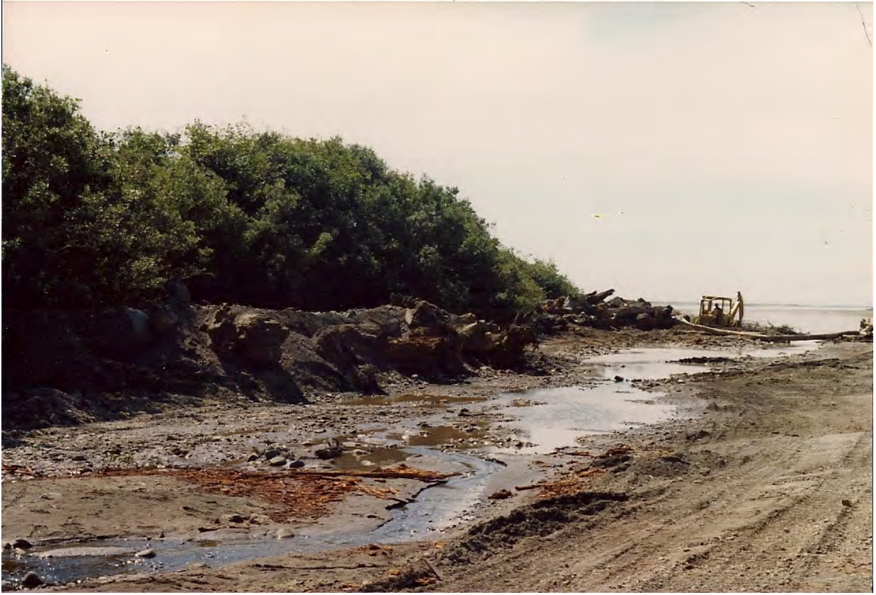
1991 Revetment structures south bank
