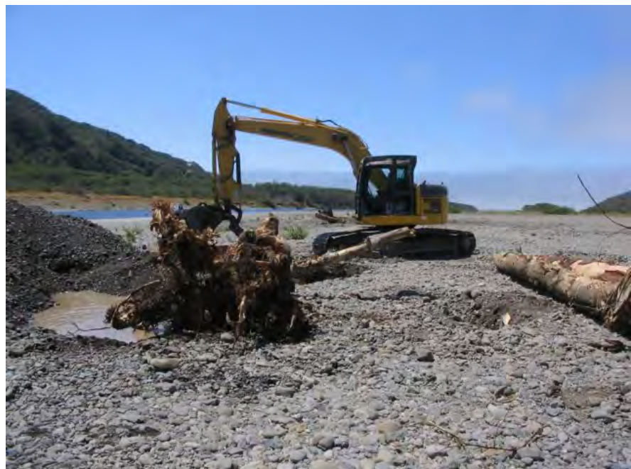
Apex jams in construction 2014
