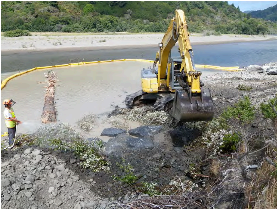
Construction in progress of the 7 th LWD structure, August 2011
