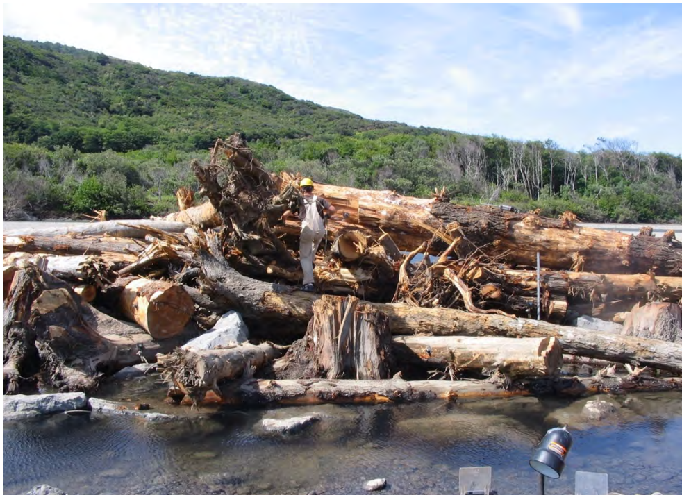
2007 structure as built
