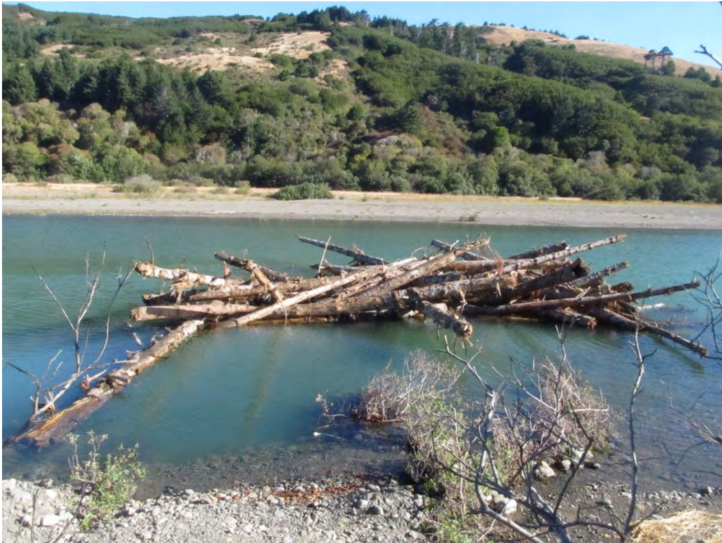
As built - 7 th LWD structure completed, August 2011
