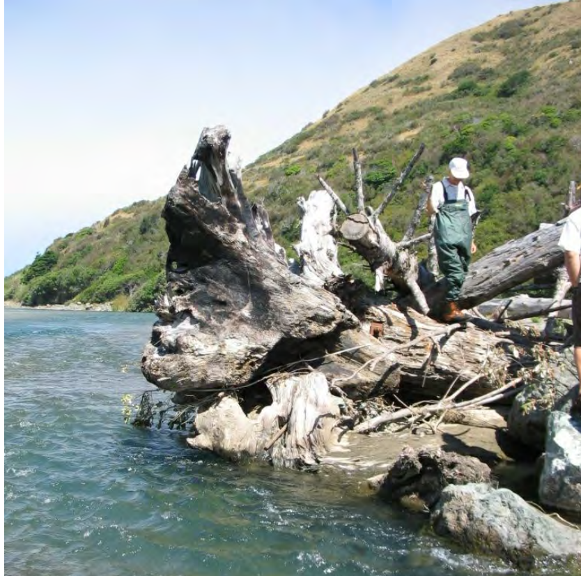
Gary Flossi (CDFW) on field tour of structure #3 built in 2003
