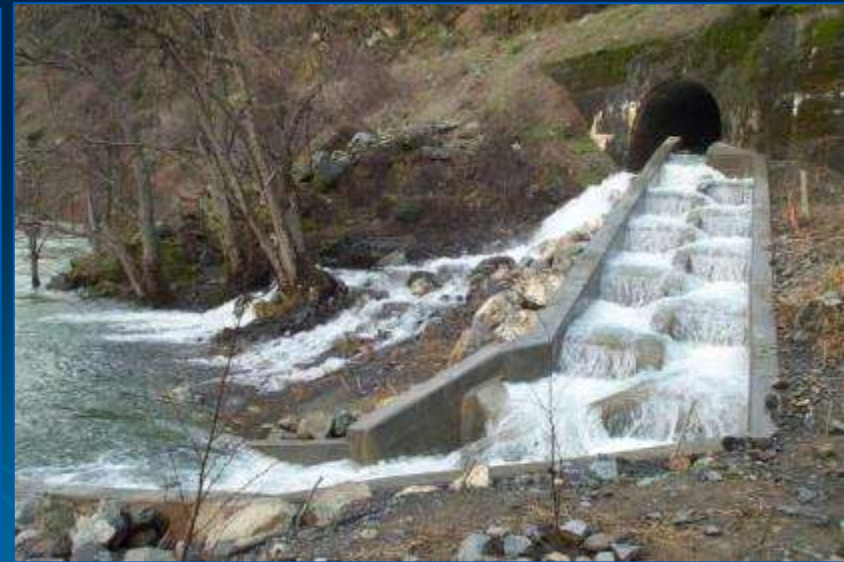
Bypass "Serpentine" Pool-and-Weir Fishway
