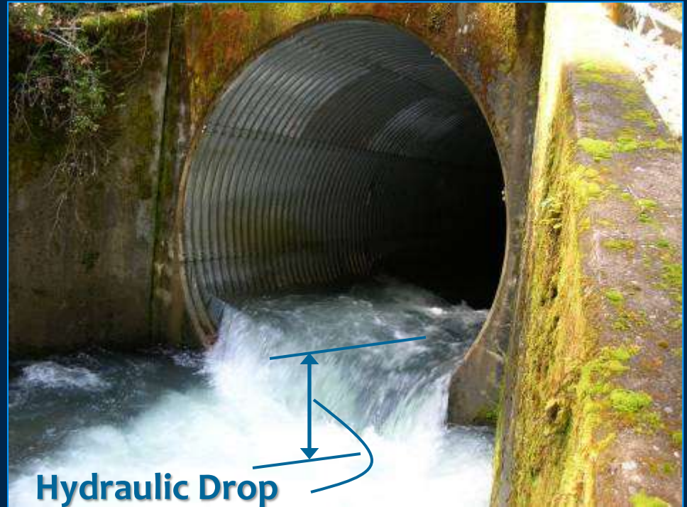
High Fish Passage Flow (excessive hydraulic drop)
