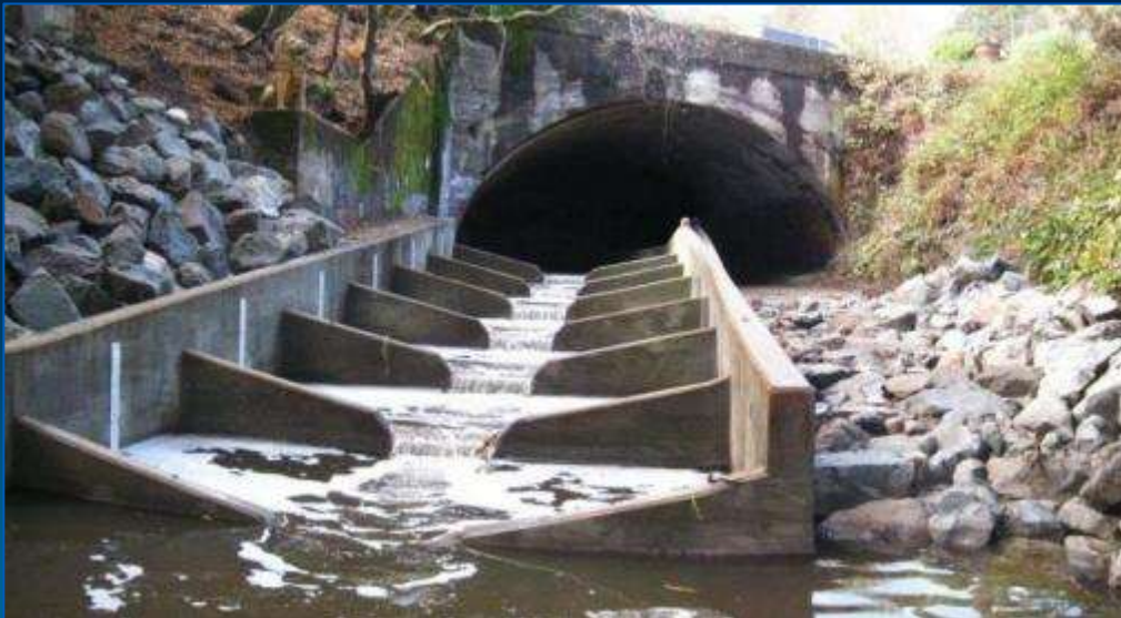
Partial Width Pool-and-Chute Fishway
