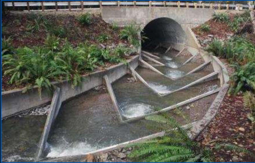
Full Width "Vortex" Pool-and-Chute Fishway
