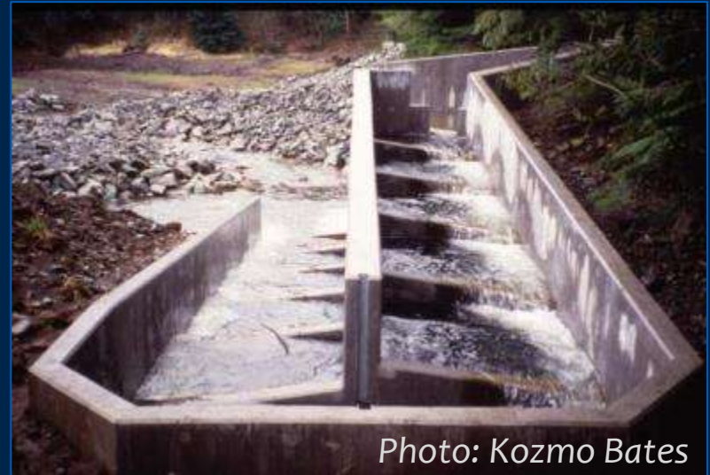
Bypass Pool-and-Weir Fishway
