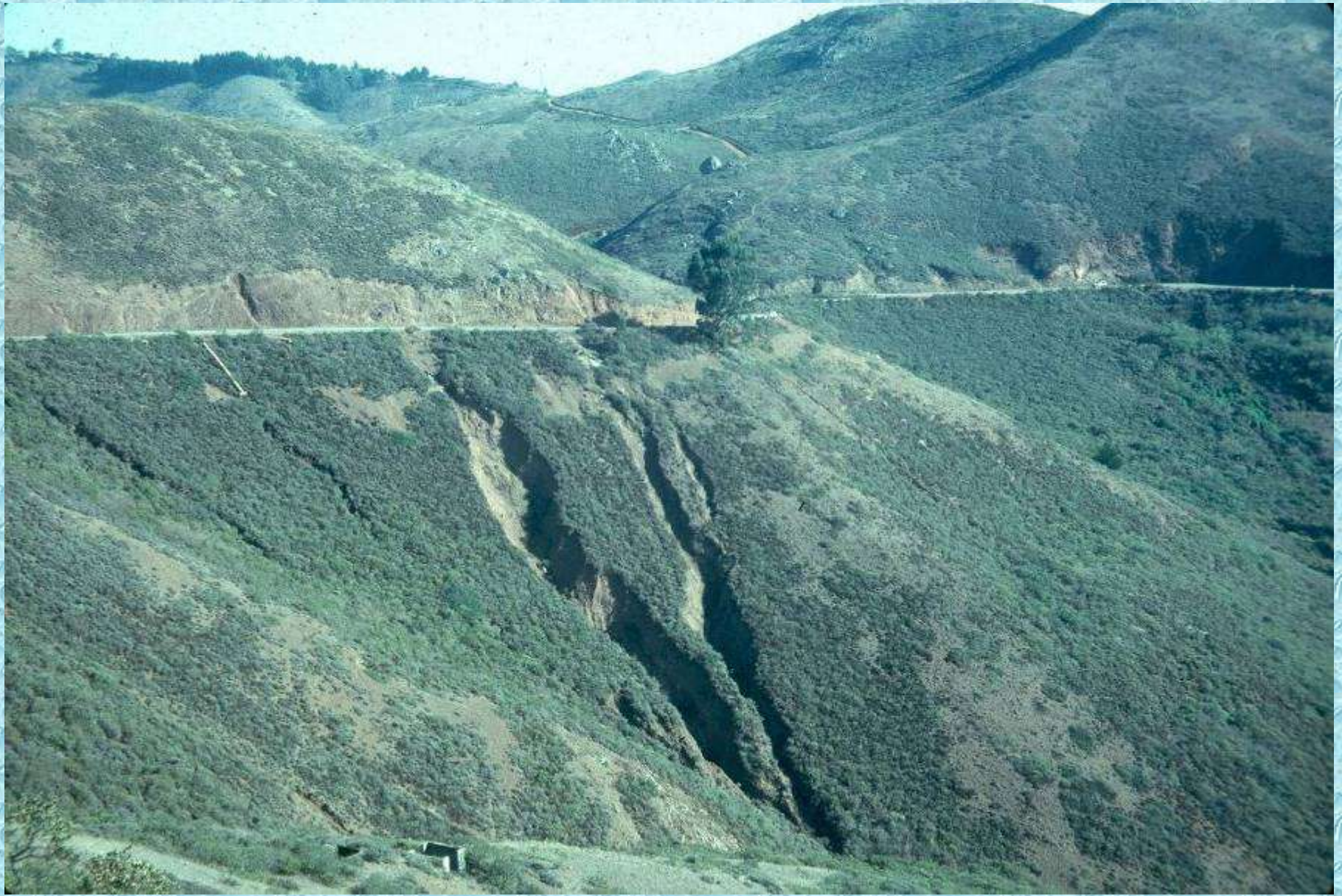
Gullies from road surface runoff
