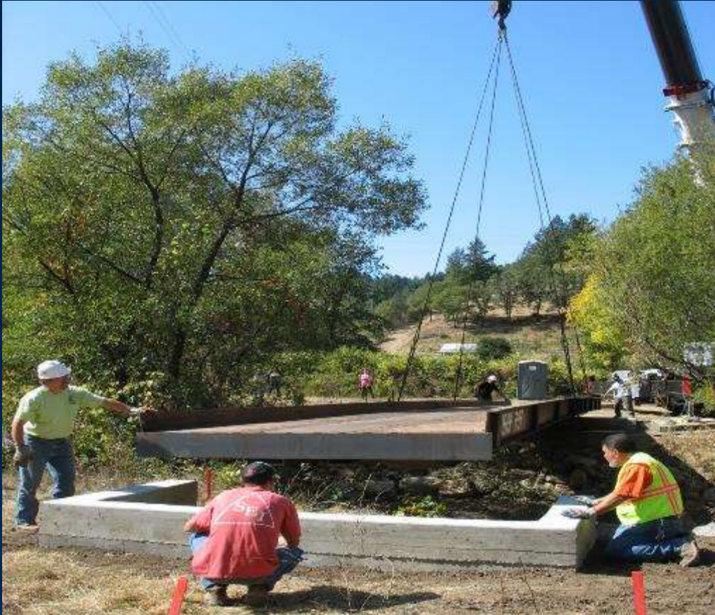
Bridge Installation, Navarro River
