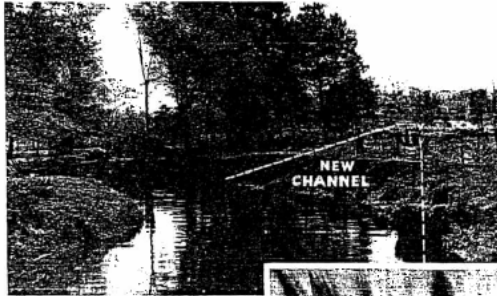
Straightening of Pequest River in New Jersey by CCC workers stopped its yearly floods. Location of new channel is seen at right. Note temporary dam at left to provide volume of water for scouring blasted channel.
