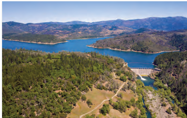
Scott Dam on the Eel River. Credit: Kyle Schwartz
