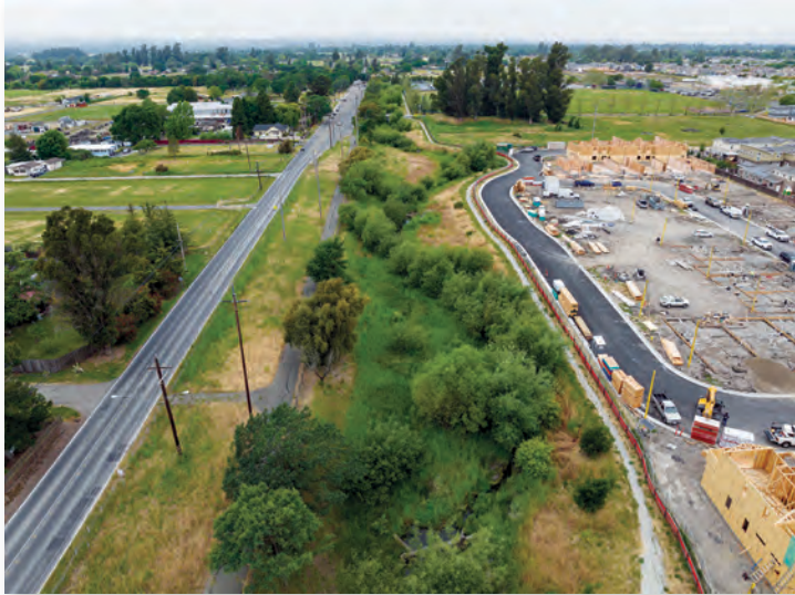
Lower Colgan Creek Restoration in southwest Santa Rosa. Credit: City of Santa Rosa
