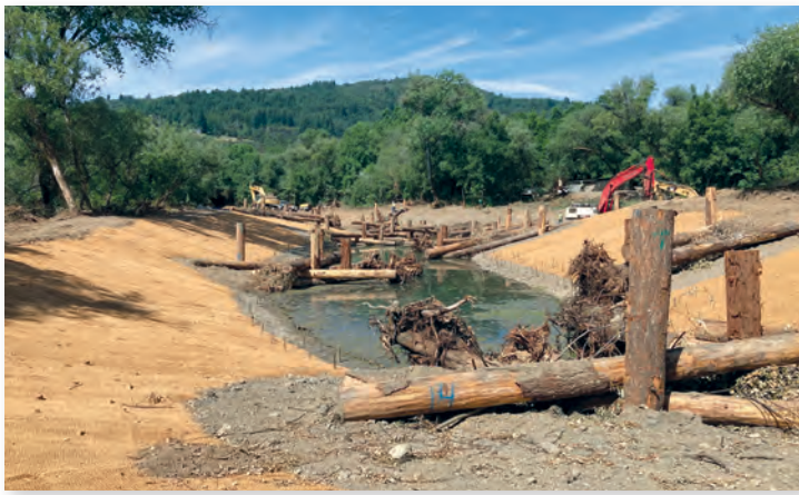
A Dry Creek habitat enhancement under construction on private property. This project was built by McCullough Construction. Implementation of the project was managed by the USACE. The photo of this newly constructed project was taken during the 2023 construction season. Credit: Justin Smith
