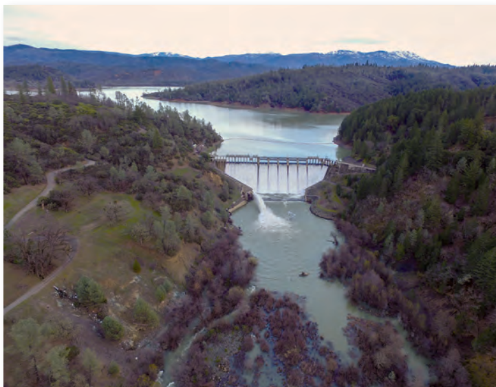
Scott Dam on the Eel River blocks 150 miles of salmon.
