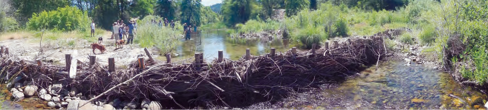
Beaver dam analogue constructed in 2014 by the Scott River Watershed Council on Sugar Creek in Scott Valley. By Eli Asarian
