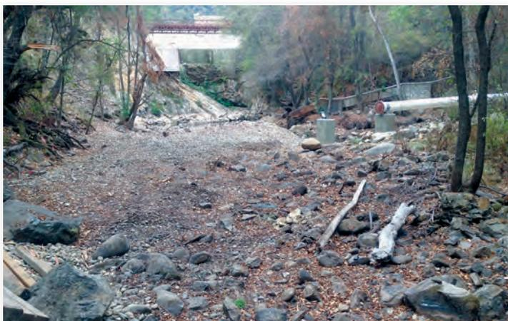
*Looking upstream to the end of the spillway of Los Padres Dam and seeing nearly complete downstream fish passage, start of ladder and trap, remains of gravel injection and extension of spillway. By Brian LeNeve*
