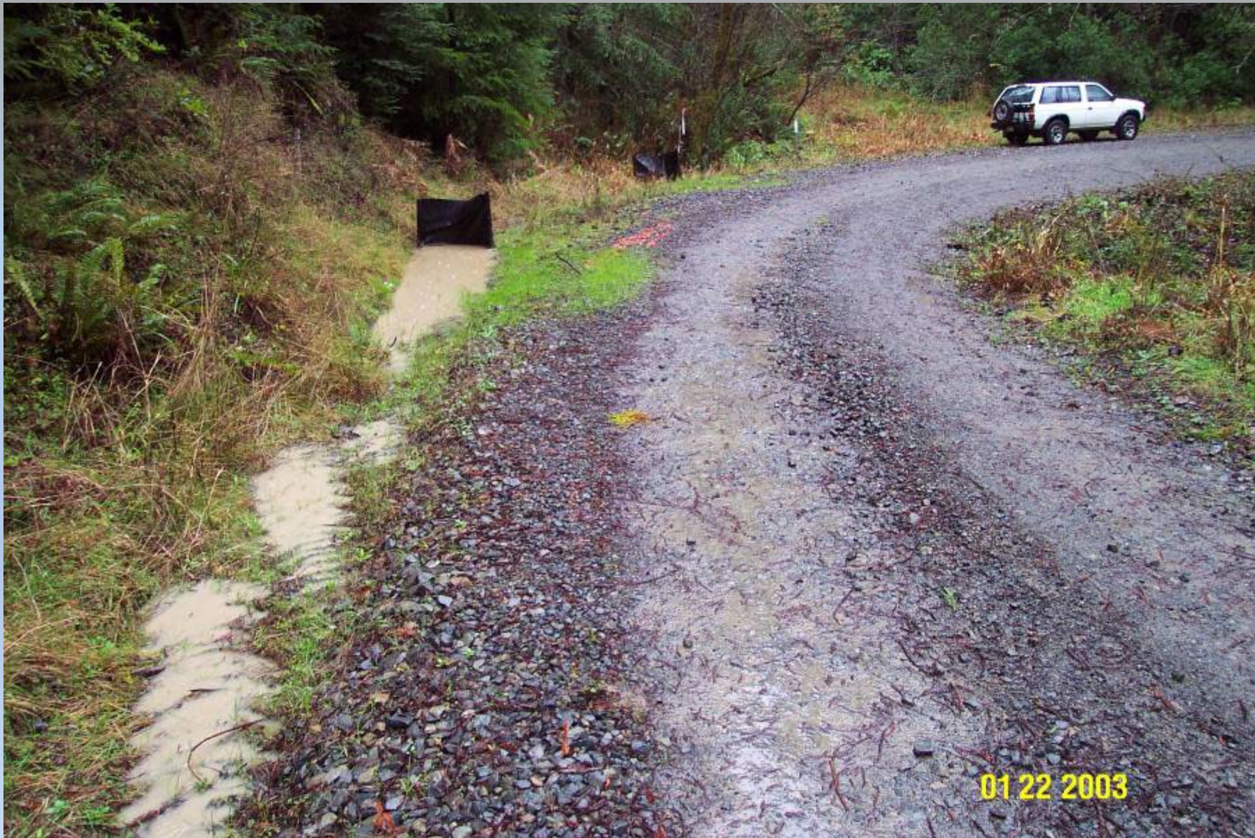
Silt fence ditch filter
