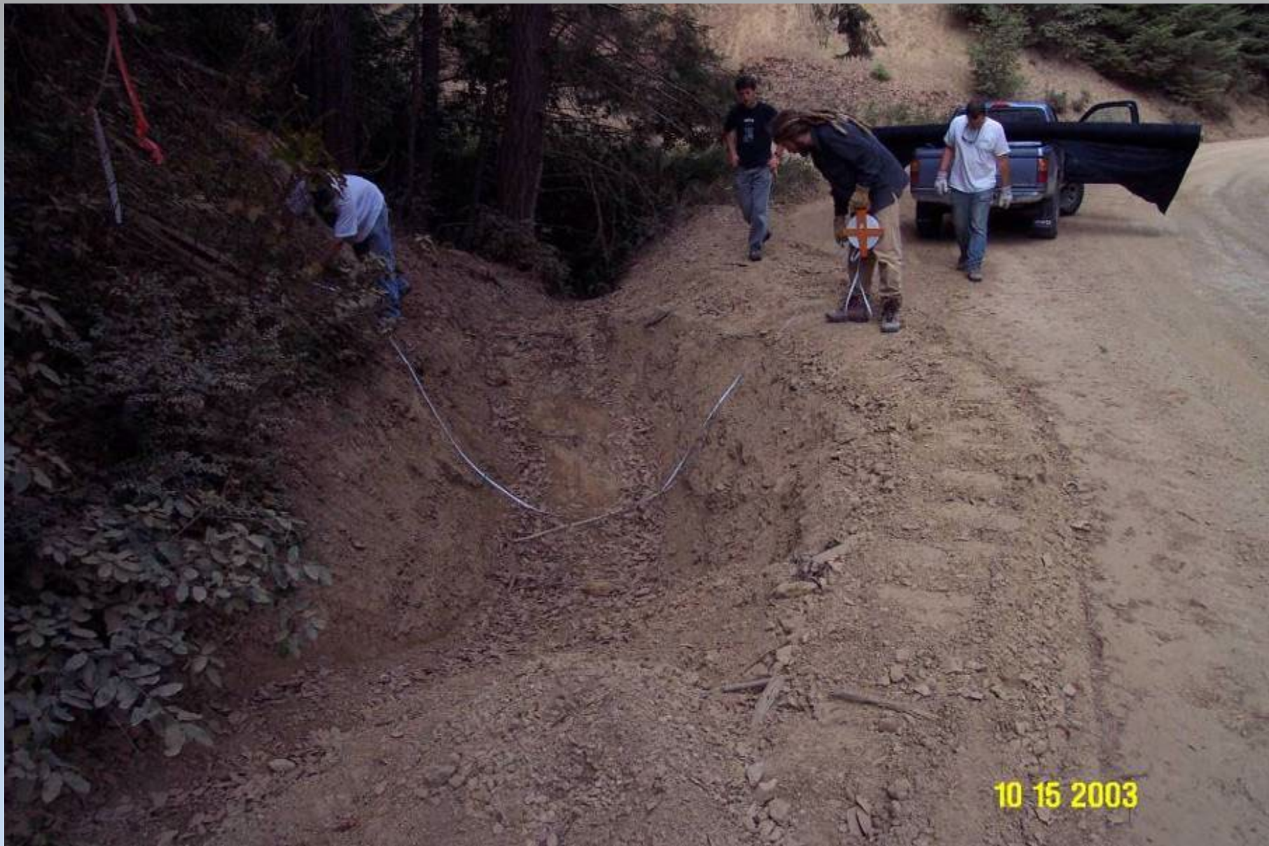
Sediment basin under construction
