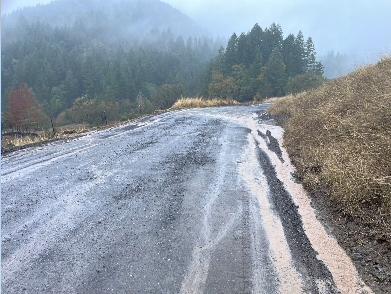
Dip does not have enough outslope
