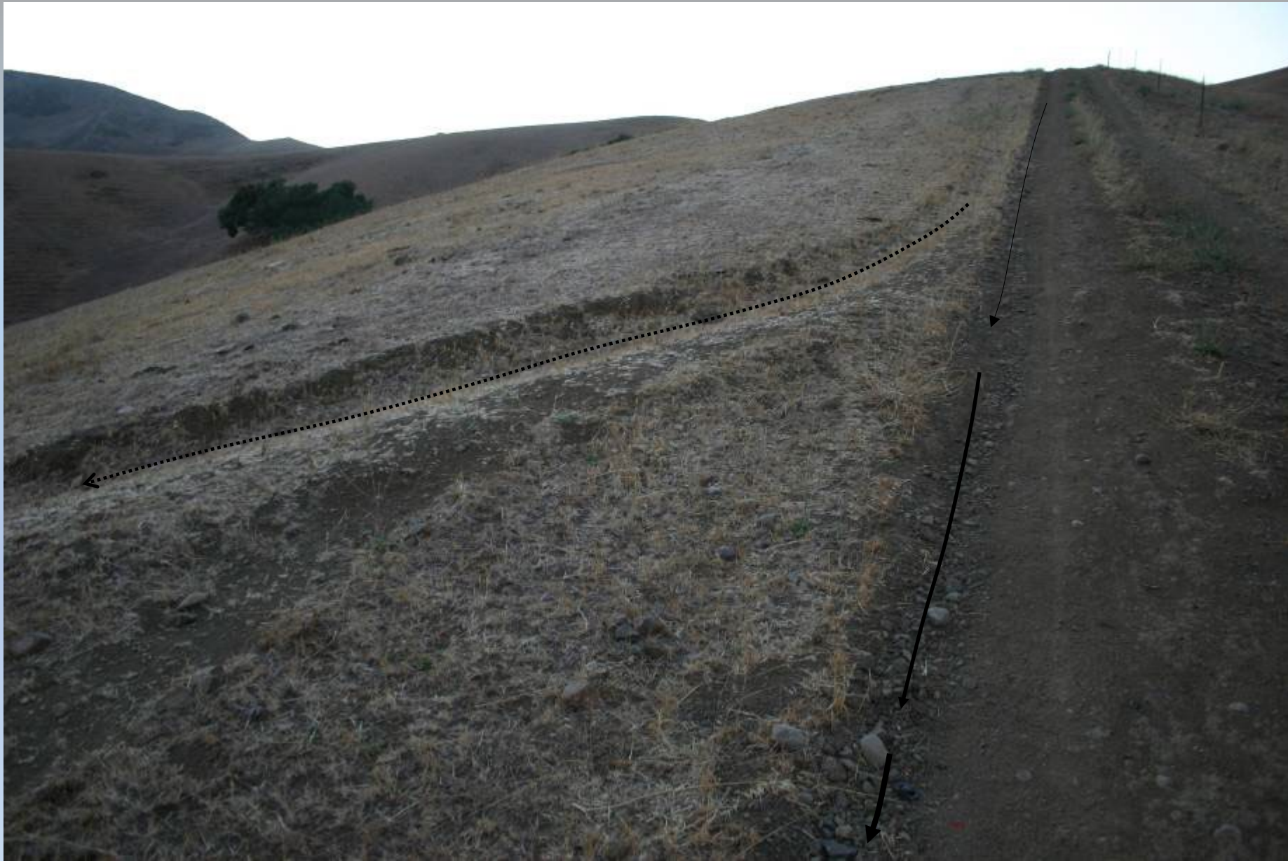
Berm Break defeated after grading
