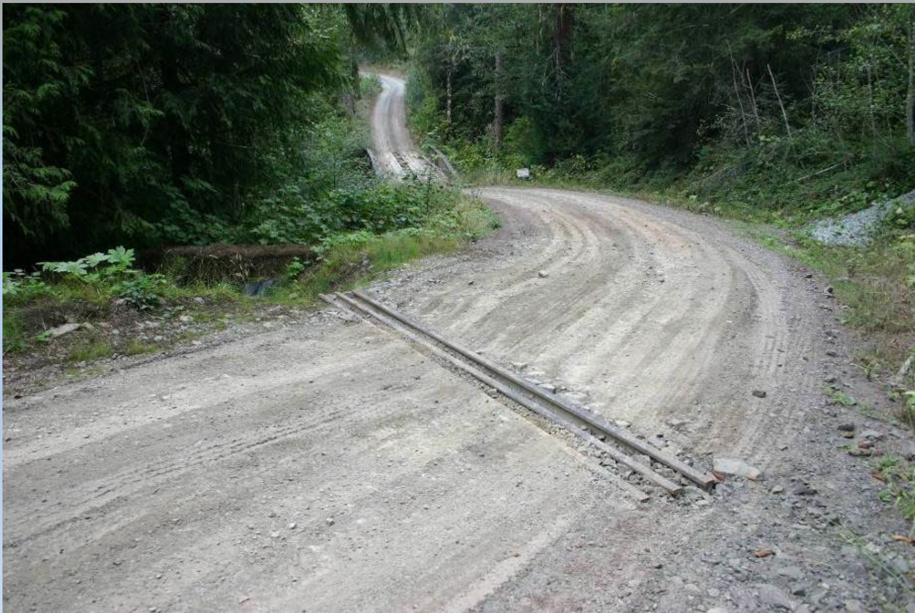
Slotted road drain and ditch infiltration gallery
