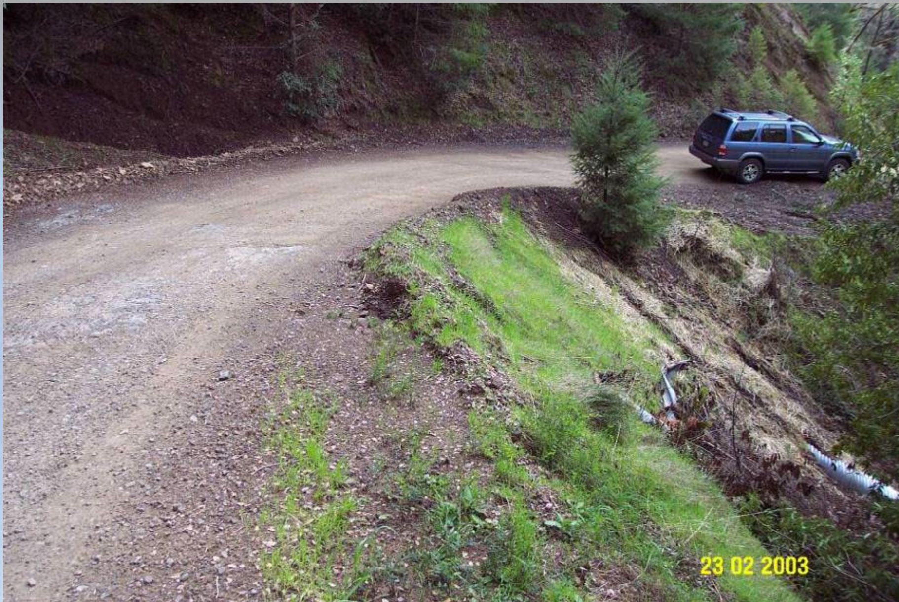
Bermed fillslope protecting stream crossing fill
