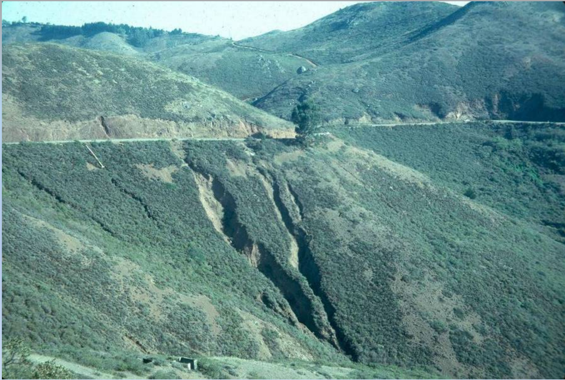
Gullies from road surface runoff
