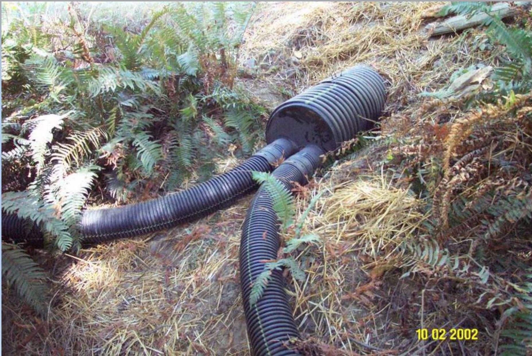
Perforated DRC flex pipe spreaders
