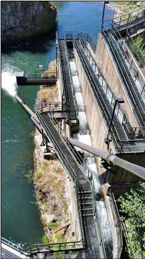
River Mill Hydroelectric Project Clackamas River, OR
