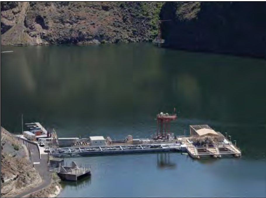
Pelton Round Butte Fixed Surface Collector Deschutes River, OR (photo by PGE)
