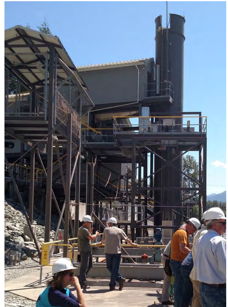
Lower Baker Adult Collection Facility Baker River, WA
