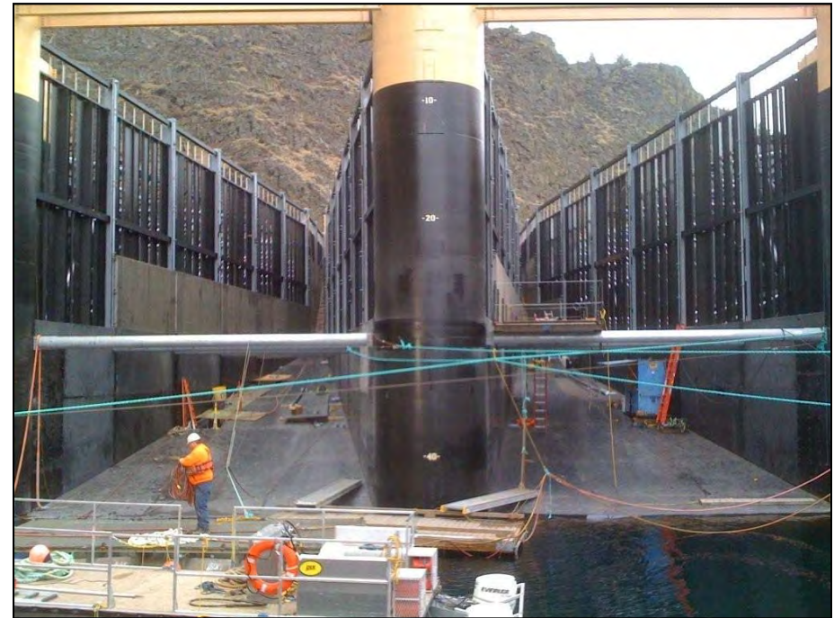
Entrance to Pelton Round Butte Fixed Surface Collector under construction (photo by PGE)
