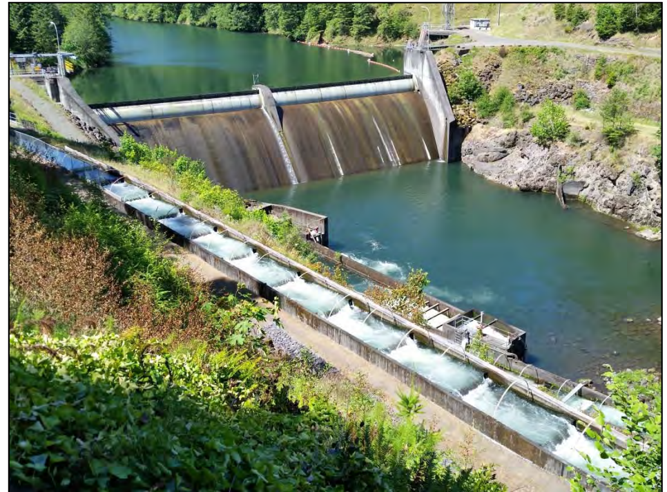
Faraday Diversion Dam and North Fork Fish Ladder Clackamas River, OR
