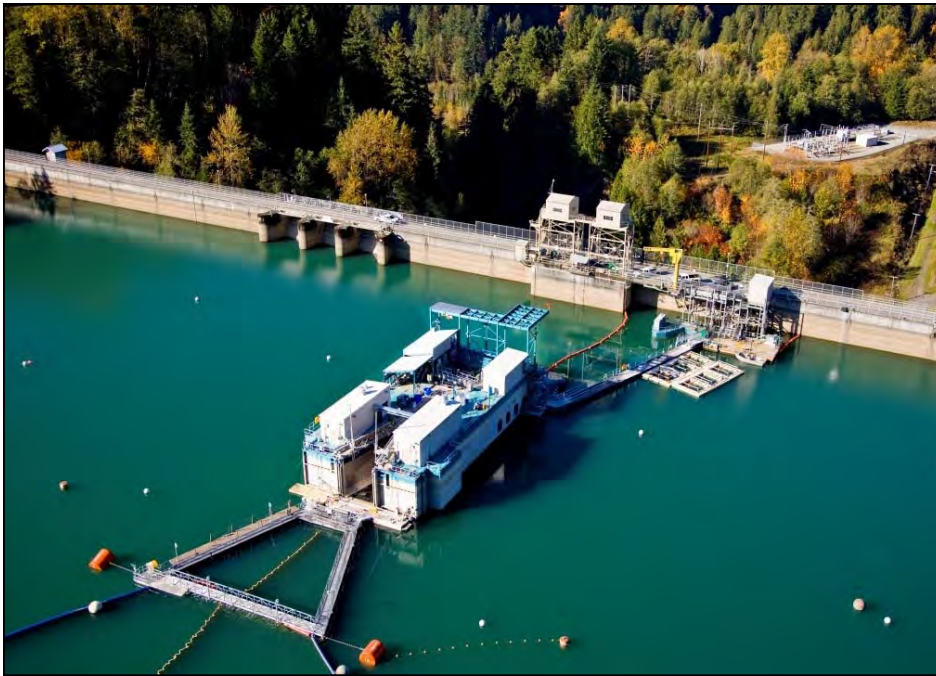
Floating Surface Collector Upper Baker Dam, WA (photo by PSE)
