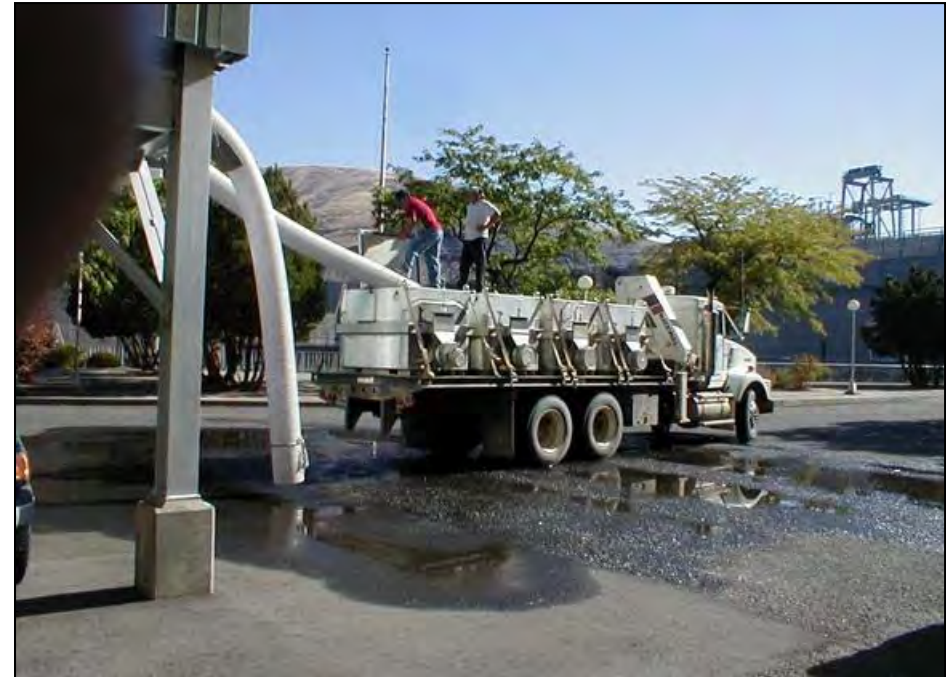
Lower Granite Dam Adult Collection Facility Snake River, WA
