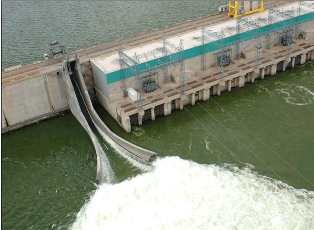
Juvenile Surface Spill Facility Wanapum Dam, WA
