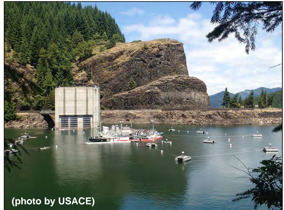
Cougar Portable Floating Fish Collector Cougar Dam, McKenzie River, OR
