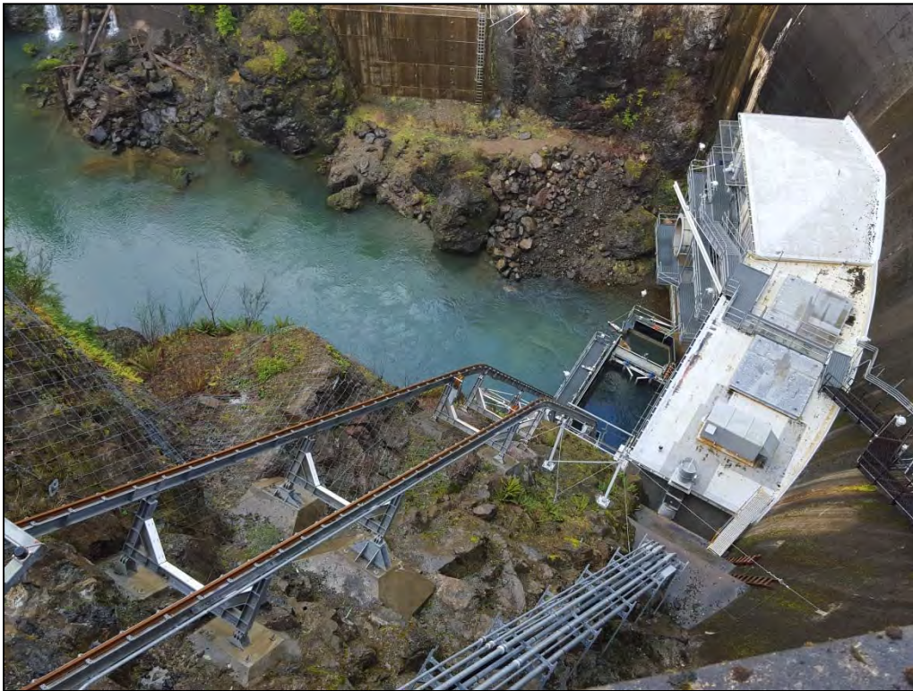
Cushman Dam No. 2 Adult Collection Facility Skokomish River, WA
