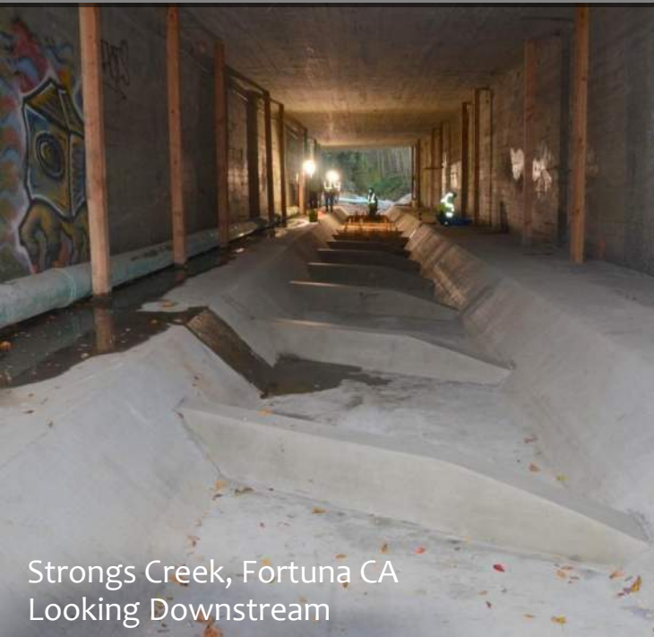
Example of a Baffled Transport Channel
