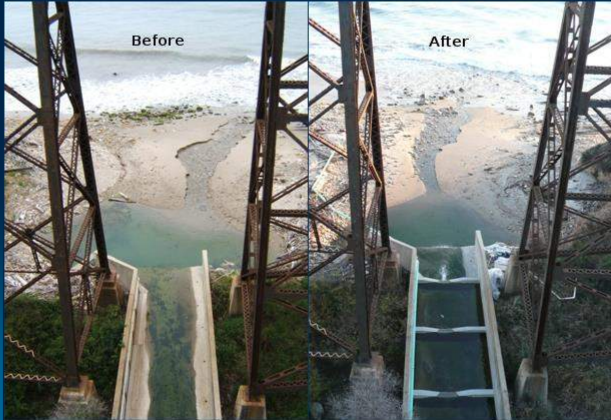
Fishway Entrance not backwatered when Lagoon Opened
