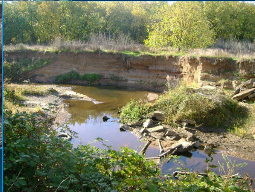
Stage III/IV Widening/Stabilizing
