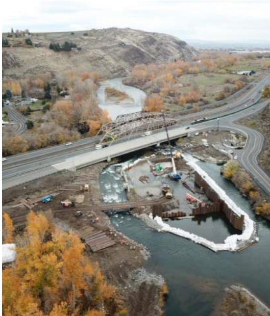
Phase 1: Care of Water October 22, 2021
