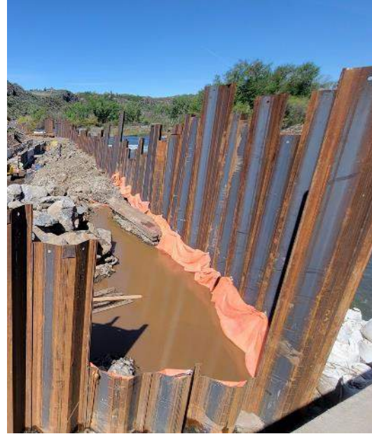
Temporary and permanent sheet pile walls
