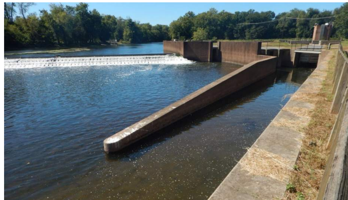
Shikellamy NLF: Photo courtesy of KC Construction
