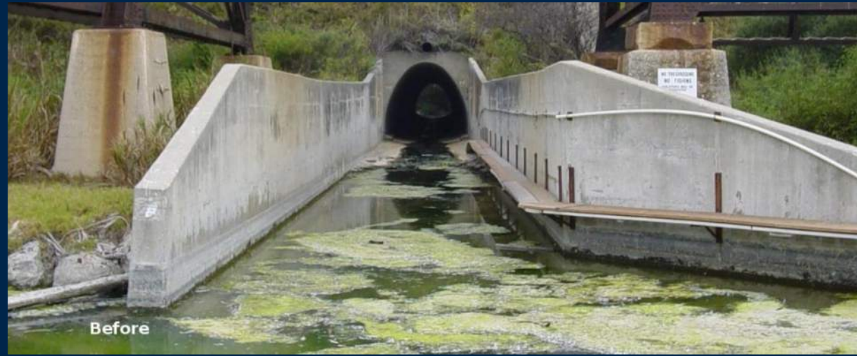
Before Project: Coastal Lagoon Mouth Closed
