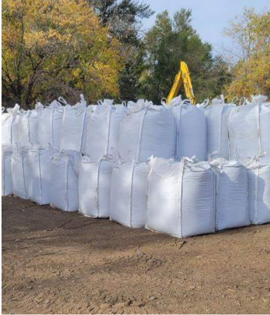
Over 2,700 supersacks used for cofferdams
