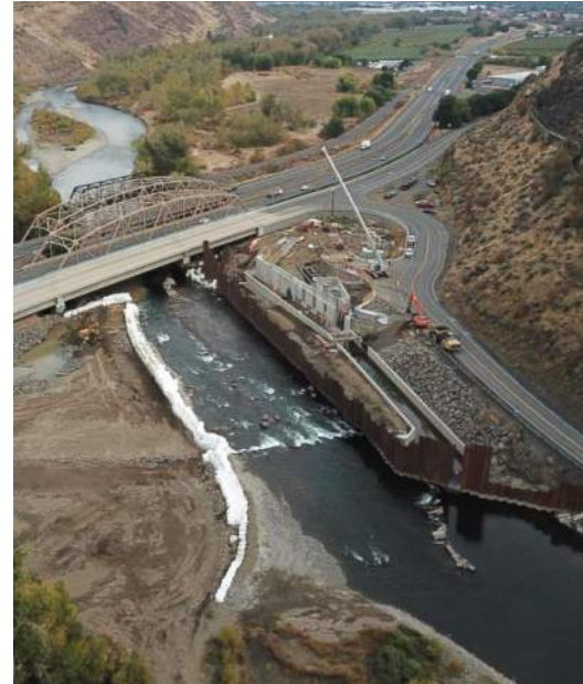
Phase 3: Care of Water October 24, 2022
