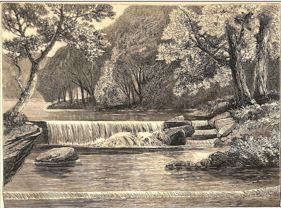
BRAAN WEIR AND FISH PASS.
