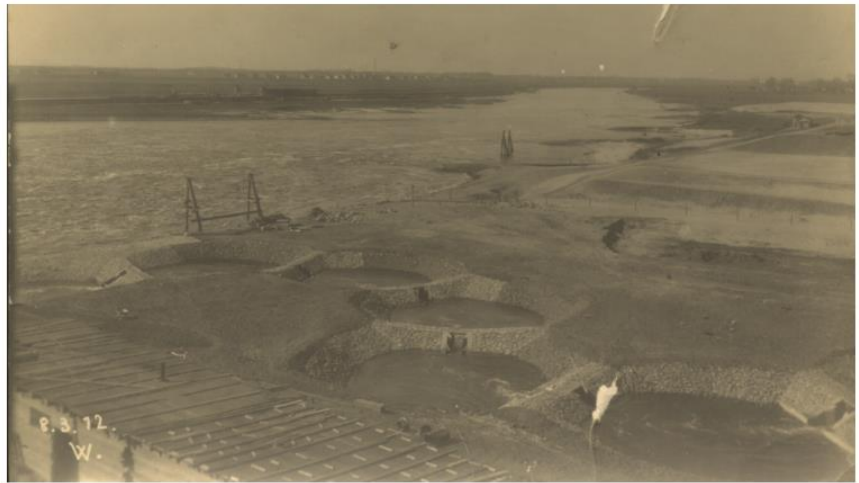
The bypass channel (Wildpass) at the Hemelinger Dam with its extensive and light-filled basins—a design that bears Landmark's signature.
