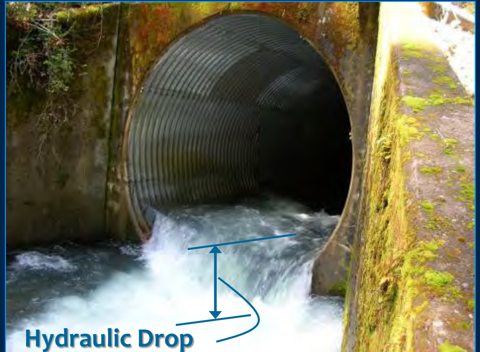
High Fish Passage Flow (excessive hydraulic drop)
