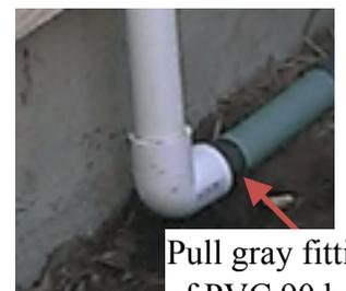
Pull gray fitting out of PVC 90 here to flush the system
