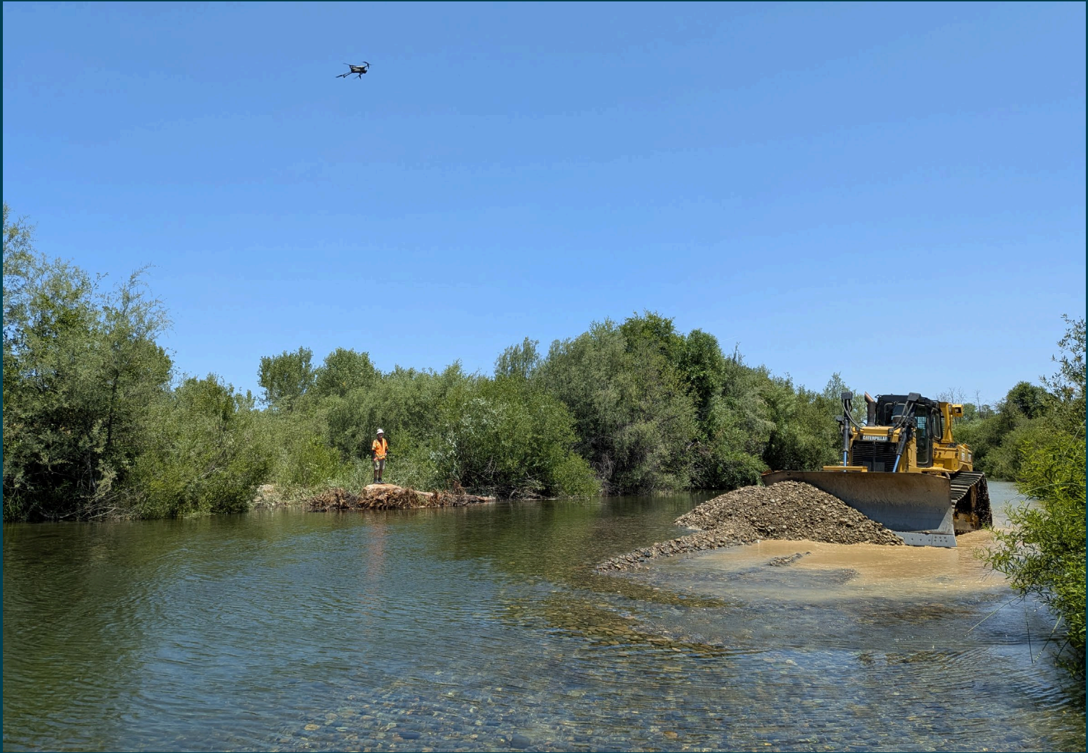
Adding coarse sediment to Bar 2 June 2025
