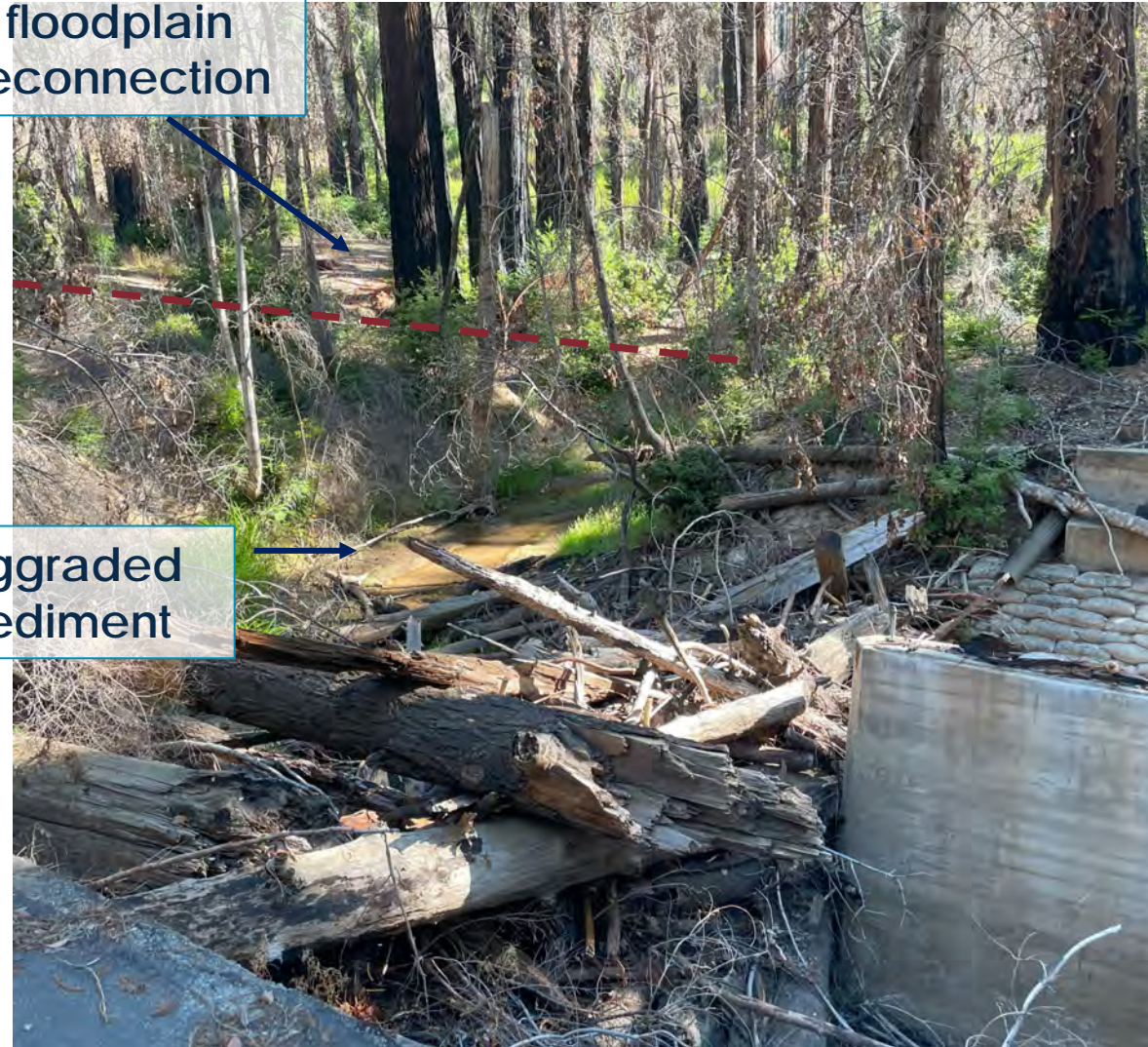
Sediment and wood trapped upstream of bridge
