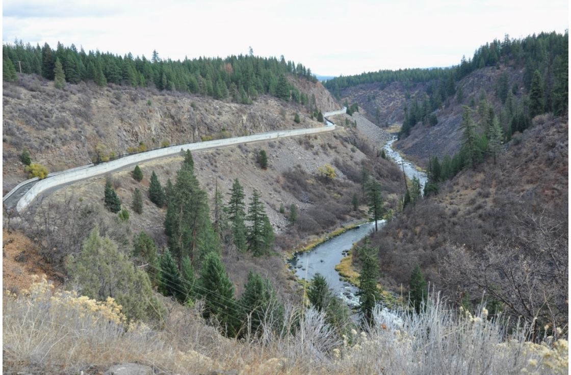
Klamath River between JC Boyle Dam and Powerhouse
