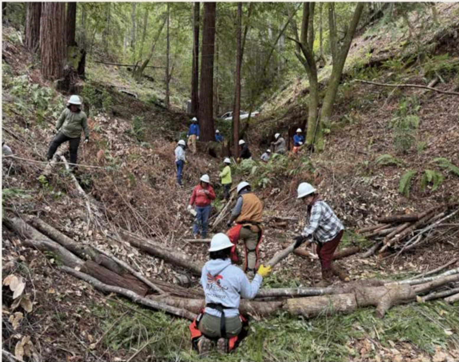
Resilience Works and North Bay Jobs with Justice stuff a gully at Monte Rio Redwoods Regional Park to mitigate the impact of a problematic road culvert that was causing significant erosion. Photo: OAEC/Brock Dolman
