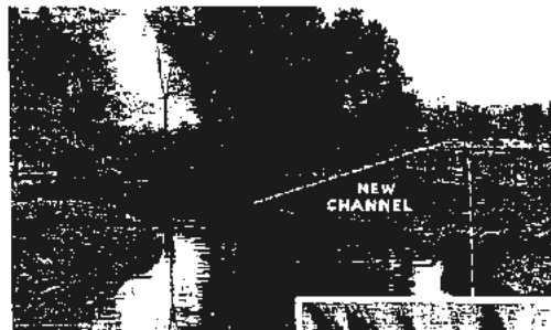
Straightening of Pequasset River in New Jersey by CCC workers stopped its yearly floods. Location of new channel is seen on right. Note temporary dam at left to provide volume of water for scouring blasted channel.
