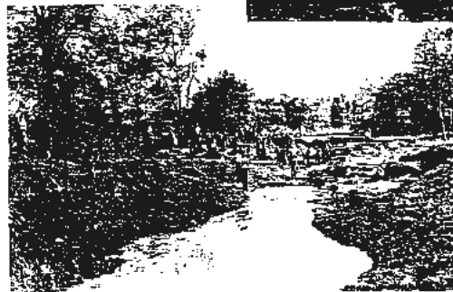
Immediately after explosion, water is entering new channel, whose banks will be smoothed and "stream-lined" by the speedier flow of water.
