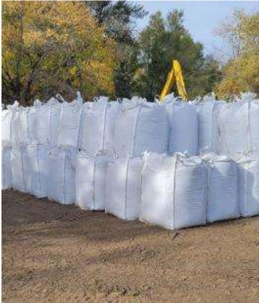
Over 2,700 supersacks used for cofferdams
