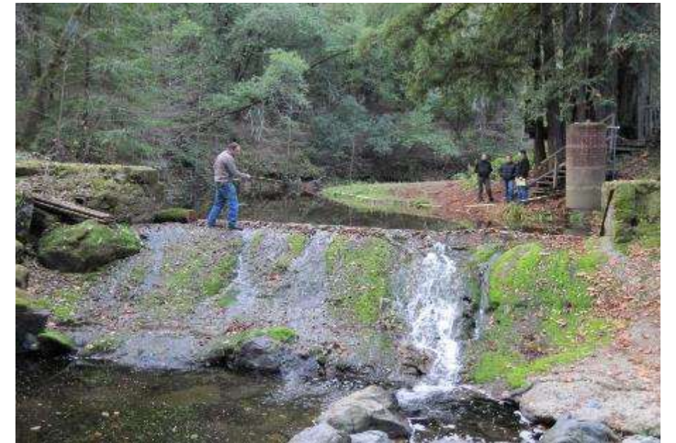
2009. Mill Creek dam apron
