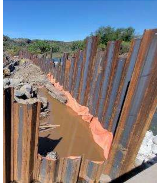
Temporary and permanent sheet pile walls
