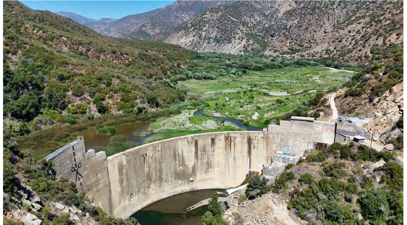
2024: Dam crest <50m, Reservoir full of sediment
