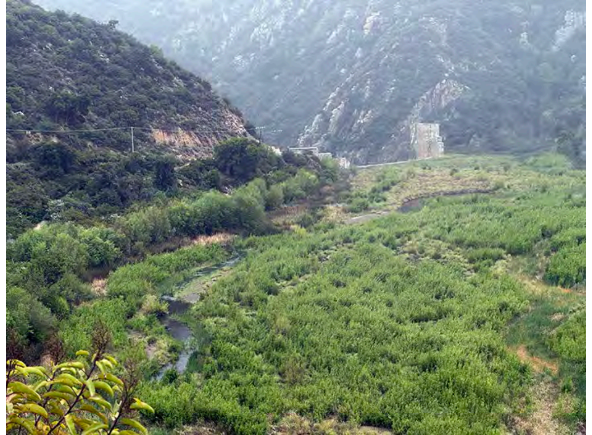
Vegetation growth and sedimentation in reservoir near dam crest
