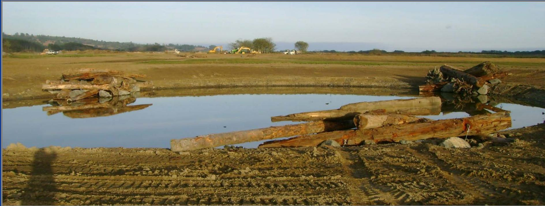
Logs Anchored together and cabled to 2-Ton Rocks. Each log required one 2-Ton Rock to counter buoyancy
