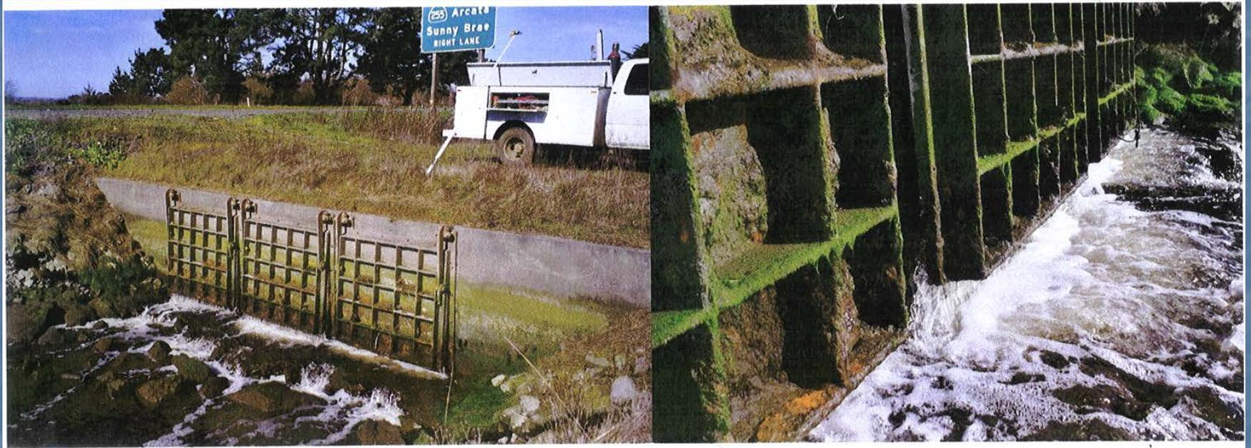
The old tidegate systems were bad for fish passage because they had a poor conveyance to size ratio which meant they had poor water flow.
