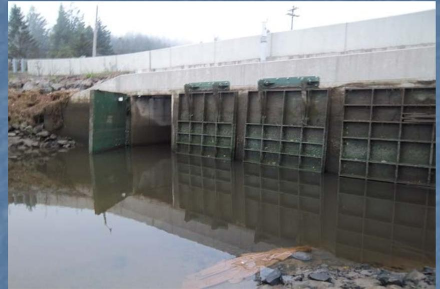
Top Hinge Side Hinge Array with MTR
