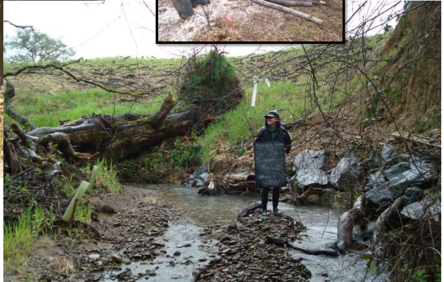
Bioengineered Bank Stabilization, Anderson Creek, Navarro River, 2005
