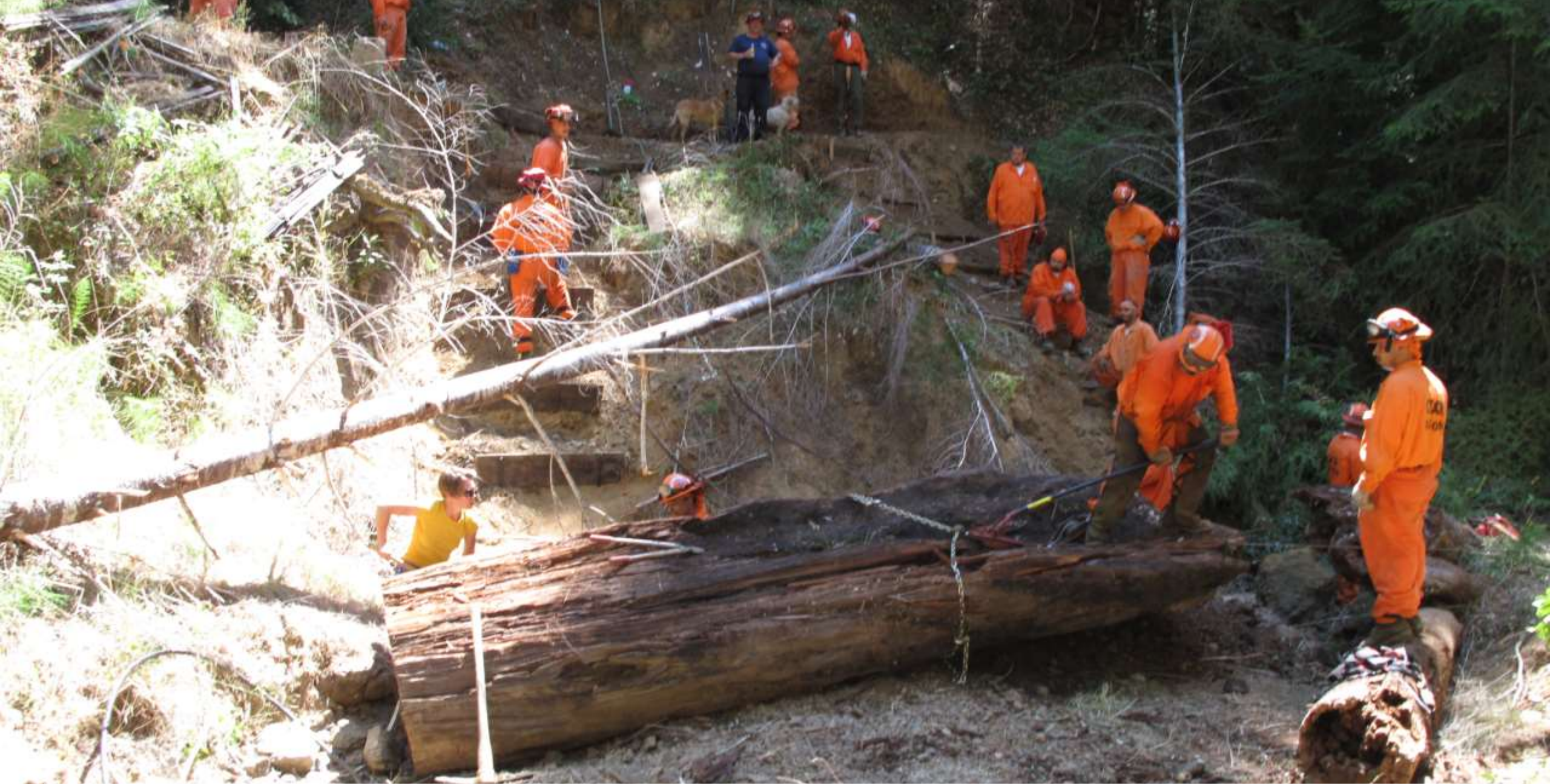
Bioengineered Bank Stabilization, Honey Creek, Navarro, 2008
