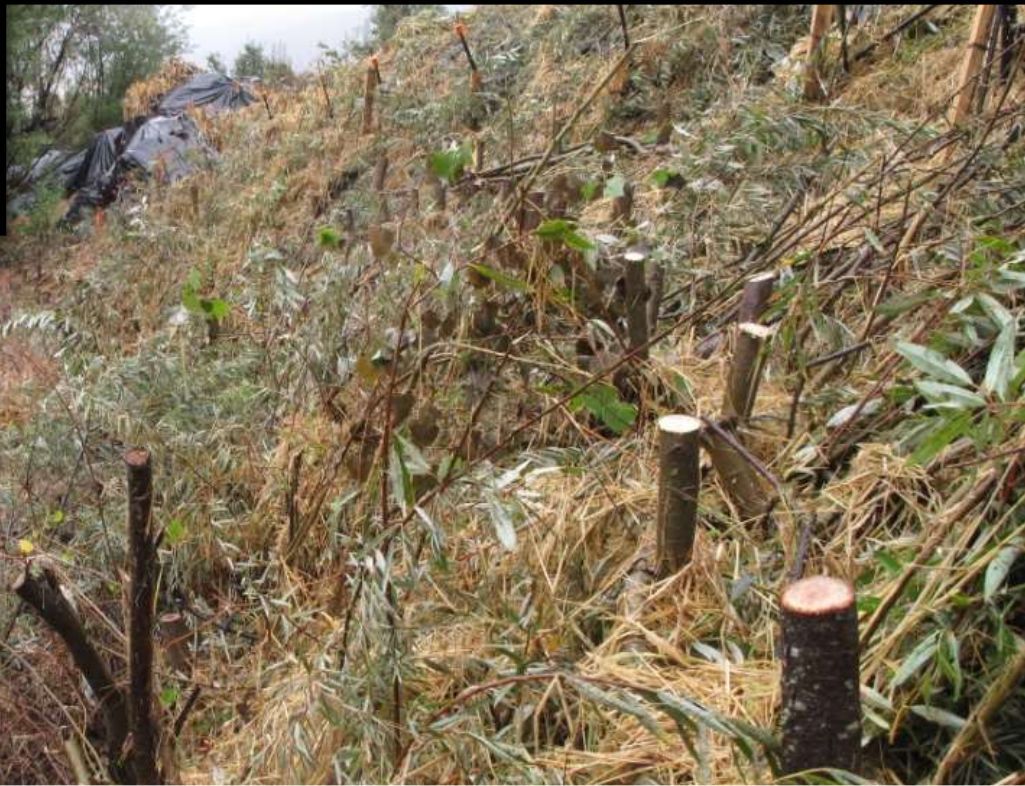
Bioengineered Bank Stabilization, Russian River, 2011
