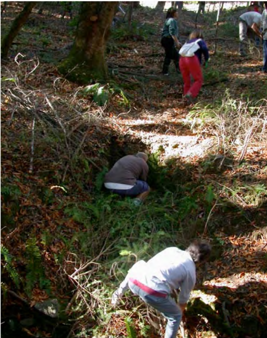
Students tightly stuffing and stomping fir into the gully
