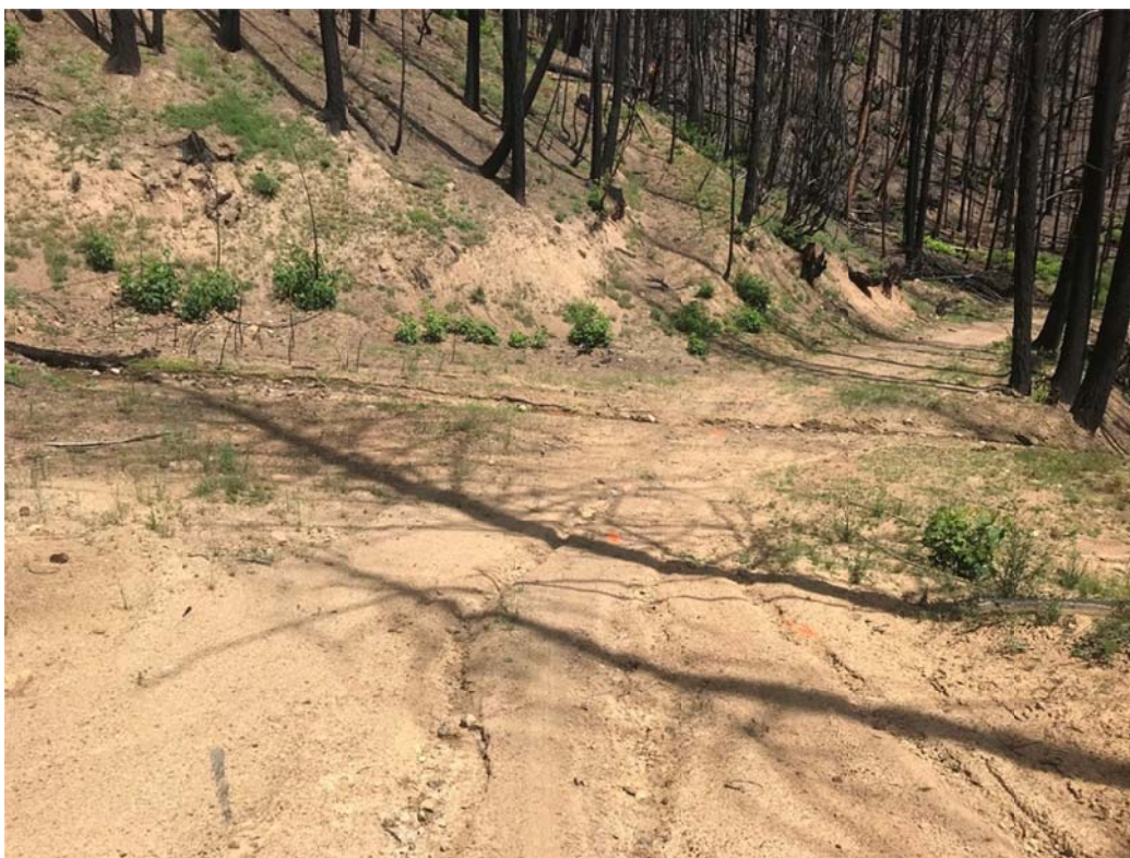
Figure 3 (above): A very large fill in a stream channel (with two logging roads entering it) with significant incision and large volumes of sediment capable of delivering to Deadwood Creek. This site also has diversion potential down the road (Site 200.5).
