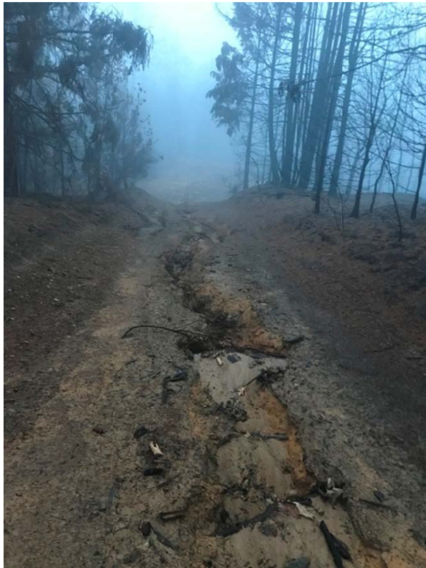
Figure 10. Significant gully erosion down the PG&E power line. The location of the road on a ridge line minimizes sediment delivery to a stream.
