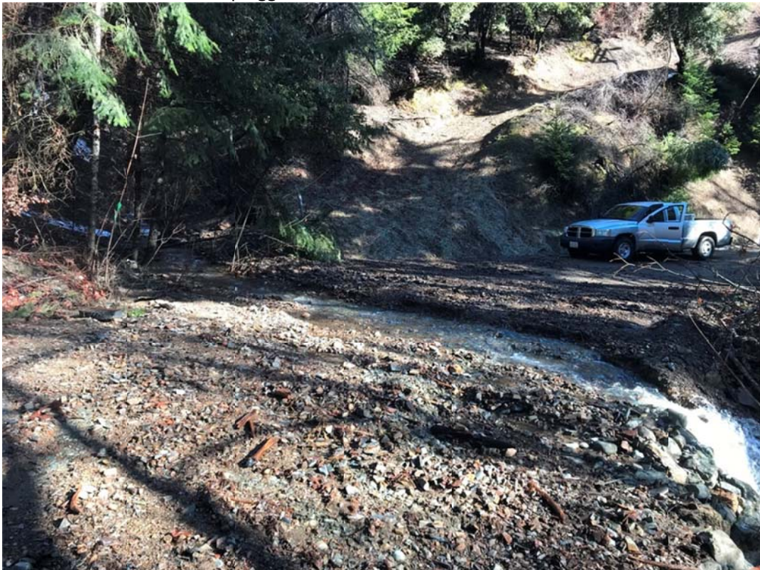
Figure 16 (above) and Figure 17 (below): Diverted streams on Deadwood Road. Site 1490 Donnelly Gulch plugged culvert and washed out fill.
