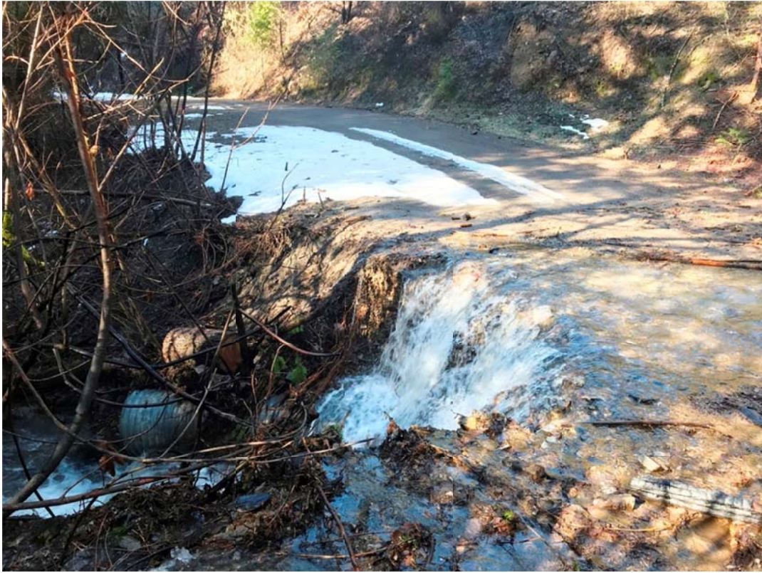
Figure 16 (above) and Figure 17 (below): Diverted streams on Deadwood Road. Site 1490 Donnelly Gulch plugged culvert and washed out fill.
