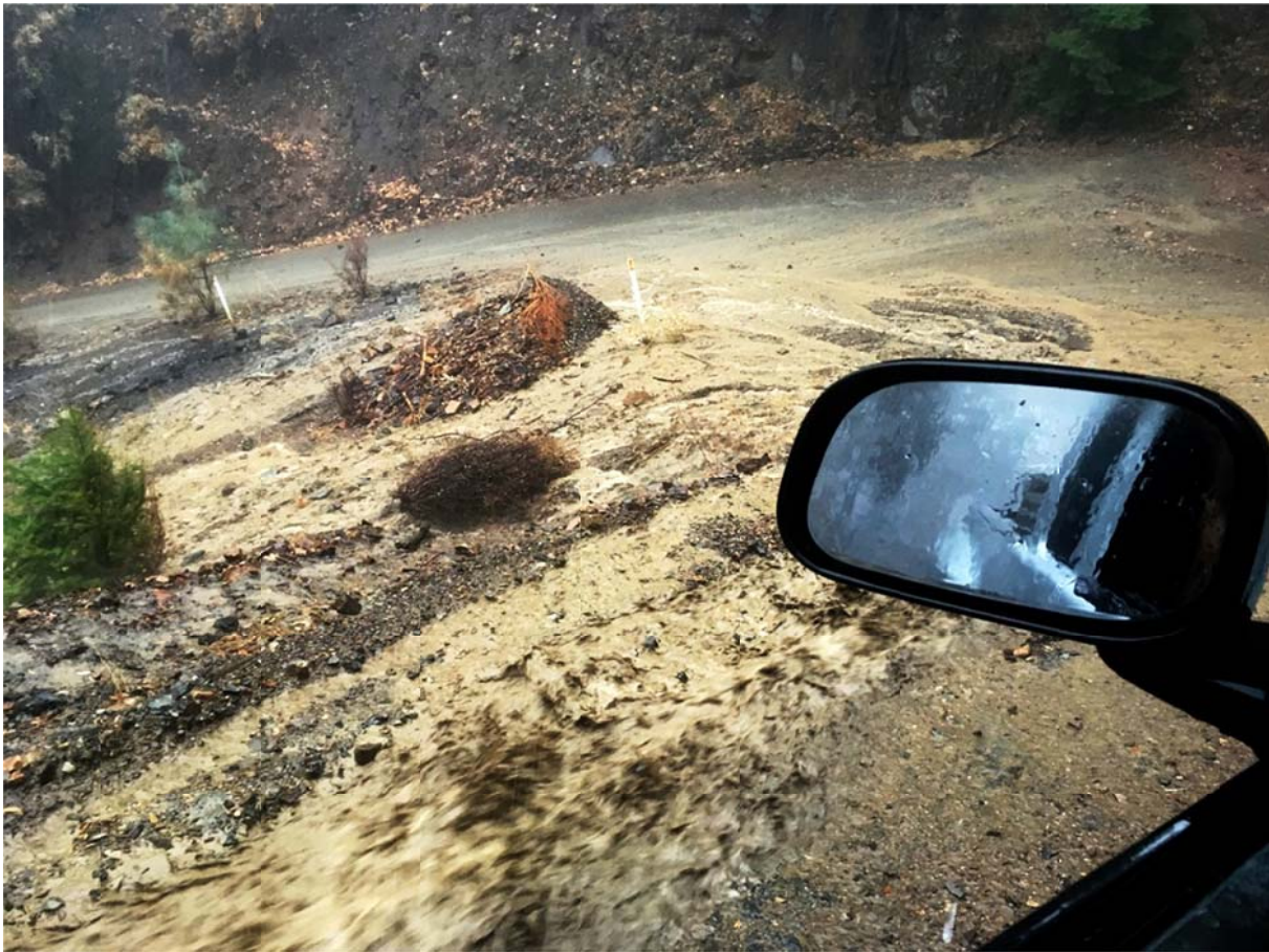
Figure 13 (above): Tunnel Gulch crossing October 4, 2018. The culvert has been completely plugged and diverted both over the road and down the road.
