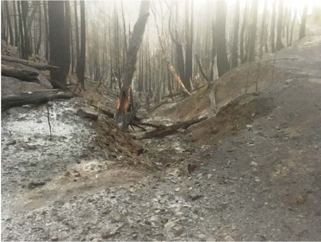
Figure 7 (above): Road crossing on the 400 Road showing aggraded fill and bank failure.
