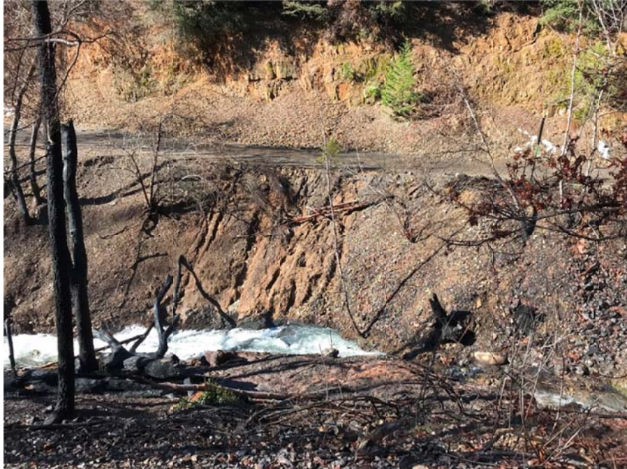
Figure 5 (above): Site 1490 on Deadwood Road. Plugged culvert crossing and diverted stream channel. Figure 6 (below): Site 1490 diverted stream channel re-entering the stream downstream of the road crossing.
