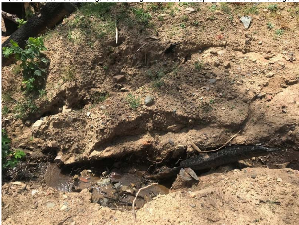
Figure 4 (below): The same site as Figure 3 showing ~4' wide by 4' deep incision at the lower edge of the fill.
