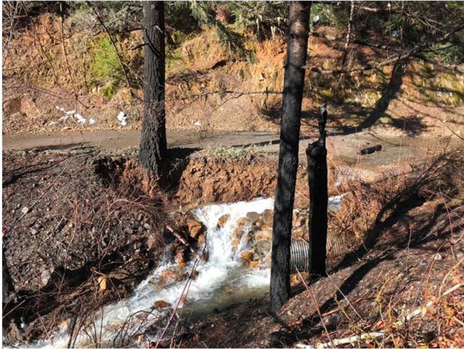
Figure 5 (above): Site 1490 on Deadwood Road. Plugged culvert crossing and diverted stream channel. Figure 6 (below): Site 1490 diverted stream channel re-entering the stream downstream of the road crossing.
