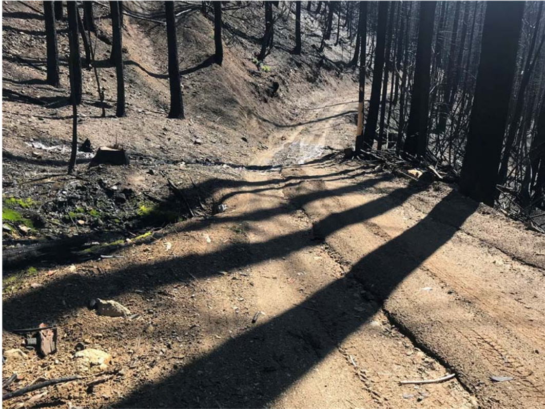
Figure 1 (above): A rill/gully (center of photo) on the 200 Road (Site 200.4). The site also contains a diverted stream crossing and a non-functioning 24" CMP culvert crossing.
