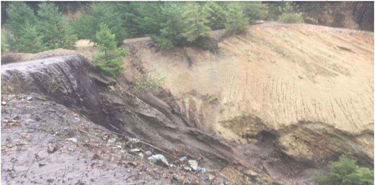
Figure 12 (below): Mill Gulch crossing outlet overtopped and flow returning over road top.
