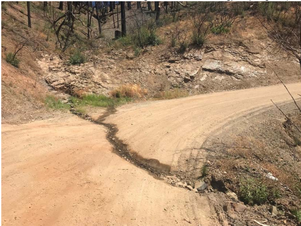
Figure 2 (below): A non-culverted stream crossing in bedrock with a critical dip and minimal future erosion potential in the road. Note the outlet of the crossing can be treated with energy dissipating rock (site 1498).
