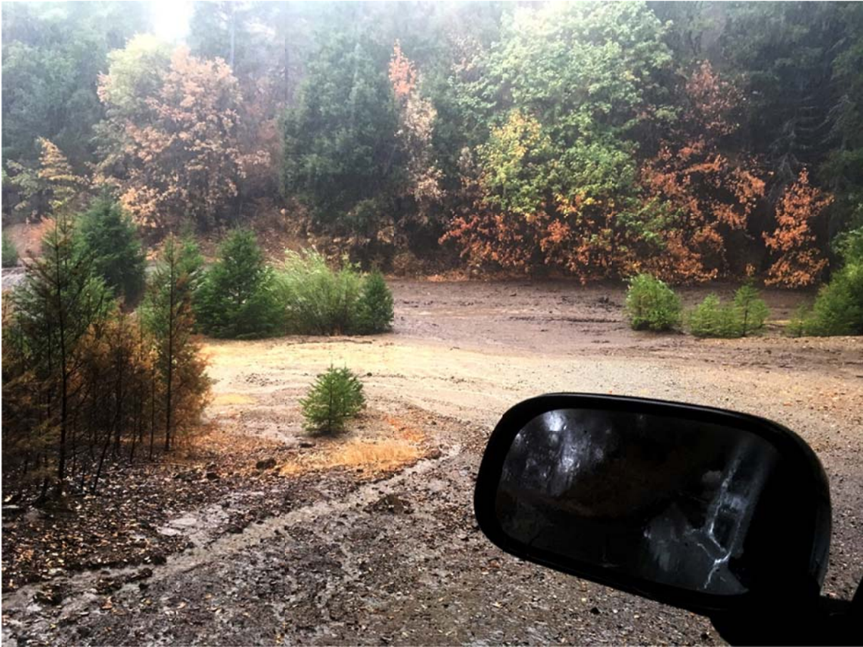
Figure 11 (above). Mill Gulch stream crossing at Deadwood Road, October 4, 2018. The culvert plugged and the channels diverted west and down the road (note the dark ash laden sediment in the middle distance and the lighter yellow road erosion sediment in the middle foreground).
