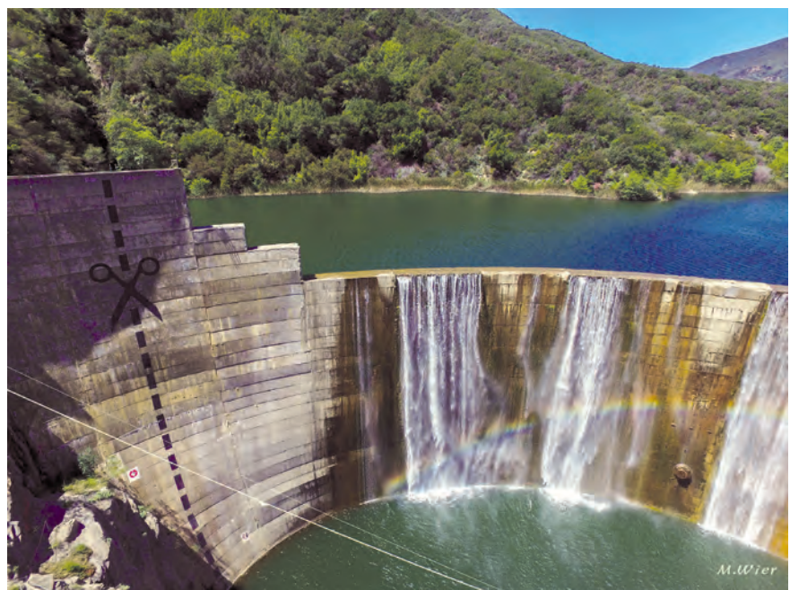
Matilija Dam in Ventura County Photo: Mike Wier
