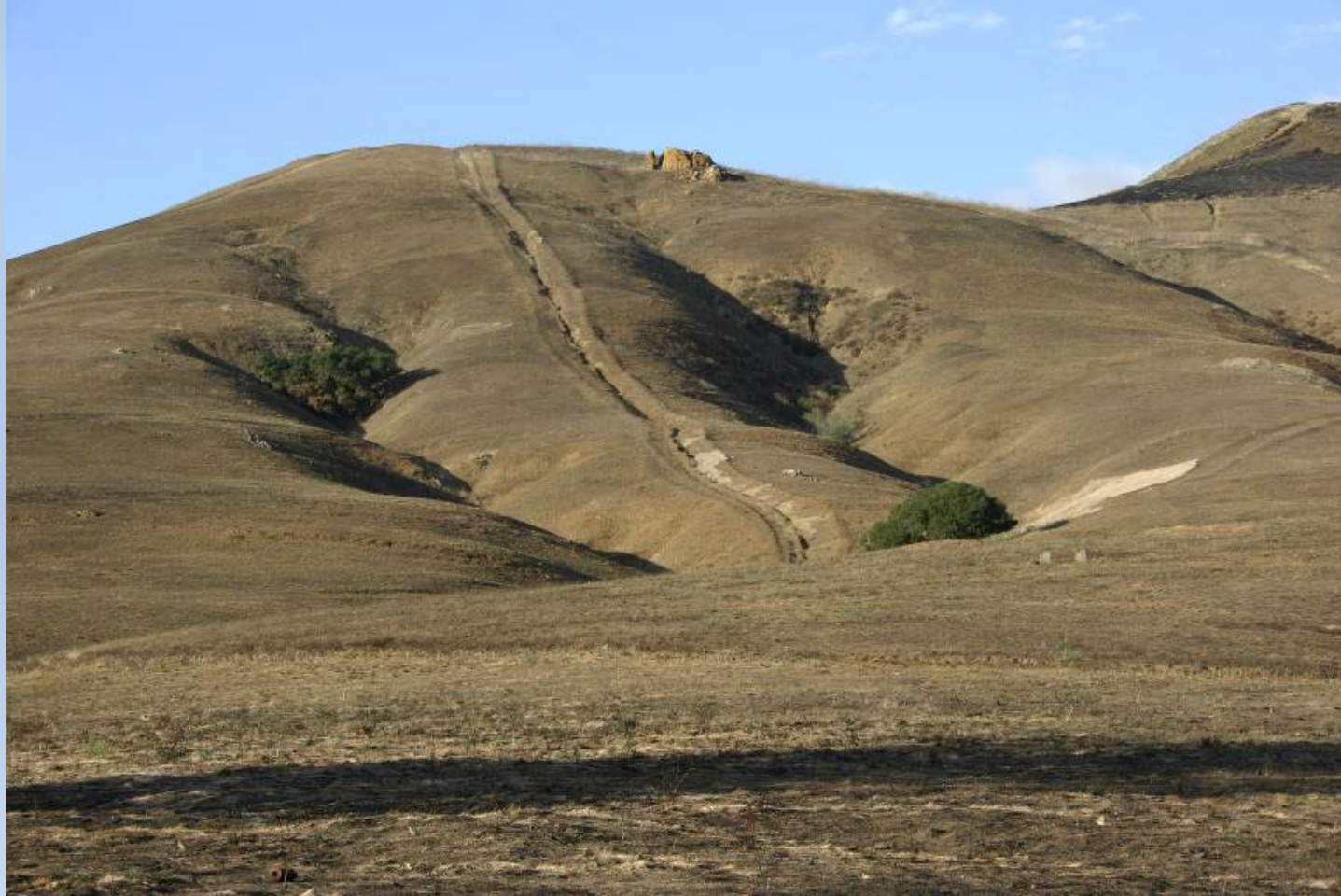
Road Surface Gullying in "fall line" road
