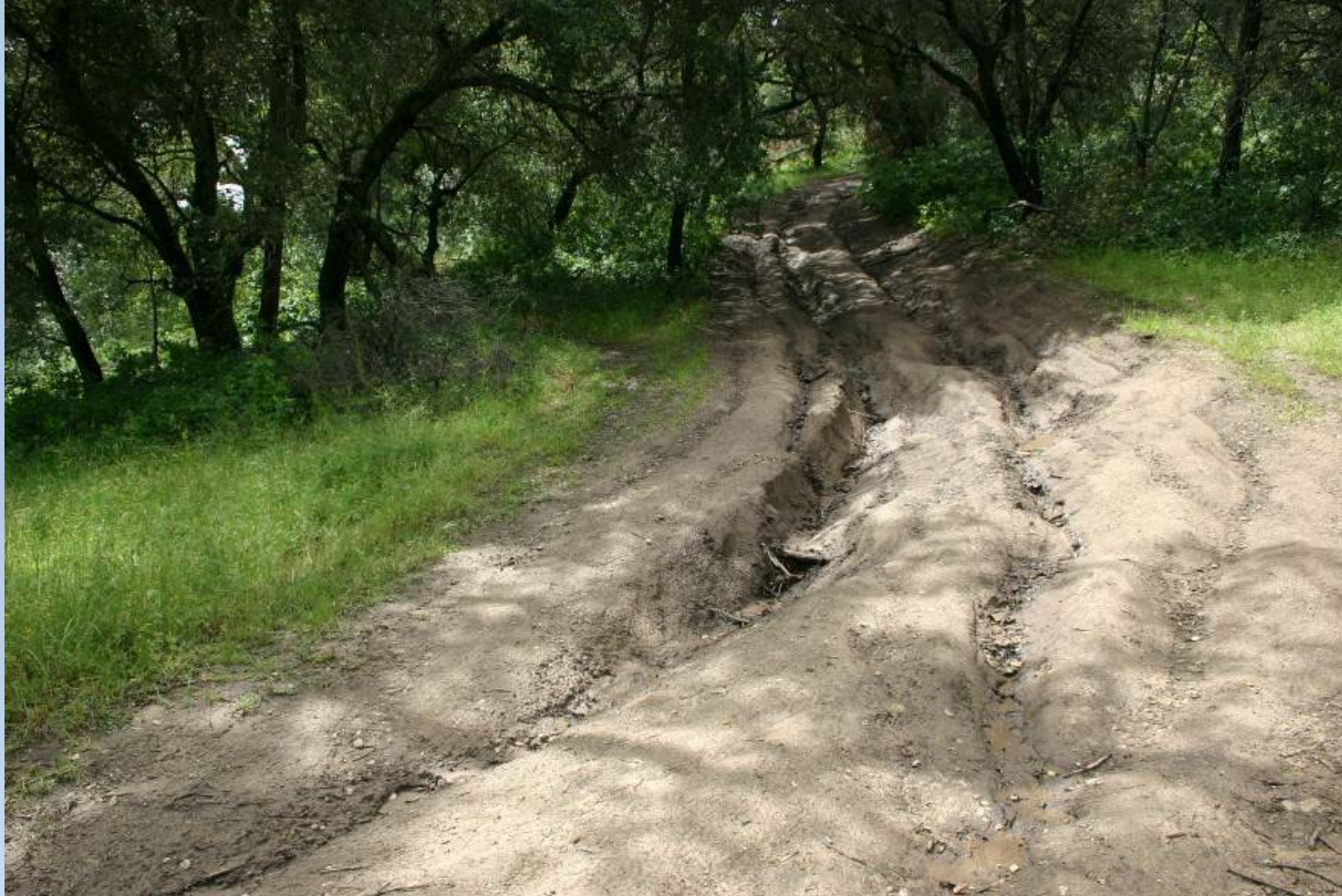
Road Surface Rilling and Gullying
