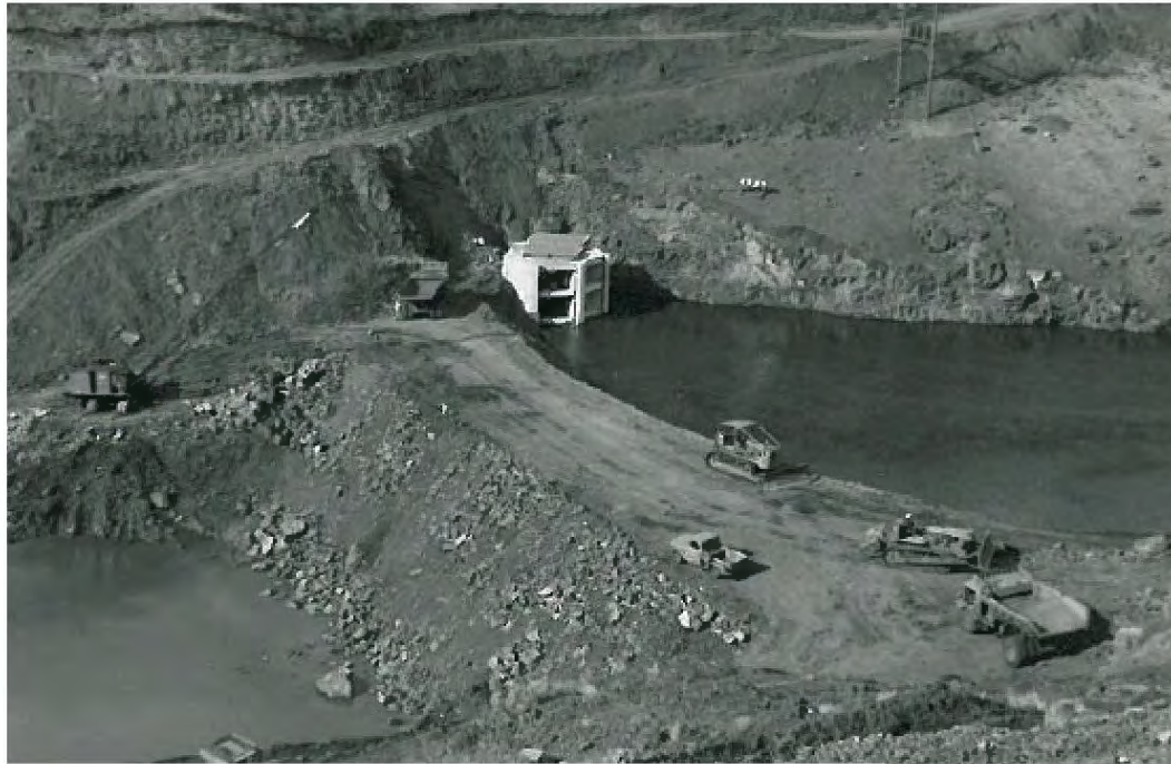
Iron Gate Dam diversion tunnel intake with cofferdam across Klamath River
