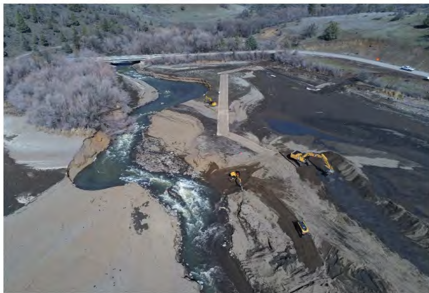
Sediment Evacuation and Fish Passage Impediment Removal
