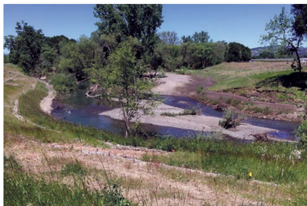
Riparian corridor expansion and increased channel complexity for velocity refuge and improved food production. Credit: Jorgen Blomberg
