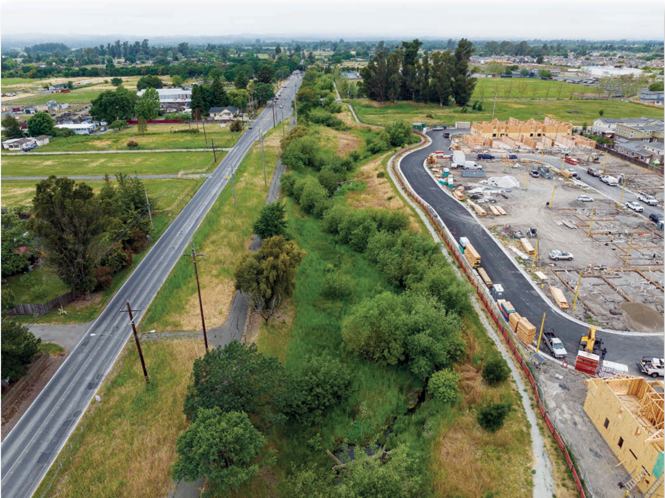
Lower Colgan Creek Restoration in southwest Santa Rosa. Credit: City of Santa Rosa
