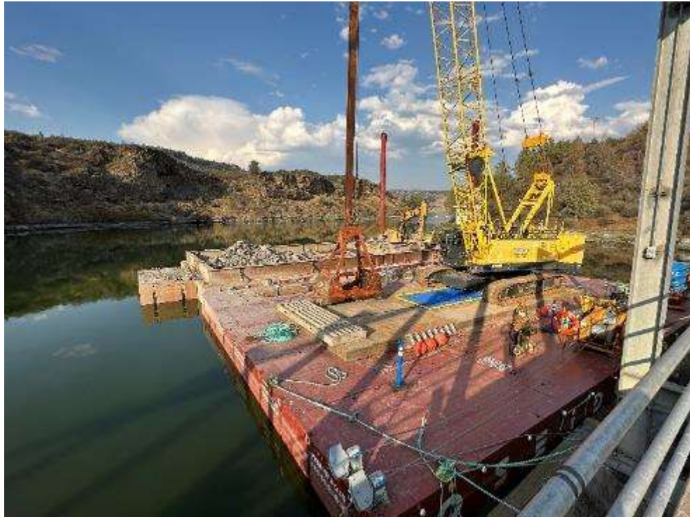
Dredging and debris barges moored at Copco 1 Dam while dredging in front of the new low-level adit. Debris, including rock and timbers, can be seen in the debris barge.
