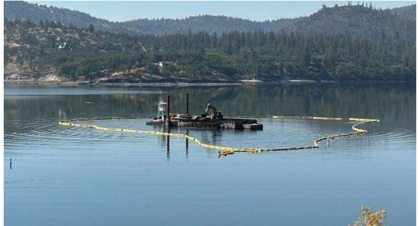
Offloading debris barge in dredging disposal area. 30 August 2023
