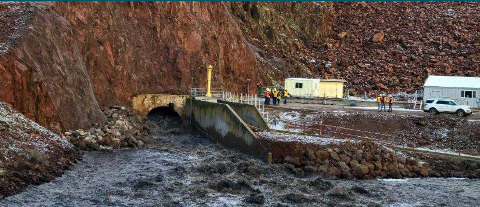
IRON GATE DAM KLAMATH RIVER, CALIFORNIA
