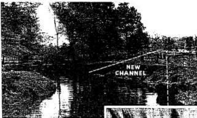
Straightening of Pequess River in New Jersey by CCC workers stopped its yearly floods. Location of new channel is seen at right. Note temporary dam at left to provide volume of water for scouring blasted channel.
