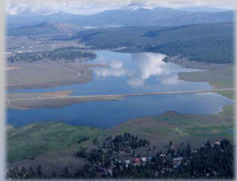
Reservoir Operations (1972-1996, during test fills and extreme storms)
