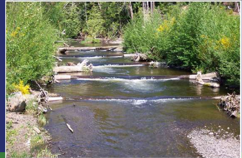
Figure XII-34. Goldsborough Dam Removal Project. An example of V-shaped rigid weirs.
