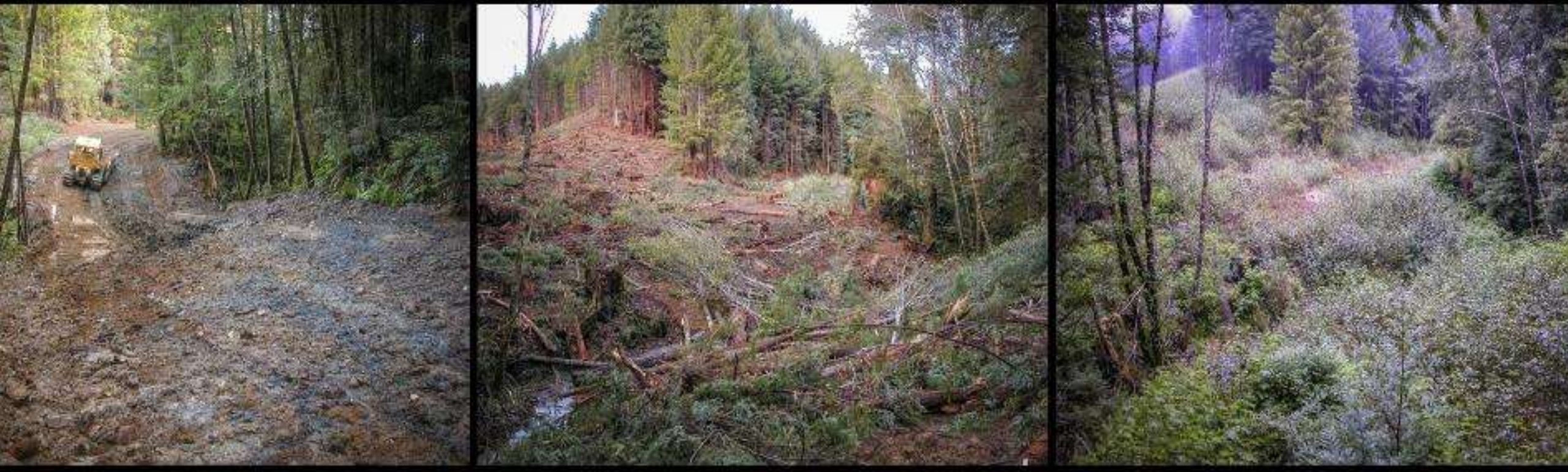
Road removal at Larry Dam Creek in Redwood National Park
