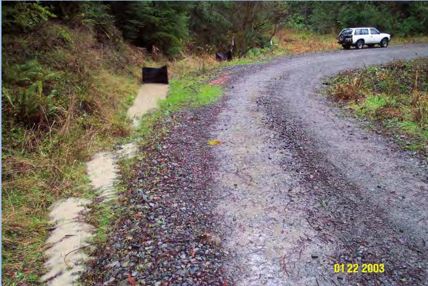
Silt fence ditch filter
