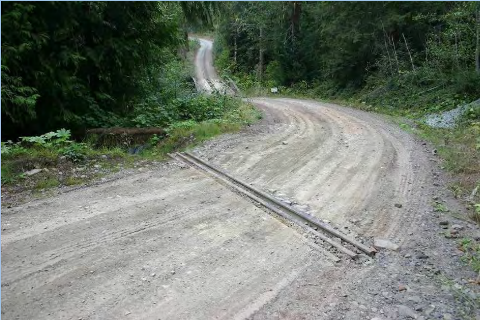
Slotted road drain and ditch infiltration gallery
