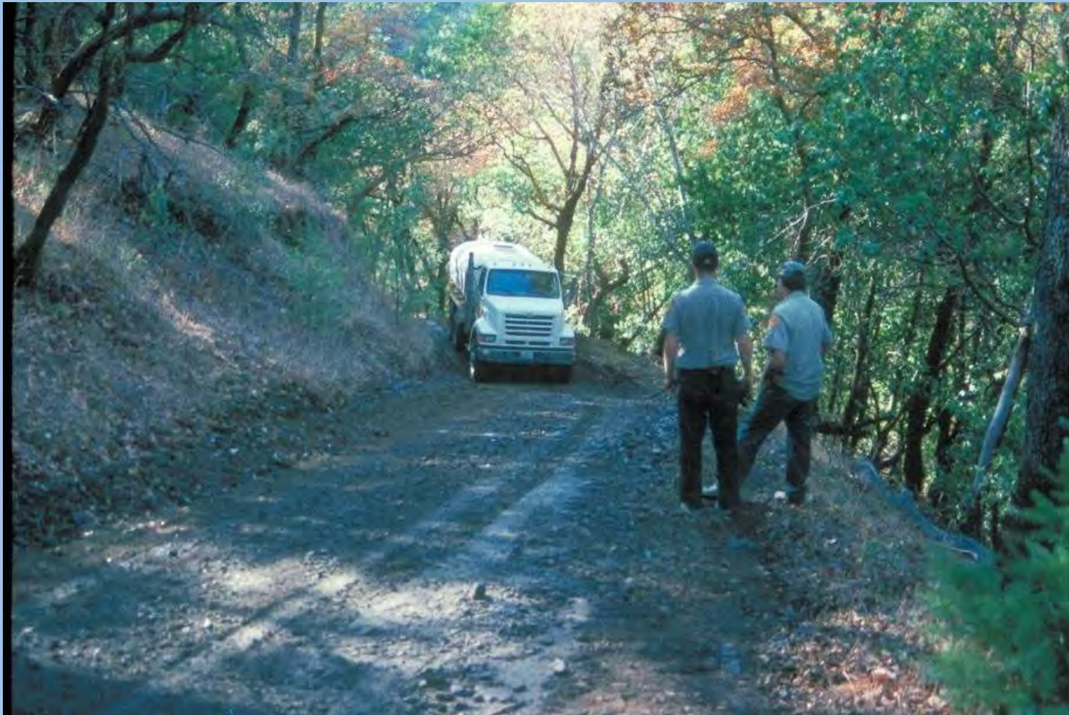
Rolling dip: watering for compaction
