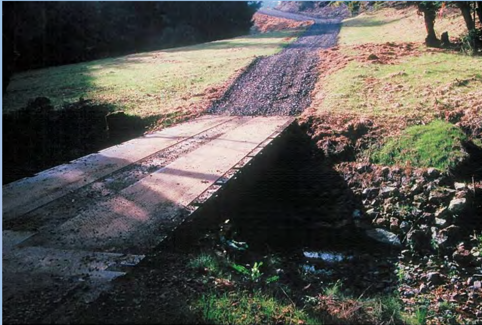
Rolling dips on a stream crossing approach
