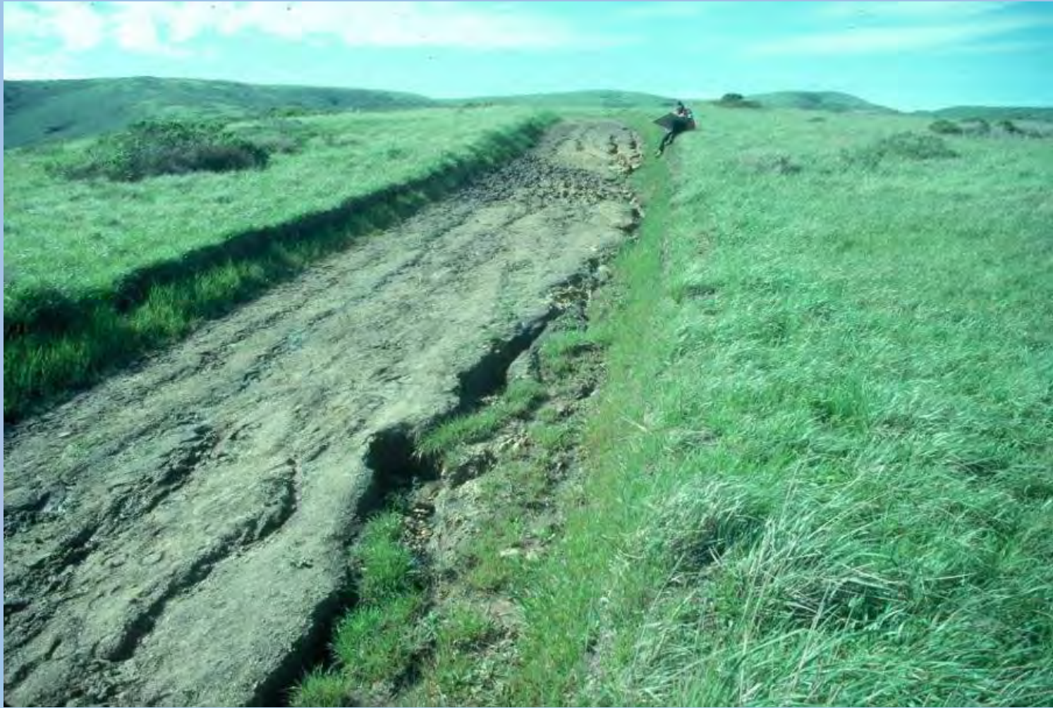
Draining through-cuts
