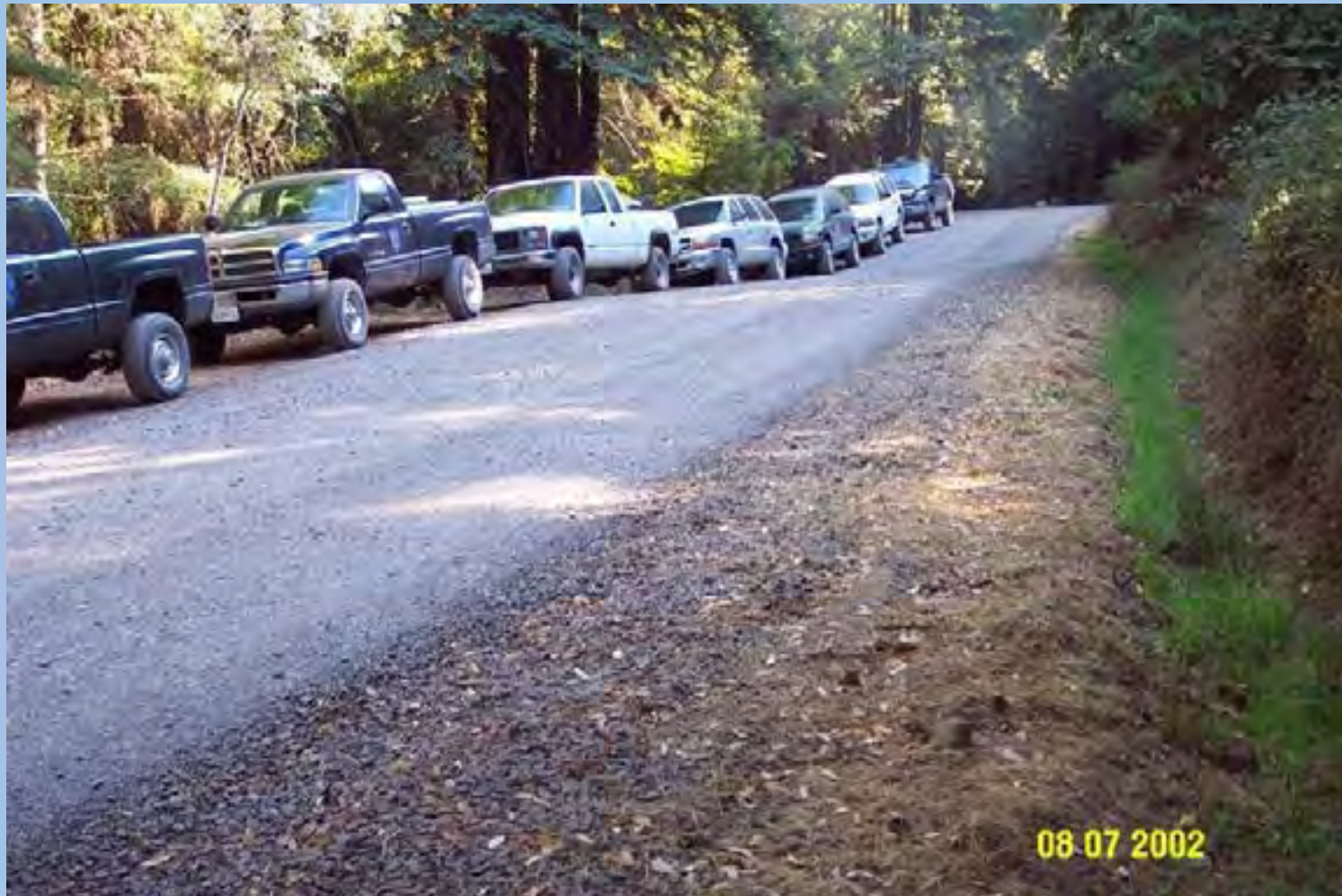
Outsloped, rolling dip and inside ditch
