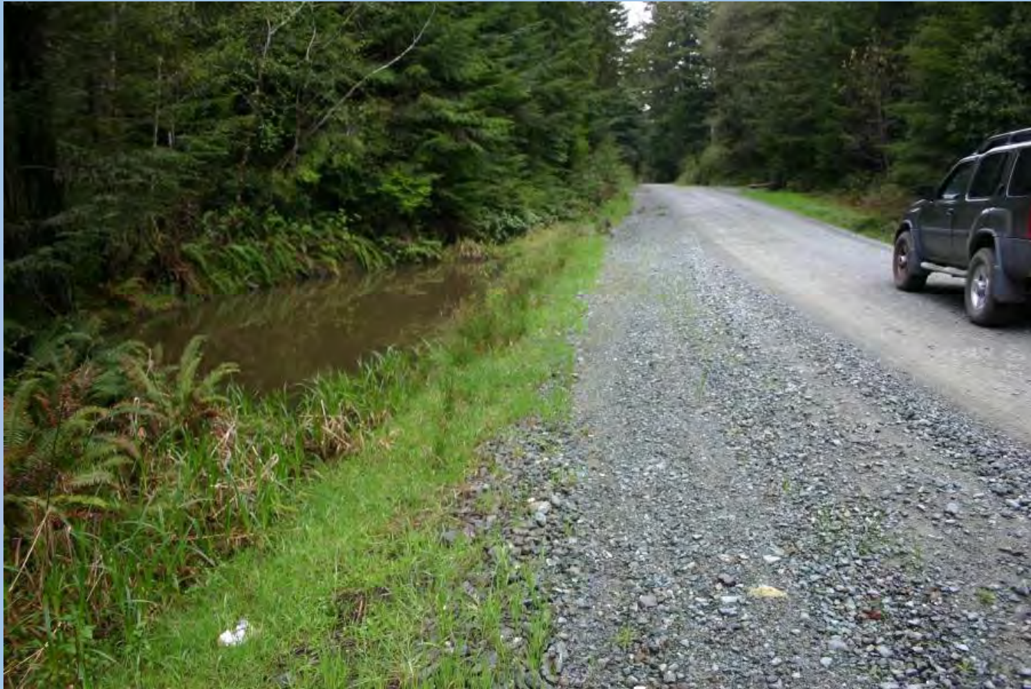
Roadside sediment retention basin
