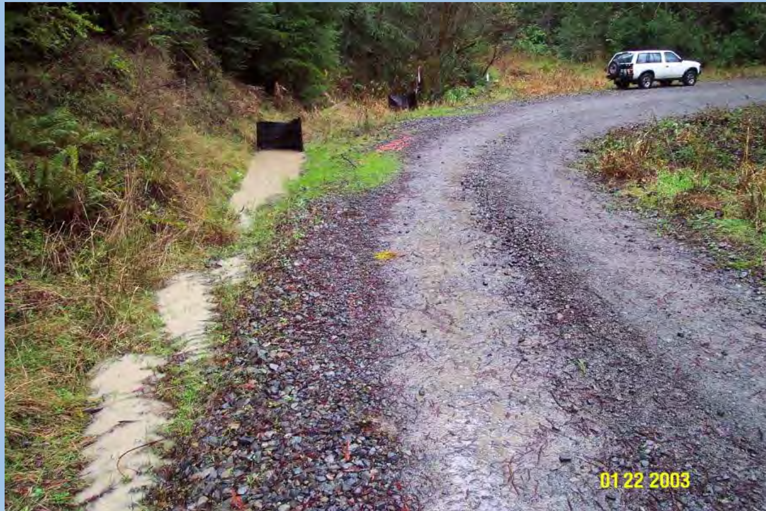
Silt fence ditch filter
