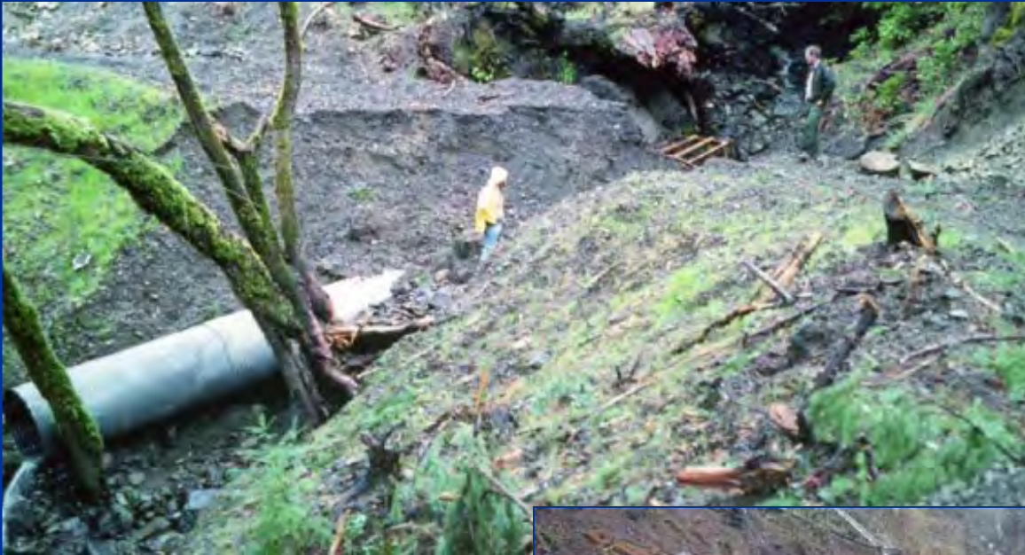
Wash out (eroded) stream crossing
