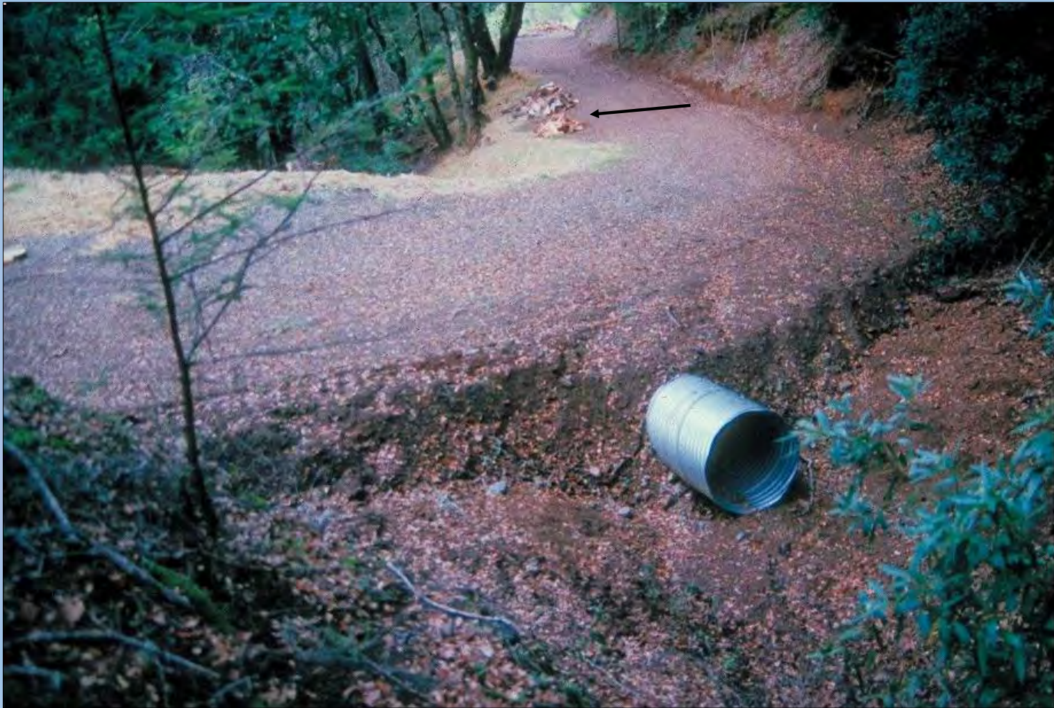
Critical dip down-road from crossing
