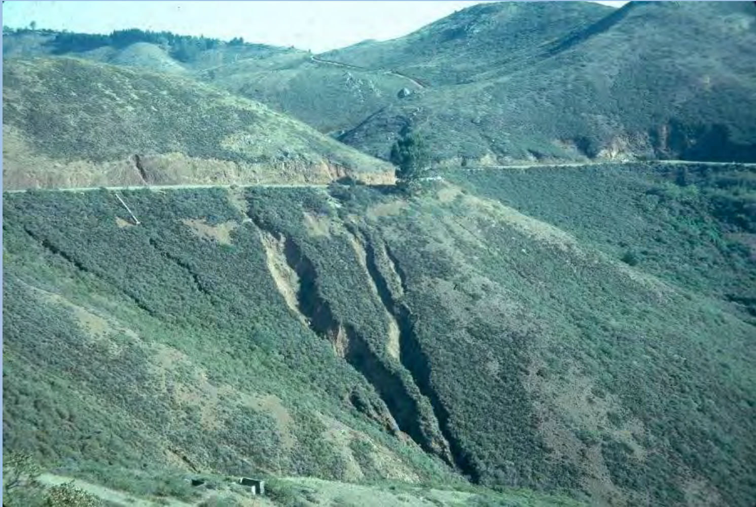
Gullies from road surface runoff
