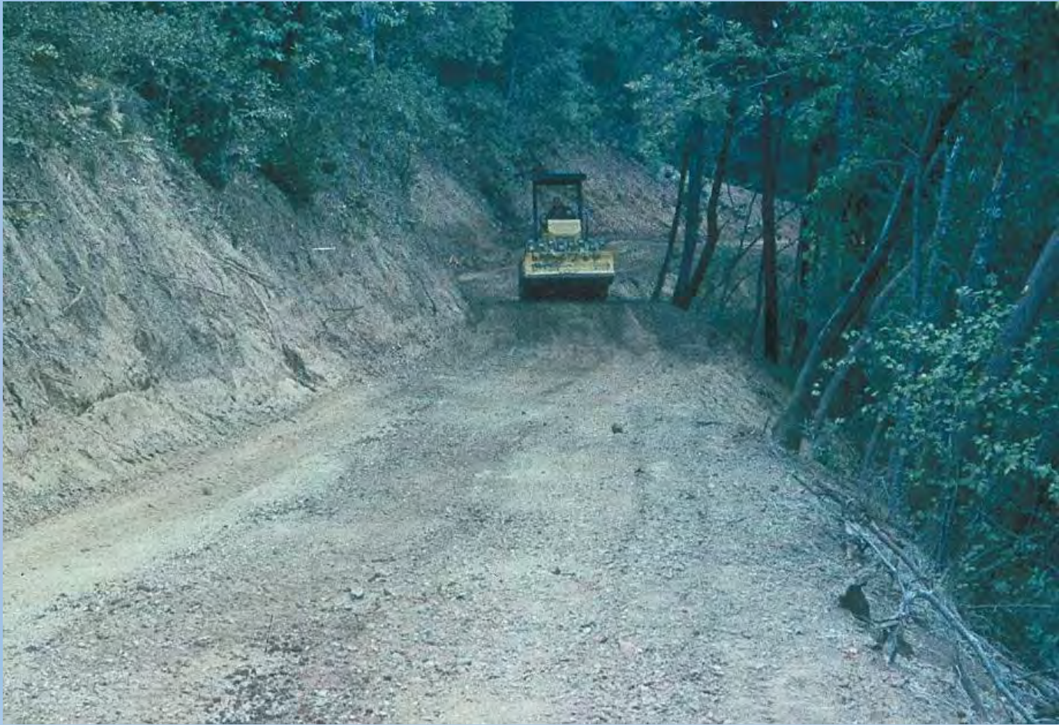
Rolling dip: rolling for compaction
