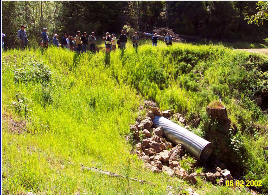
Vegetated 2:1 fillslope with extended culvert outlet and minimal armor
