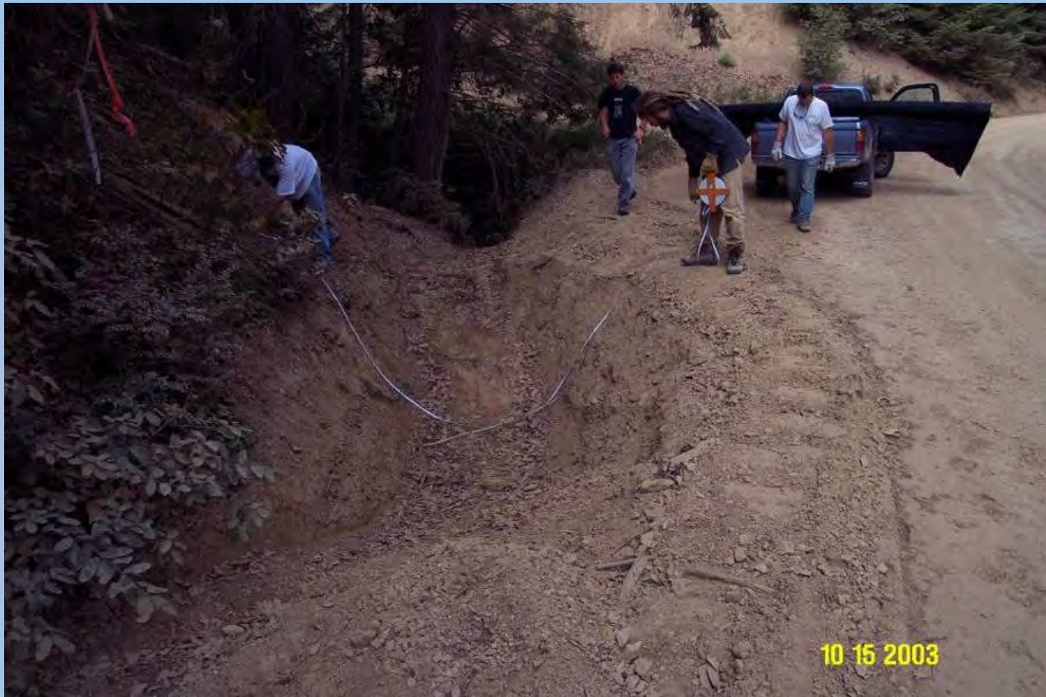
Sediment basin under construction
