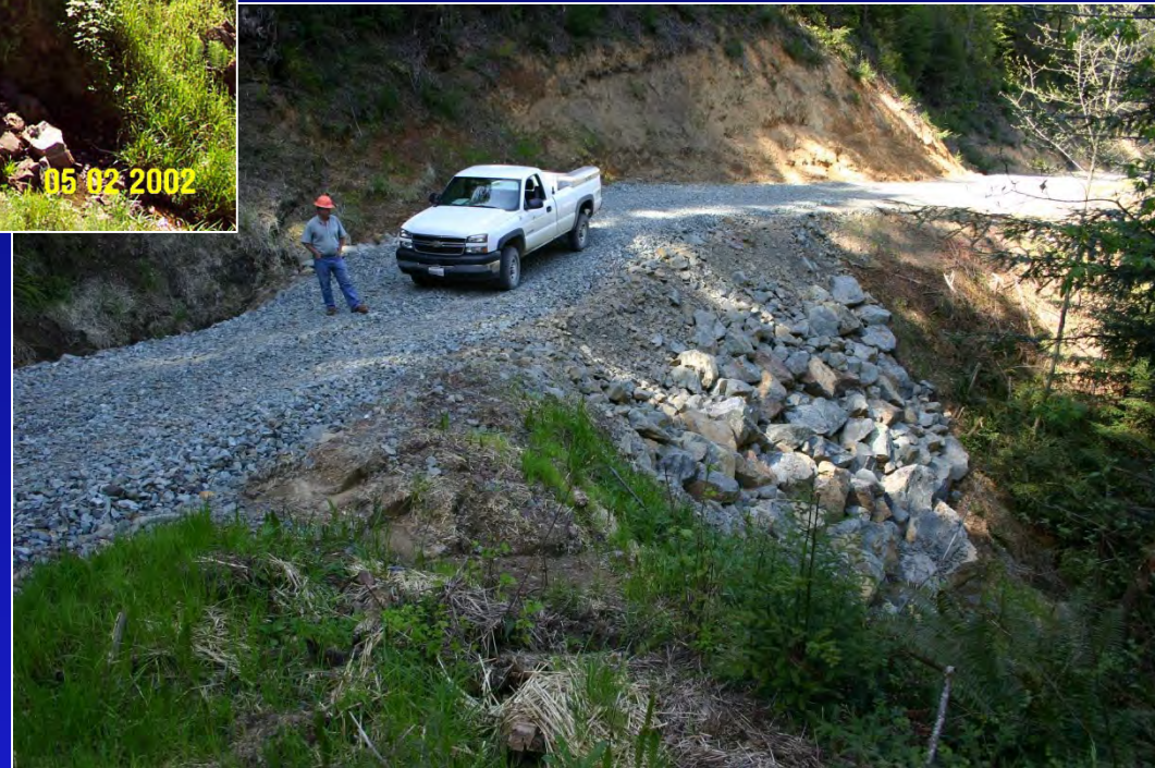
Armored 1:1 fillslope, with dense internal compaction, on steep Class III channel
