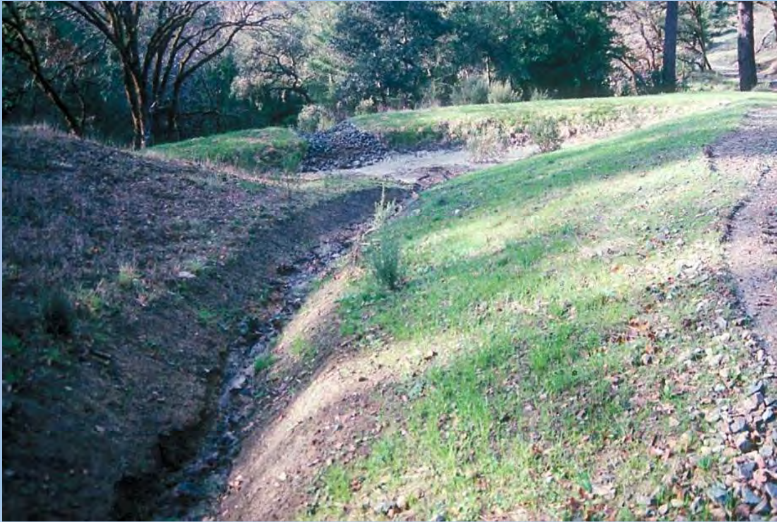
Sediment basin drainage outlet
