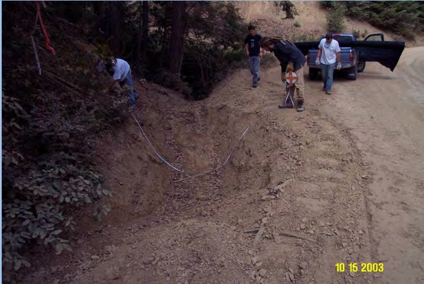
Sediment basin under construction
