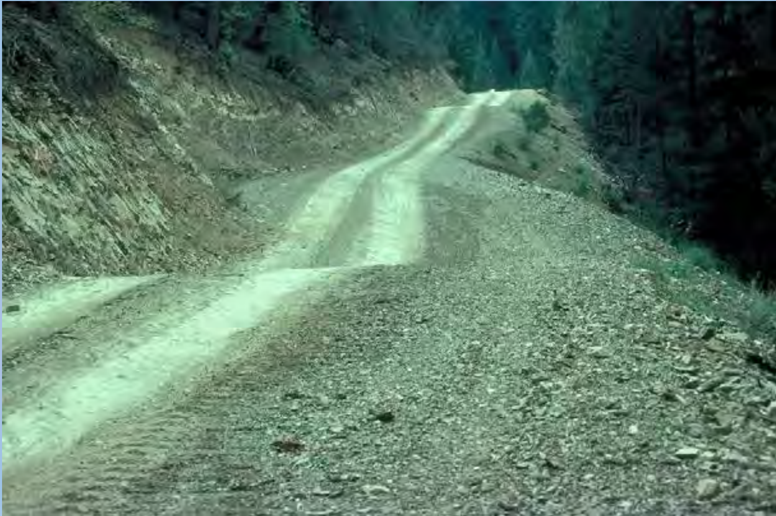
Outsloped with rolling dips
