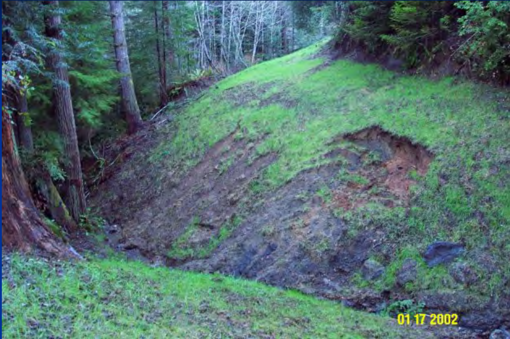
Spoil disposal on sideslopes of decommissioned stream crossing
