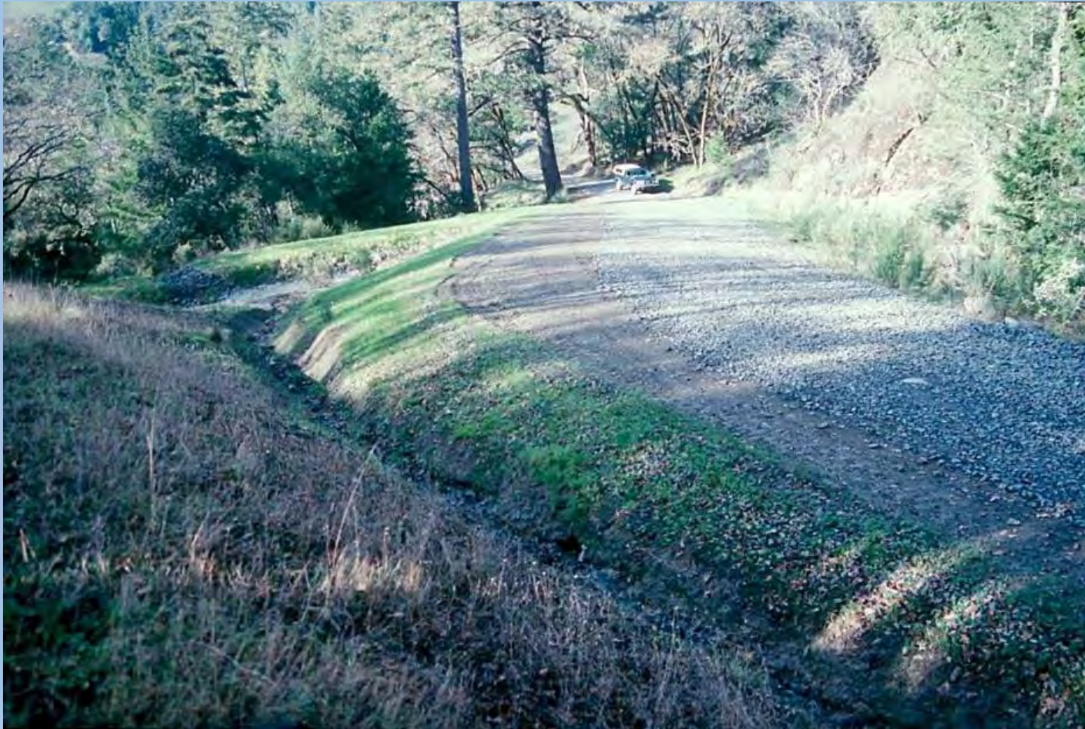
Sediment basin at end of through-cut
