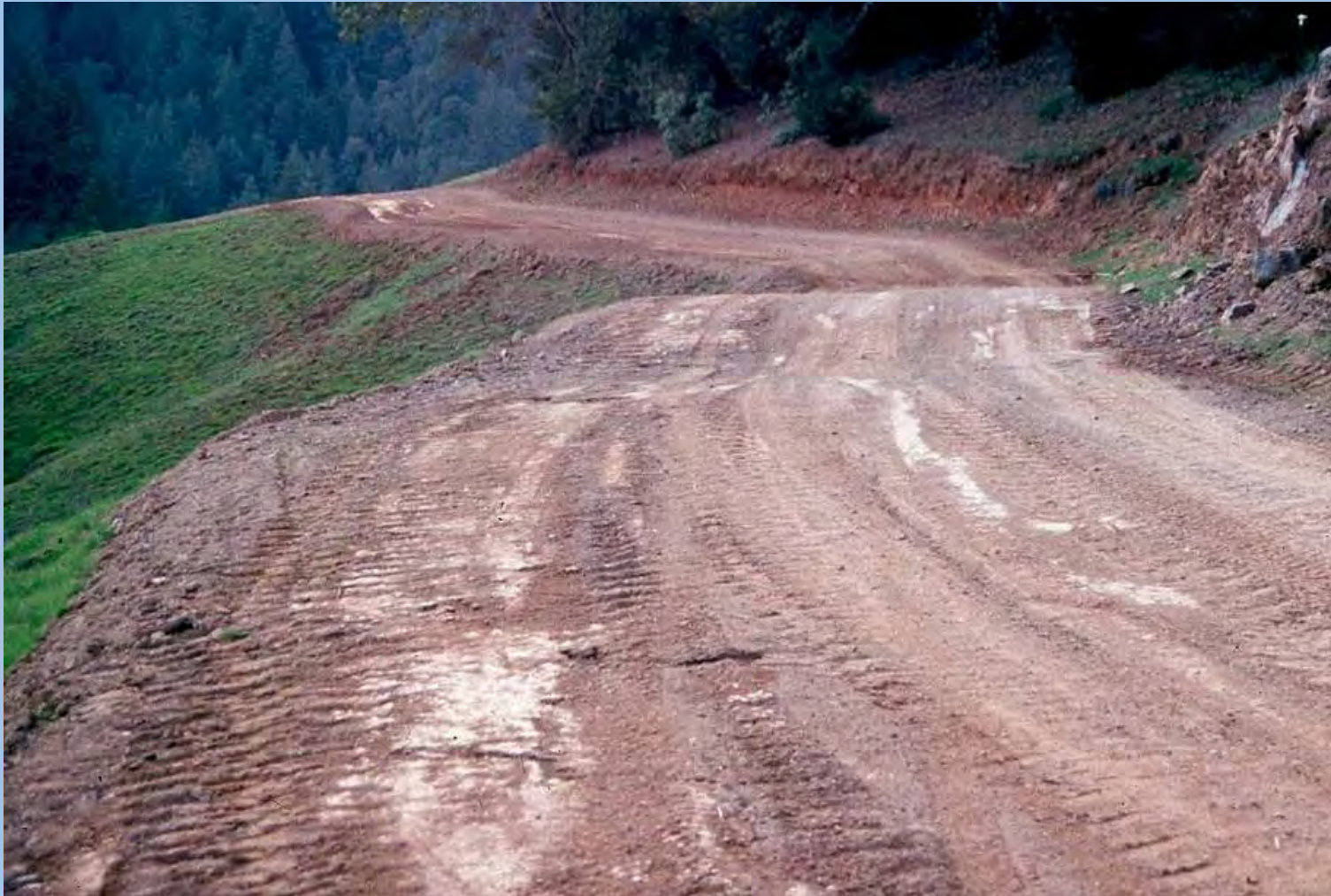
Outsloped with abrupt rolling dip
