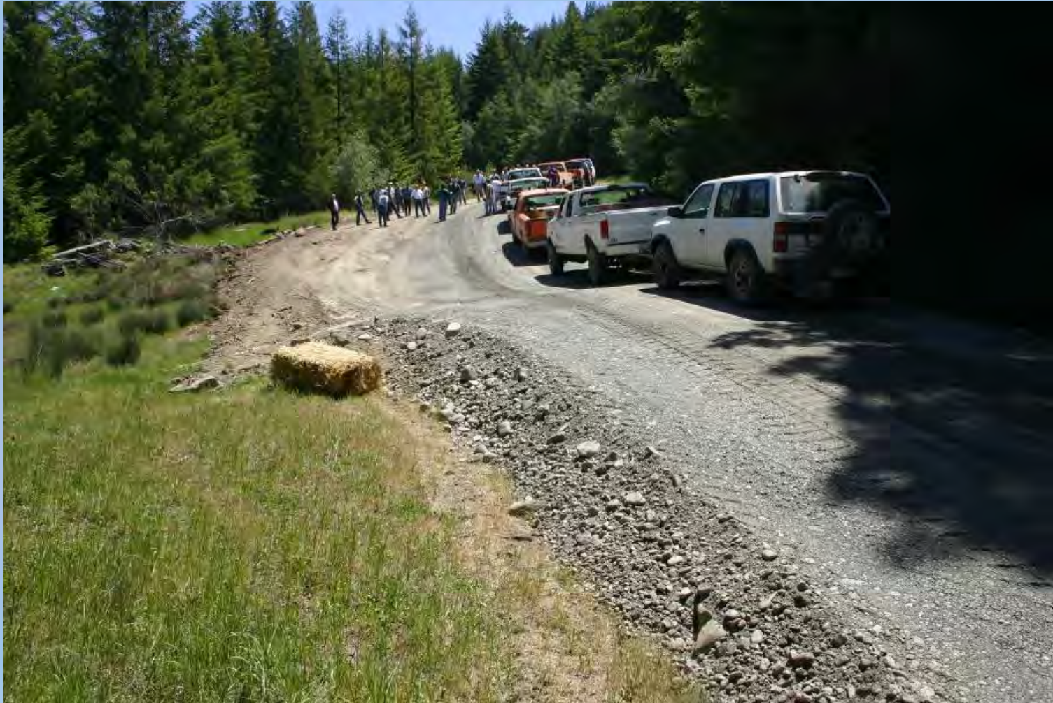
Outsloped with rolling dips
