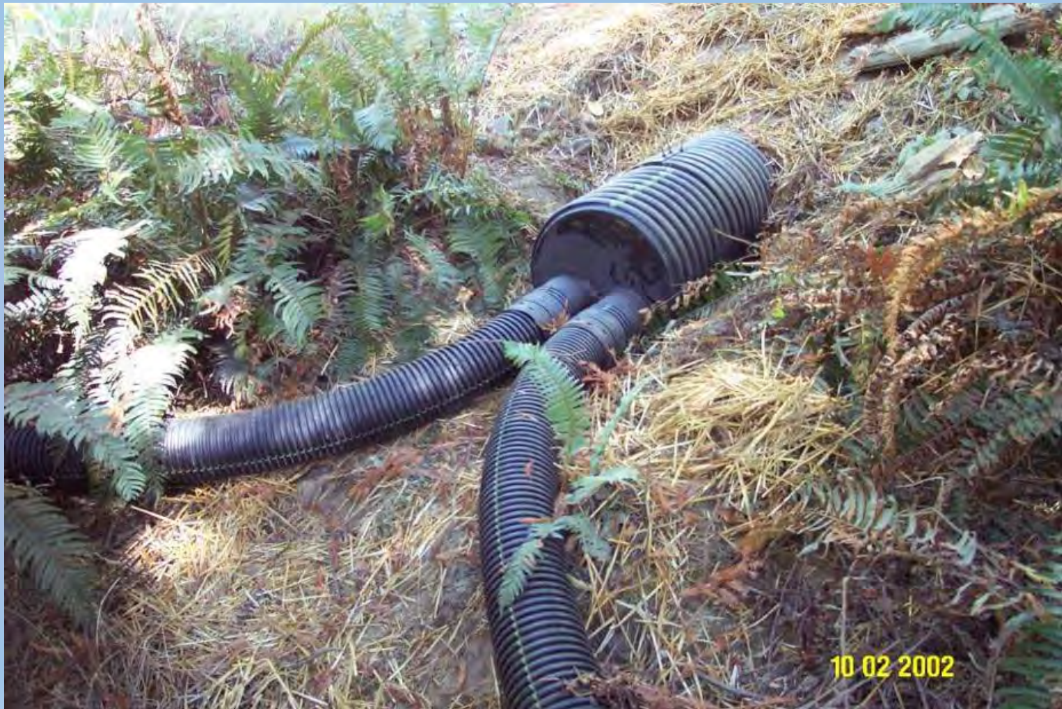
Perforated DRC flex pipe spreaders
