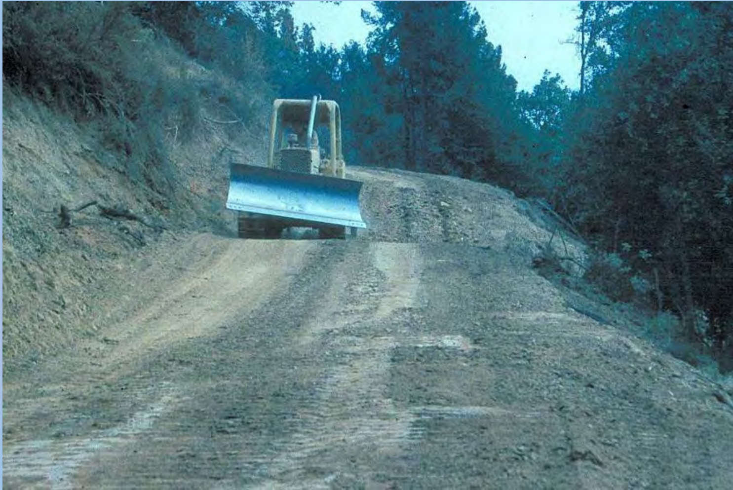
Rolling dip construction using ripping cat
