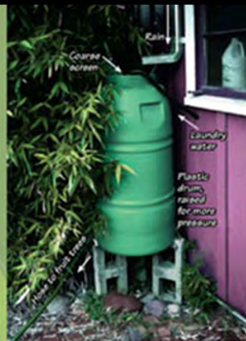
Simple Laundry Drum with Rainwater Harvesting
