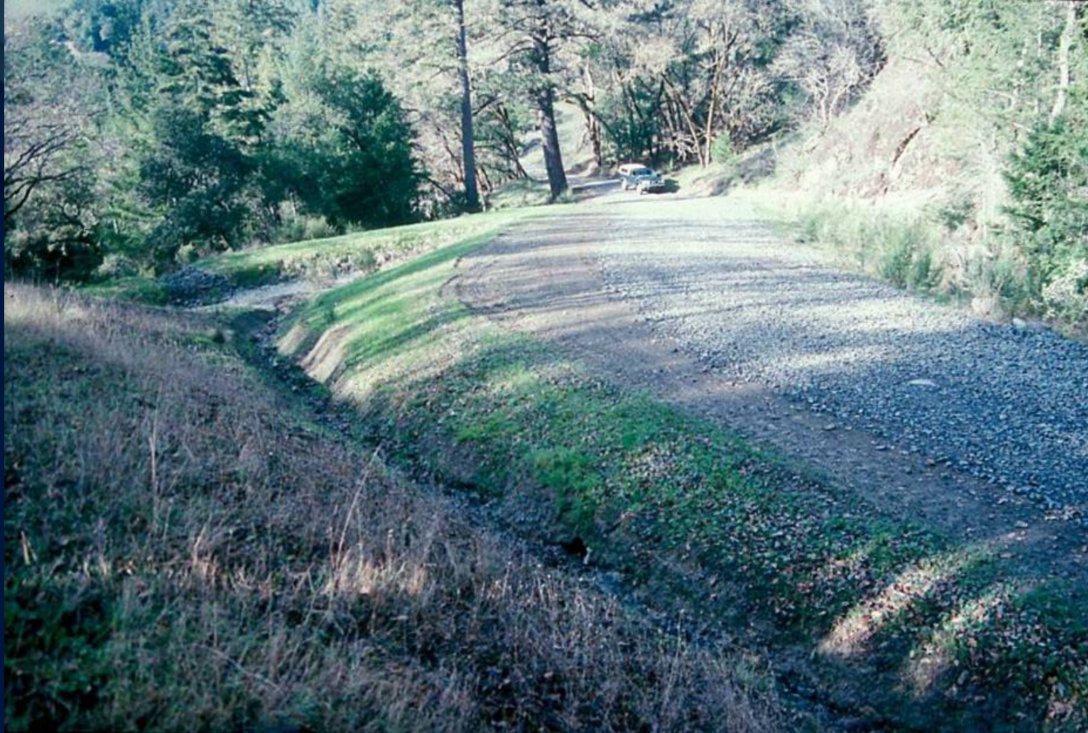
Roadside sediment retention basin
