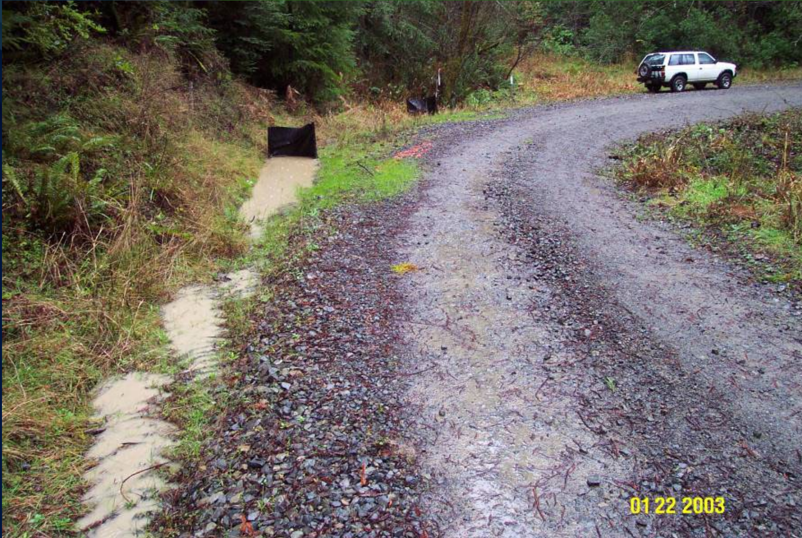
Silt fence ditch filter
