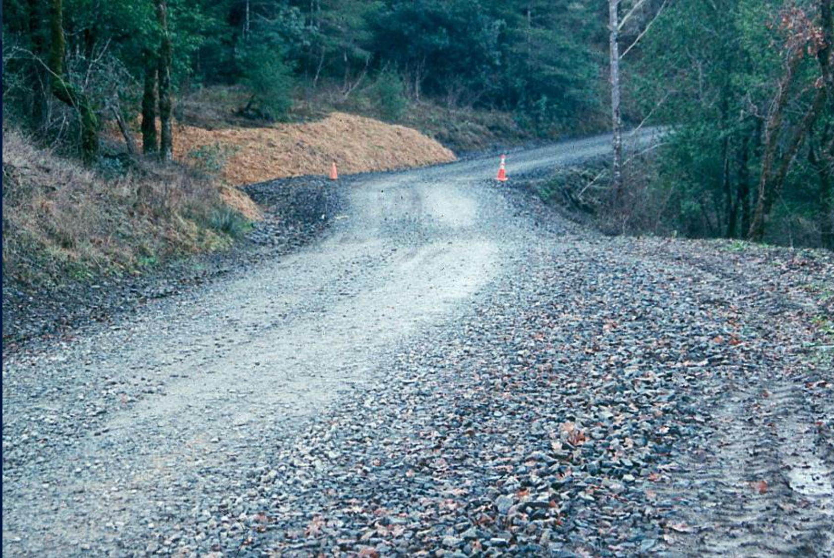
Outsloped with ditch
