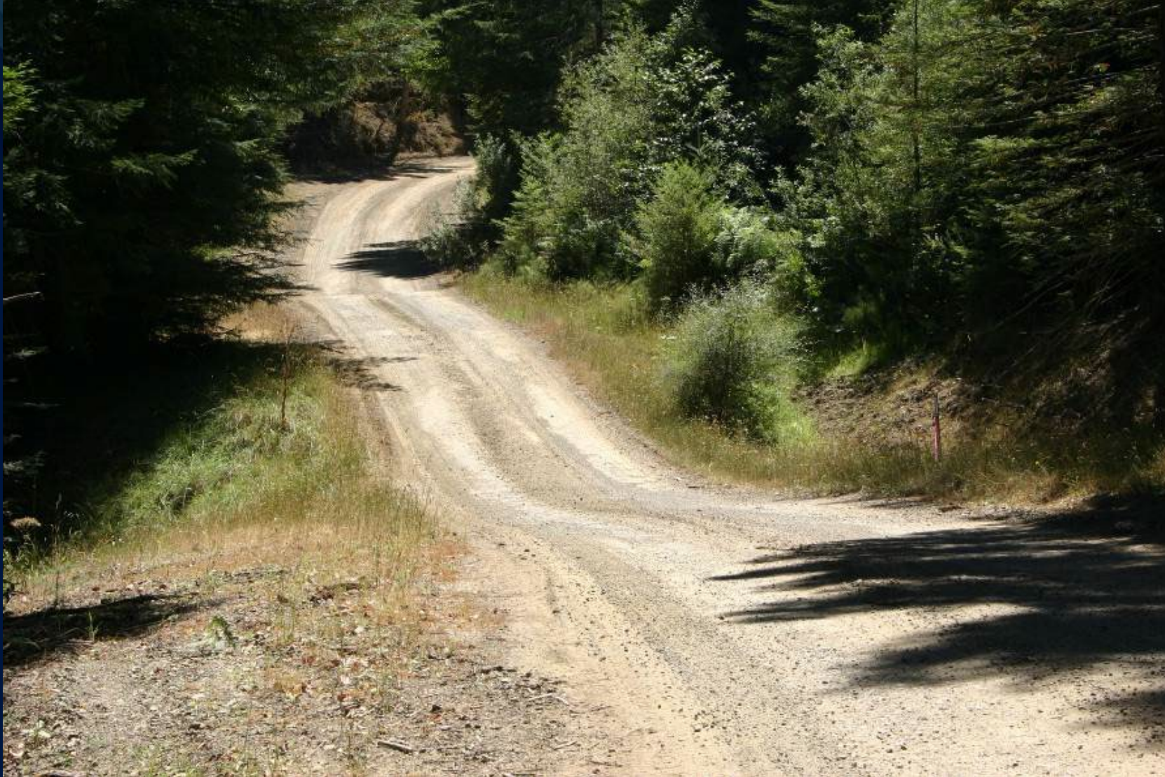
Road with rolling grade
