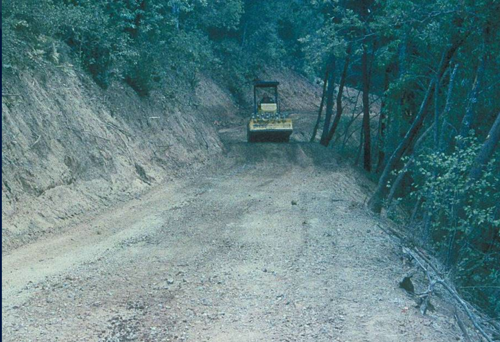
Rolling dip: rolling for compaction
