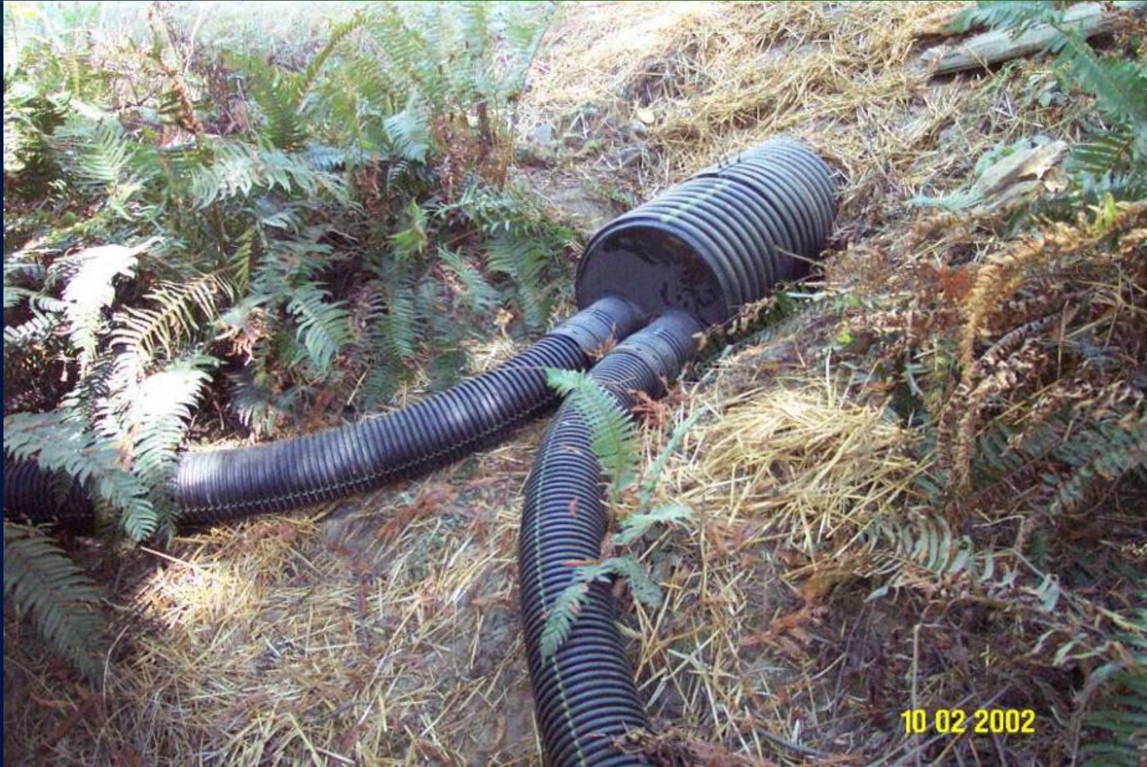
Perforated DRC flex pipe spreaders
