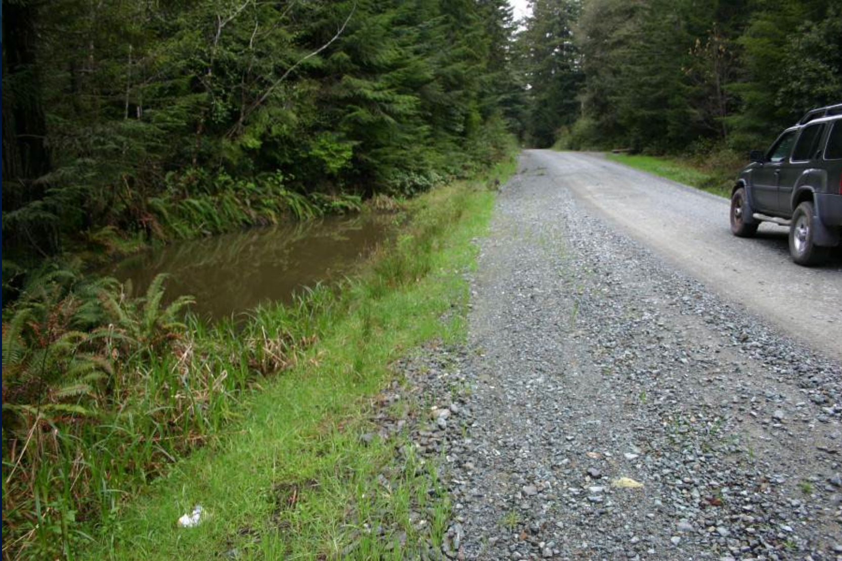
Roadside sediment retention basin
