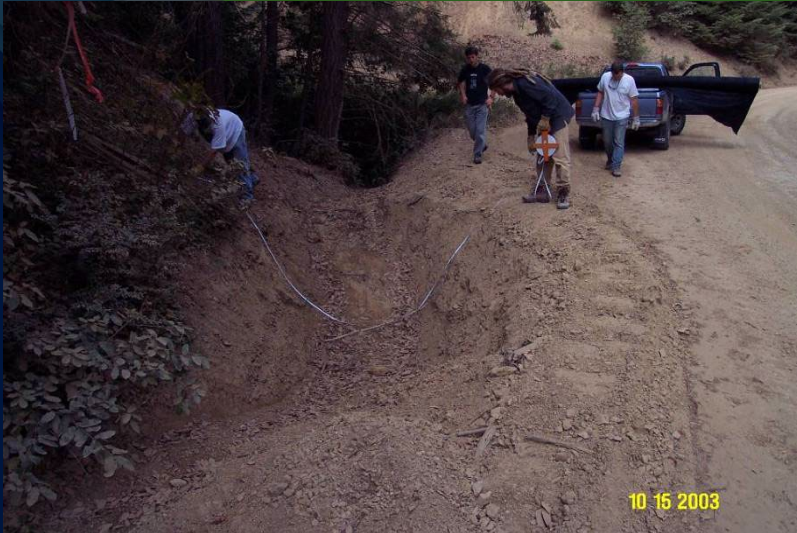
Sediment basin under construction
