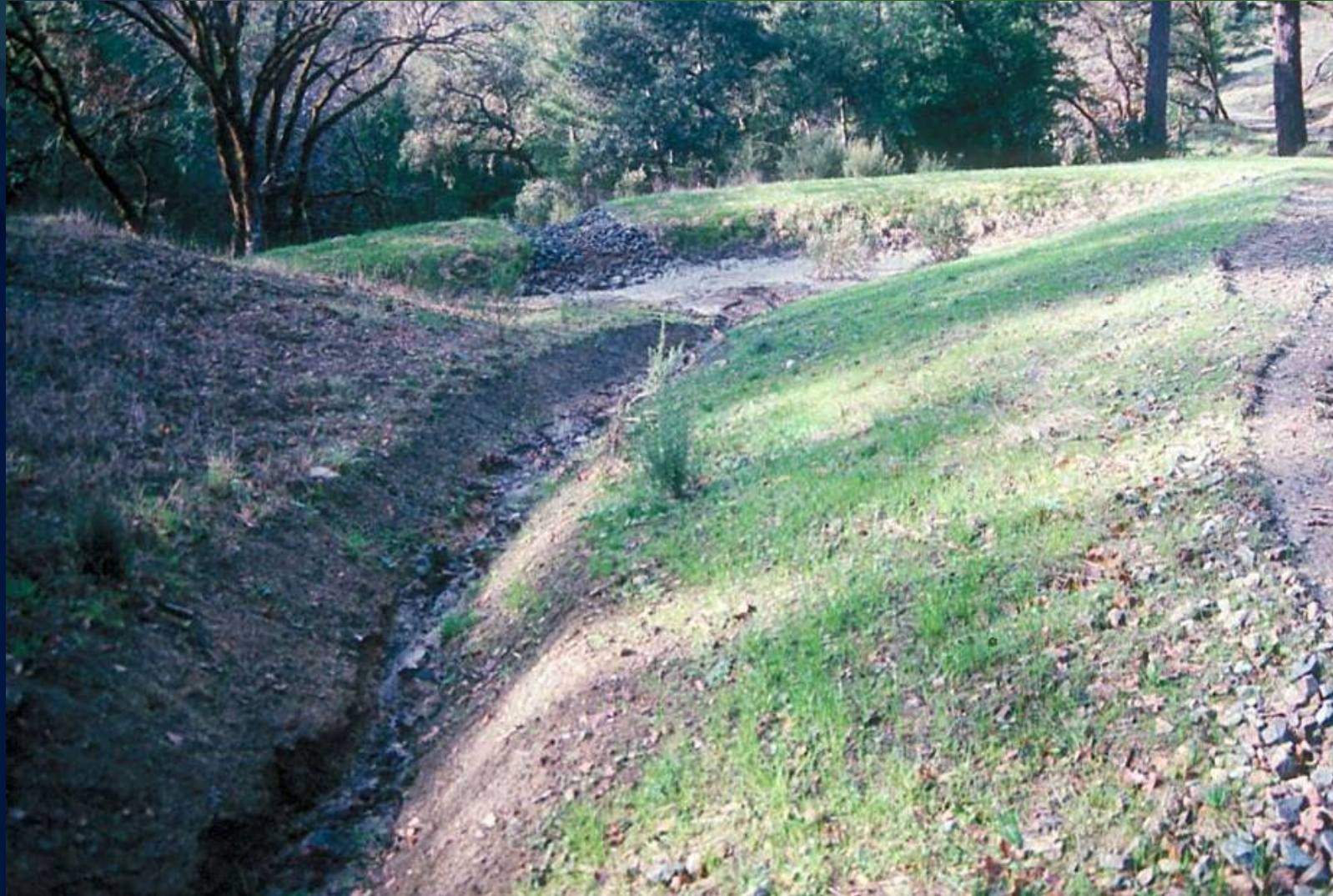
Sediment basin drainage outlet
