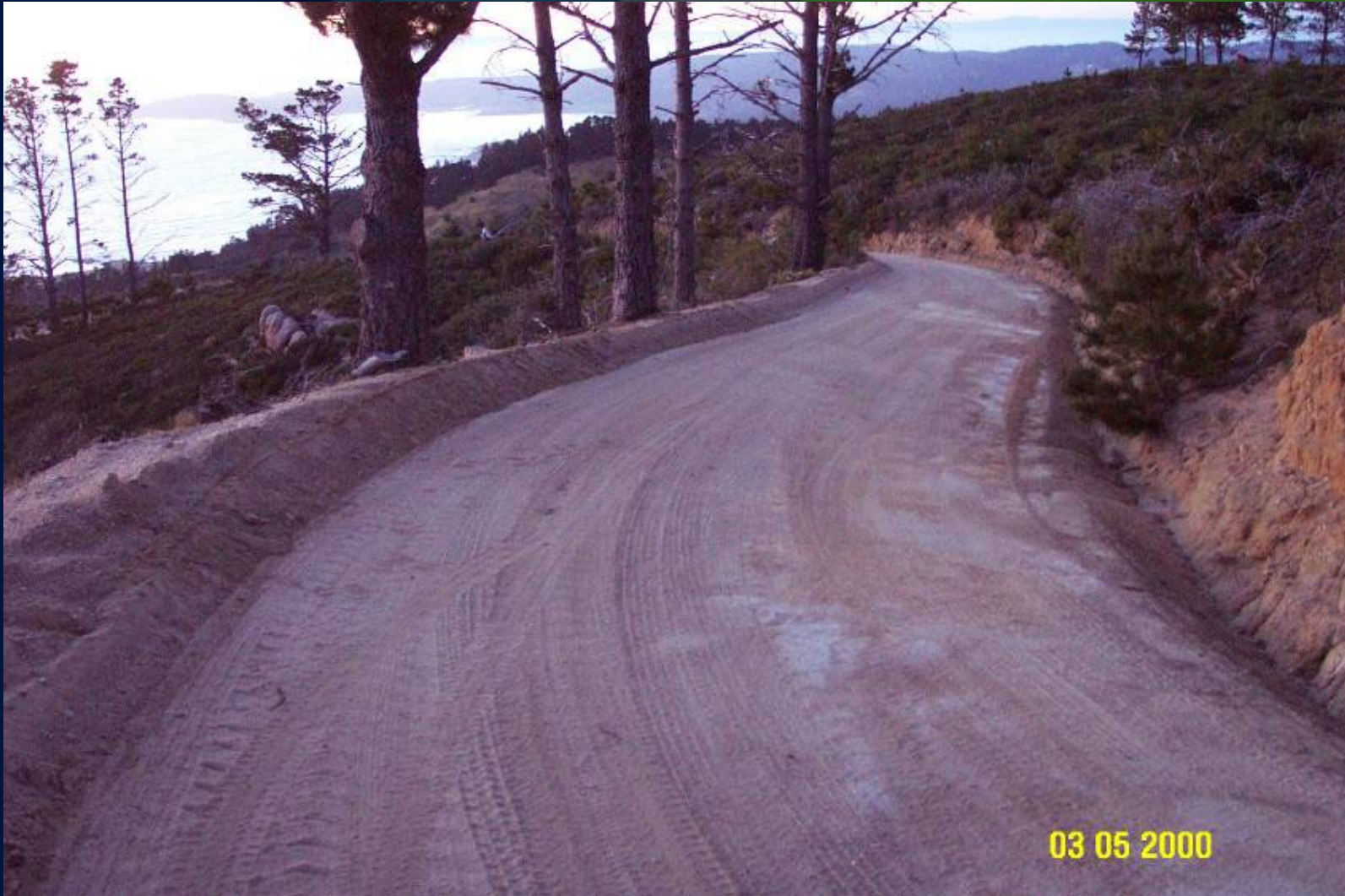
INSLOPED ROAD WITH DITCH AND BERM
