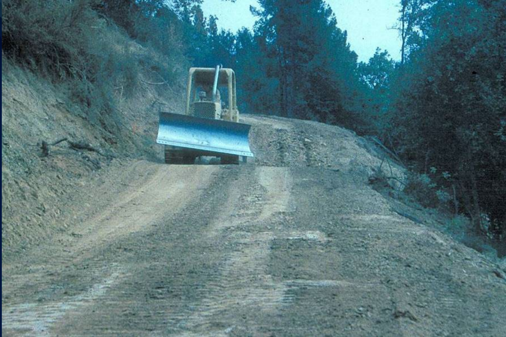
Rolling dip construction using ripping cat
