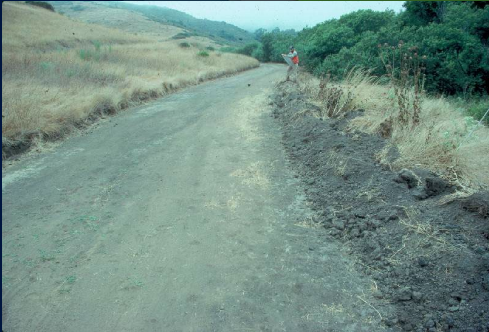
FLAT ROAD WITH SIDECAST BERM
