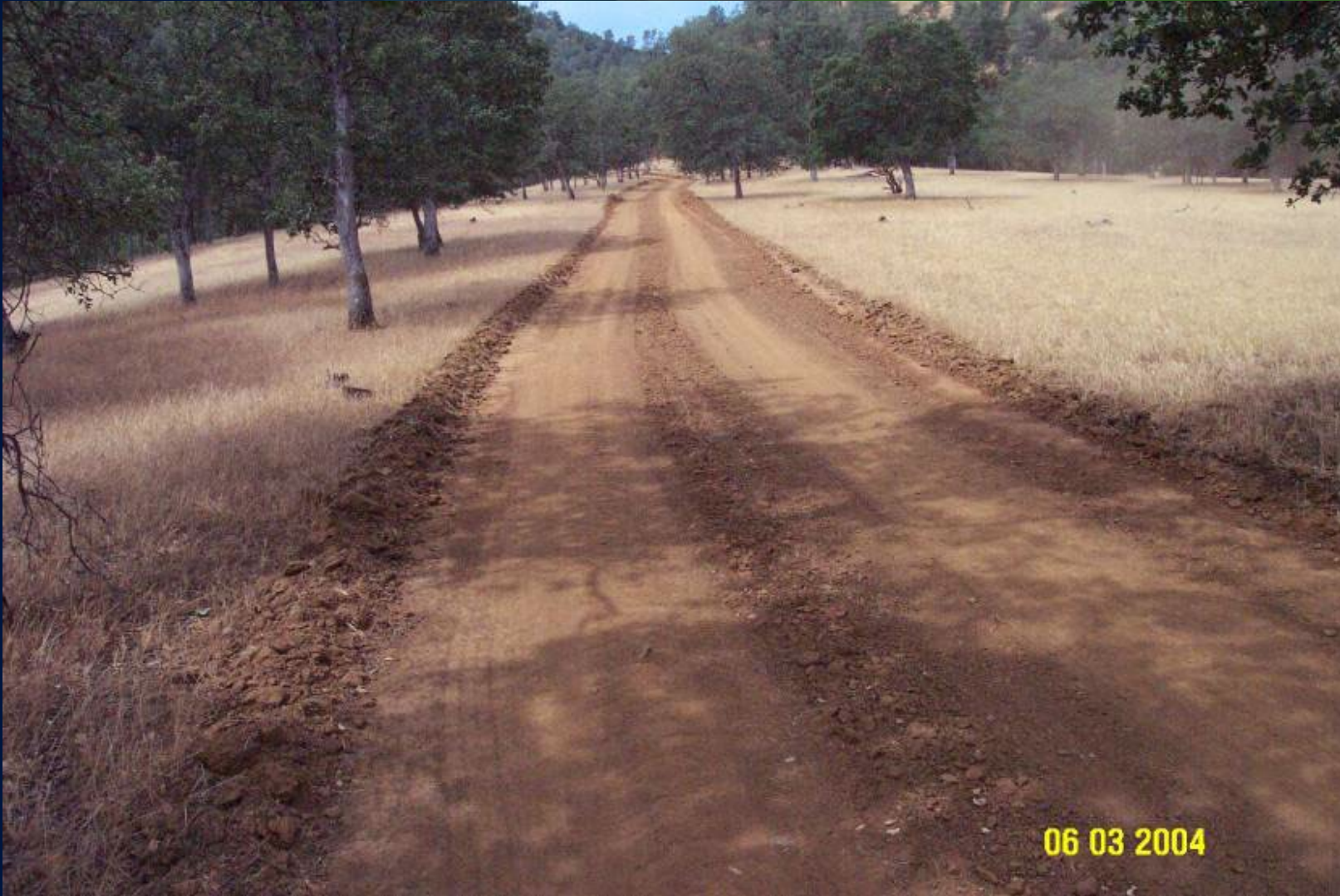
OUTSLOPED ROAD WITH SMALL BERM
