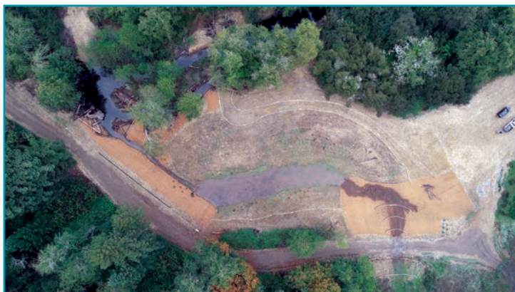
Newly constructed flooded wetland feature on South Fork Ten Mile River. Photo Credit: The Nature Conservancy.
