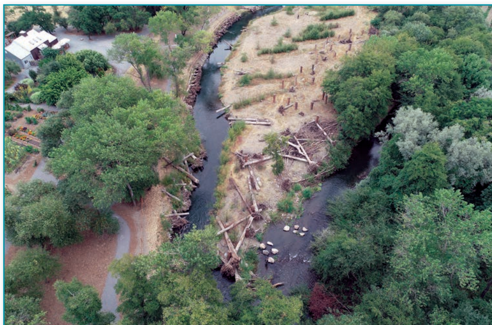
Side channel constructed in 2016 on Dry Creek at the Truett-Hurst tasting room which is where the Dry Creek tour will culminate.
